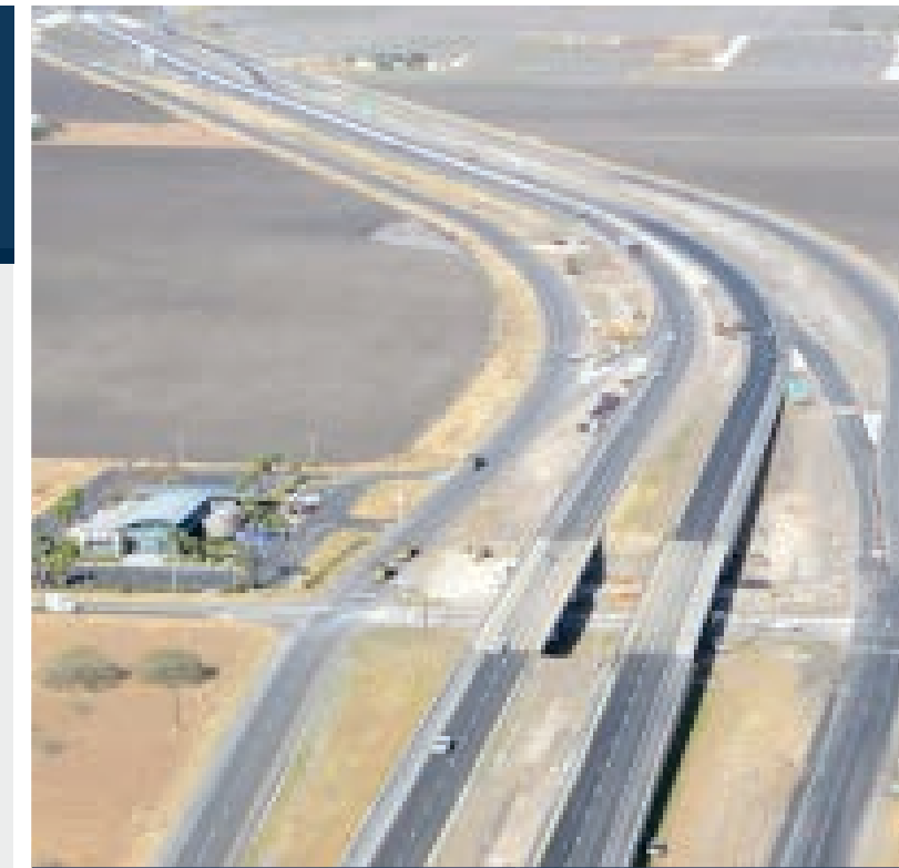
US 77 Overpass in Bishop, TX
