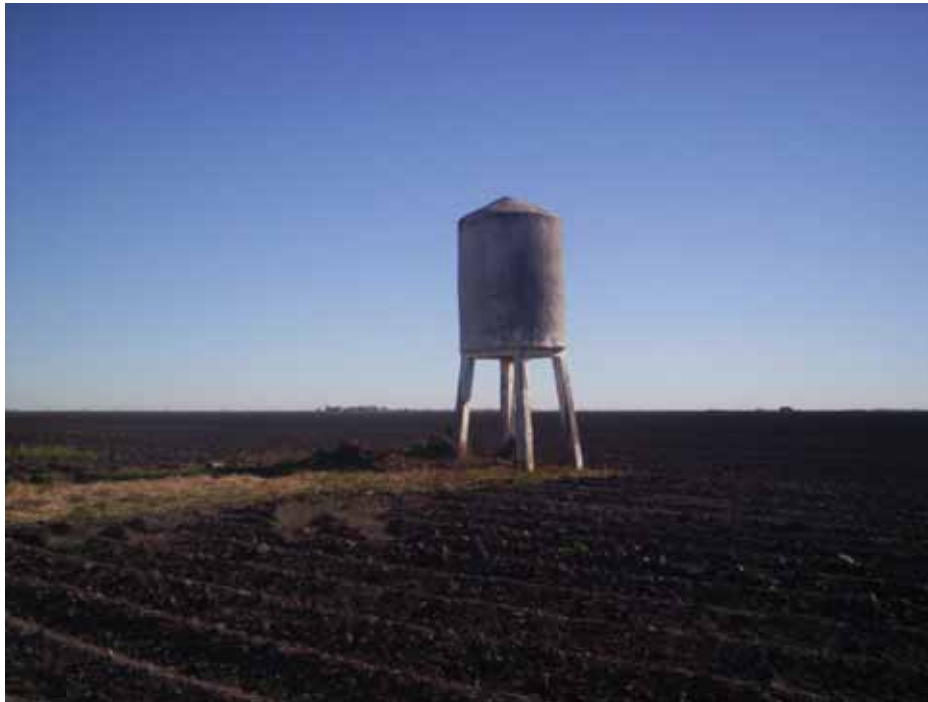
Photo 20 Water storage tank (Map ID 12 – Figure A.4.13-4) within proposed ROW (December 2008).
