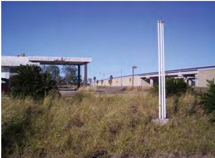
Photo 26 Abandoned B&E gas station (Map ID 21 – Figure A.4.13-10) adjacent to ROW. UST stick-up vents on right side of photograph (December 2008).
