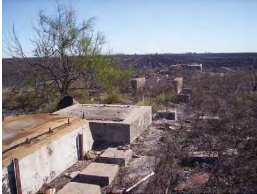
Photo 19 Potential petroleum well site (Map ID 10 – Figure A.4.13-2) within proposed ROW (December 2008).
