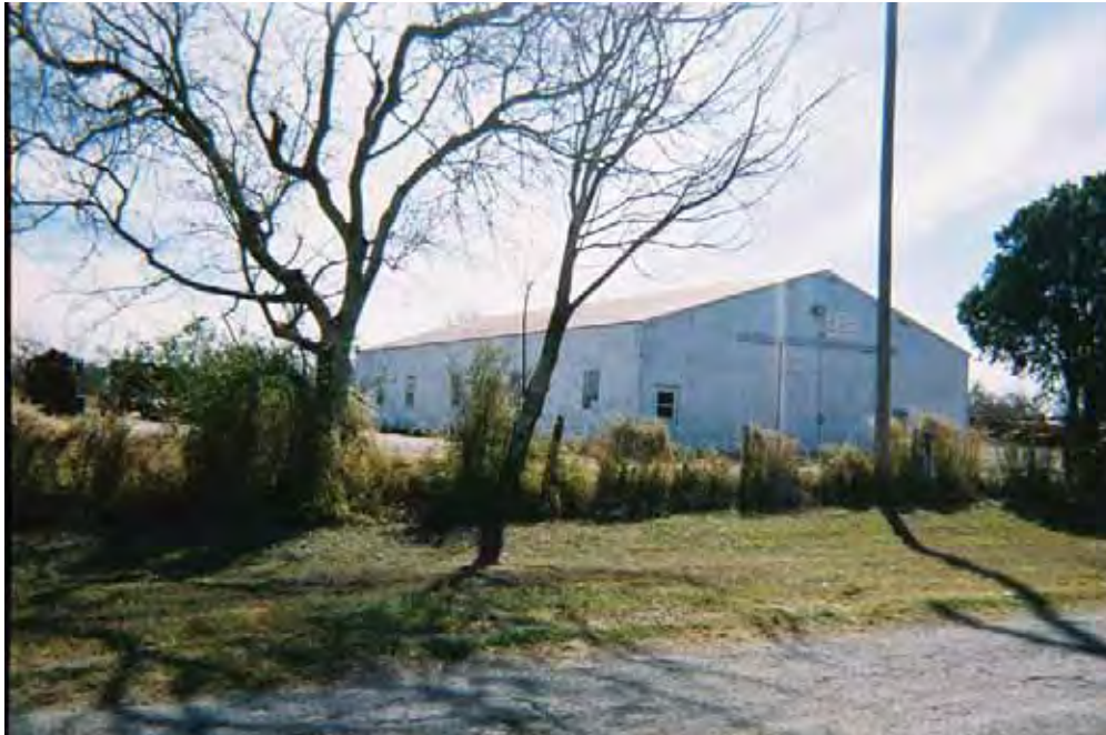
Photo 25 Kleberg County Maintenance Yard (Map ID 20 – Figure A.4.13-9) adjacent to proposed ROW (February 2009).
