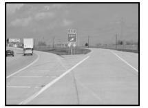
The part of an interchange that allows a motorist to exit a controlled access roadway.
