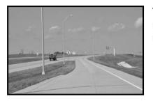
The part of an interchange that allows a motorist to enter a controlled access roadway.
