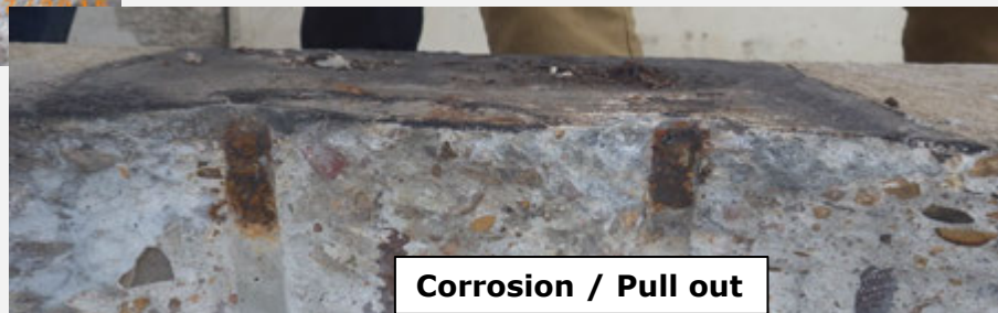
Damaged Anchor Bolt
