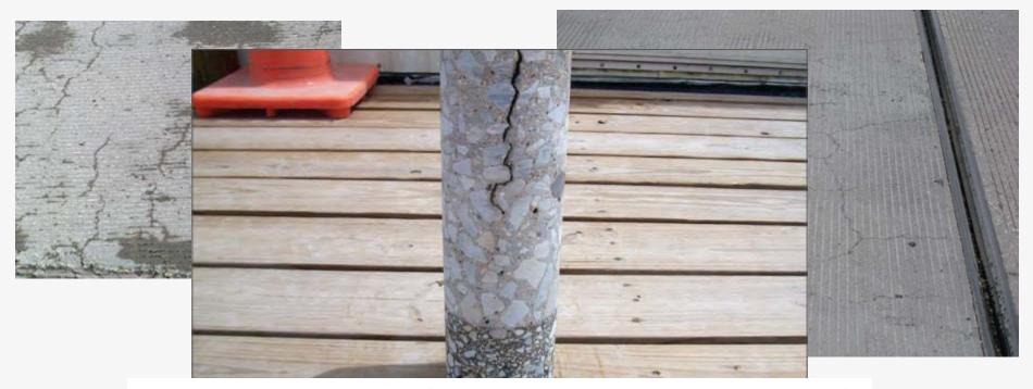
The Engineer will inspect the deck or slab for plastic shrinkage and settlement cracking after completion of final curing and within 5 days after curing mats are removed. Seal any noted shrinkage cracks attributable to Contractor placing, curing, and finishing practices as well as transverse cracks over interior bents in continuous units using gravity feed crack repair as directed in accordance with Item 780, "Concrete Crack Repair," at no cost to the Department.
