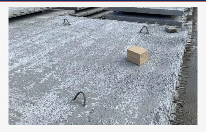
Any flaking, scaling, or laitance must be removed prior to placing concrete.
