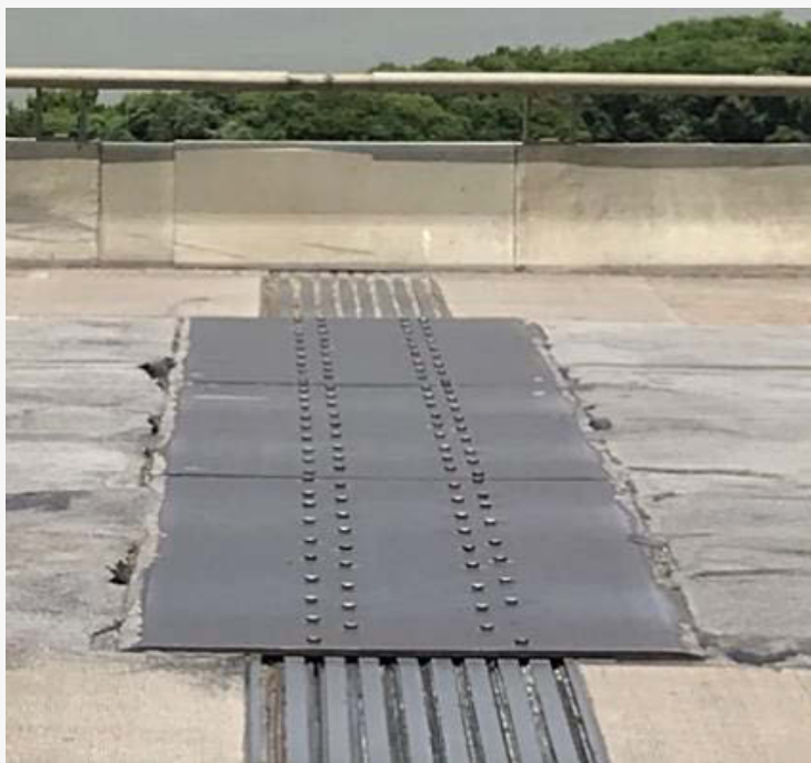
Modular Joint Deterioration
