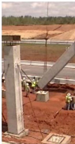
(a) Full-height precast column
