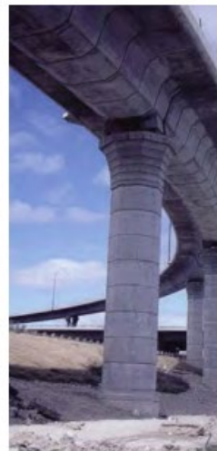
(b) Precast segmental column
