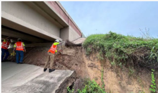
Rotational Failure
