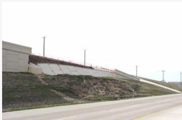
Excessive load at top of slope
