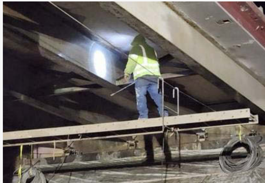
Worker Supported on Cables
