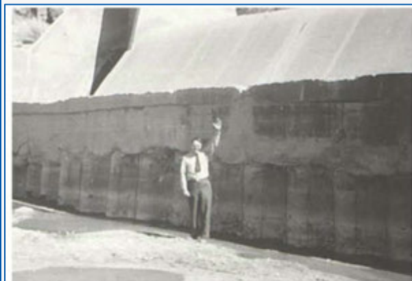
i. Channel degradation resulting from lack of upstream sediment source, downstream from Sumner Dam near Fort Sumner, NM.
