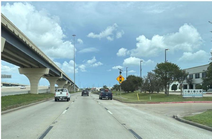
Photograph 1. South Sam Houston Parkway East at Syzygy Plasmotics Driveway (shared driveway with proposed development – to right) Photograph Date: 9/2/2024
