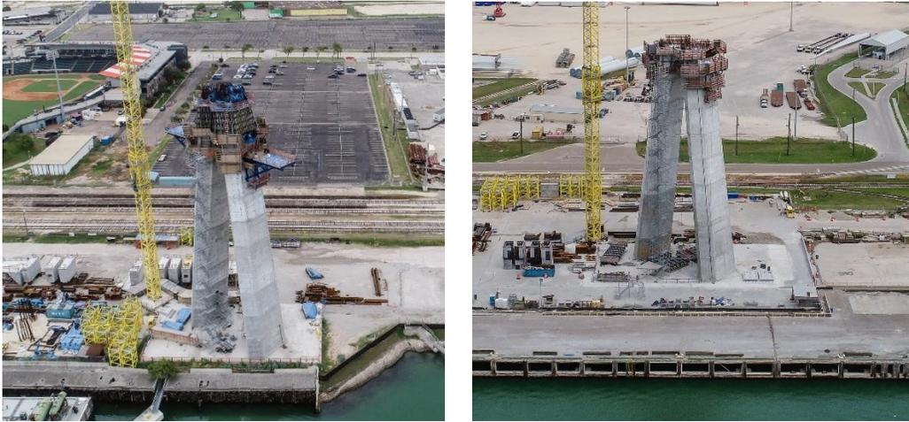
Figure 3: Proximity of footing to bulkheads (left: south tower, right: north tower).
