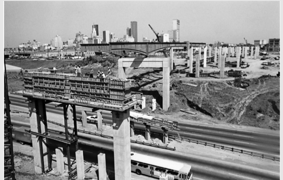
Interstate 345 under construction in 1969 Source: The Dallas Library
