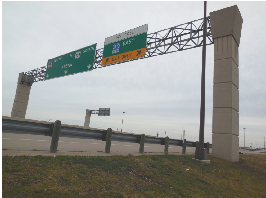
Figure 7.2 – Example of concrete sign columns supporting horizontal trusses
