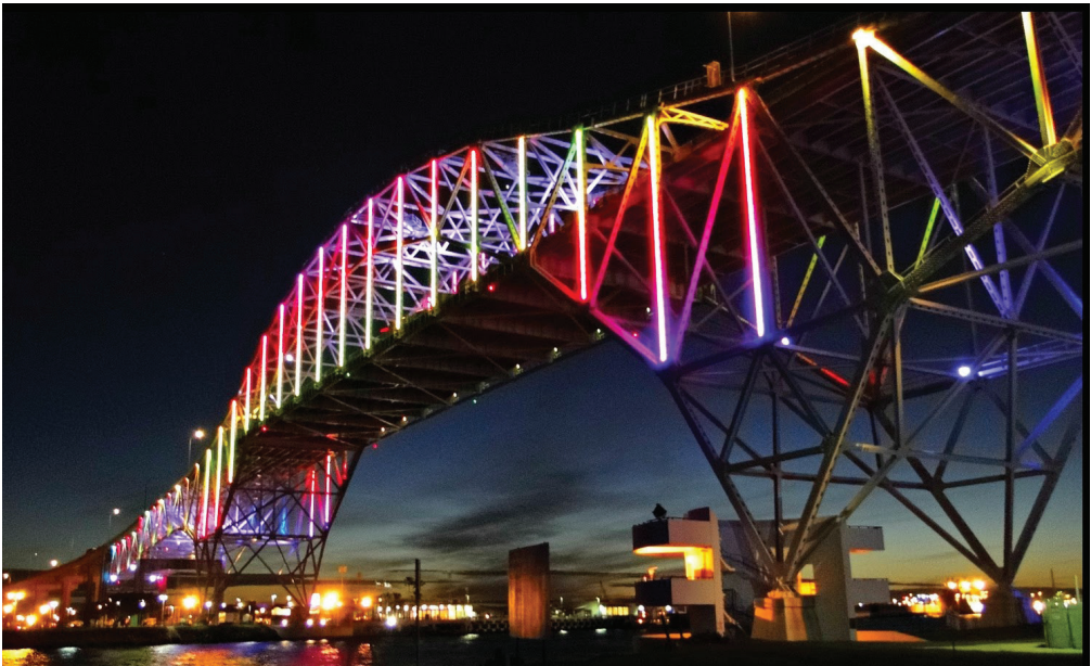
Figure 8.1 – Existing Harbor Bridge multi-color display
