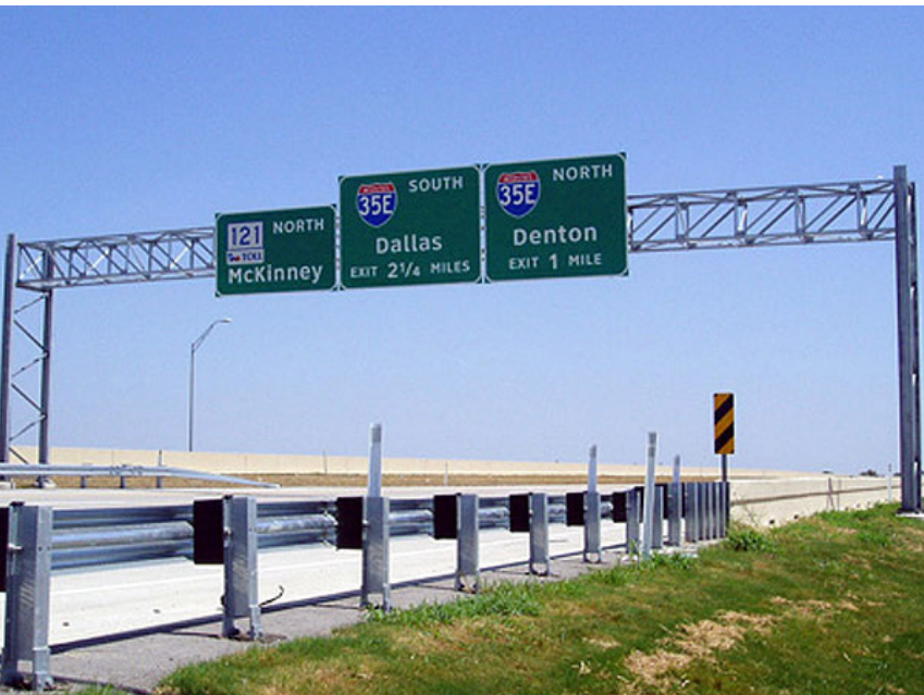
Figure 7.1 – Overhead roadway signage, visibility of open vertical trusses shall not be accepted
