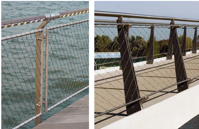
Figure 6.4 – Examples of acceptable fence fabric
