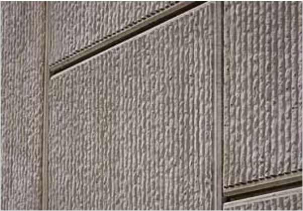
Figure 5.1 – Fractured fin texture on retaining walls shall not be accepted
