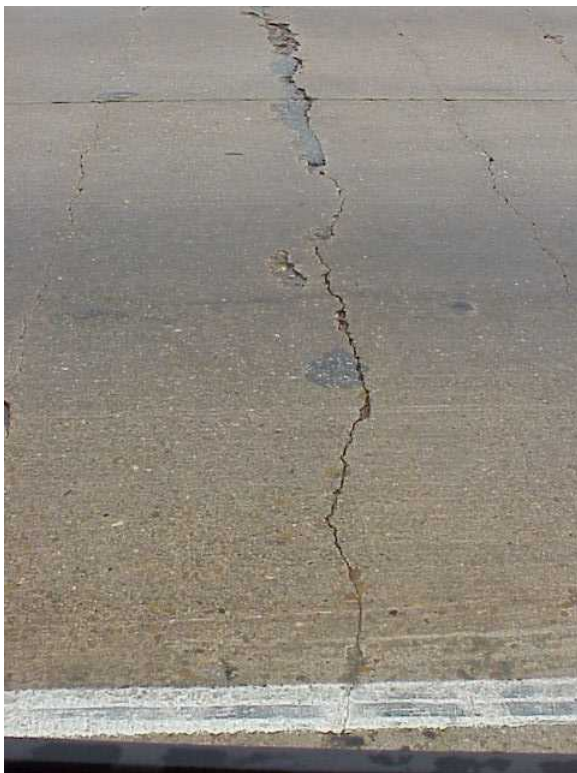
Figure 32 – Spalled Cracks
