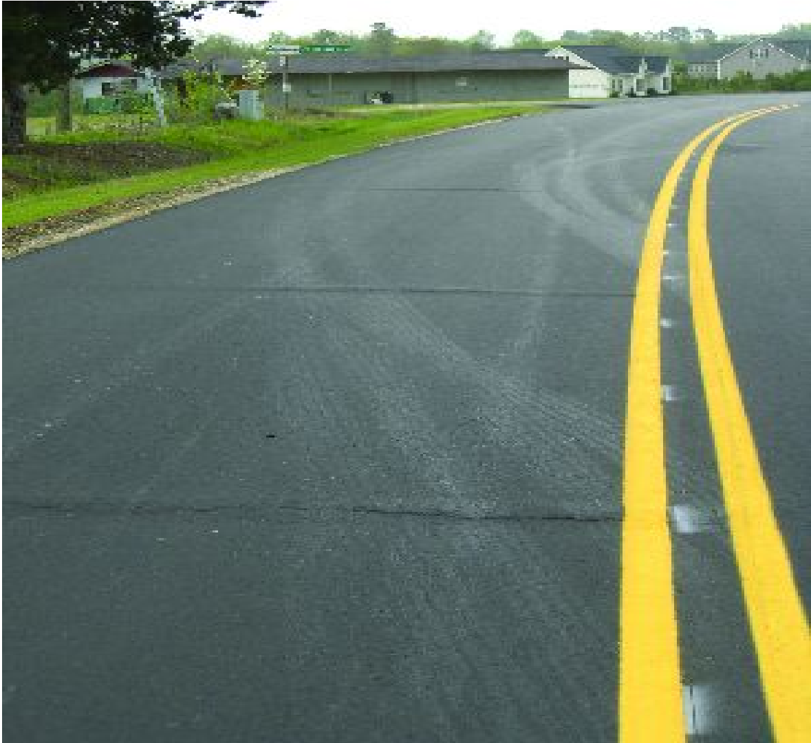
Figure 27 – Transverse Cracking
