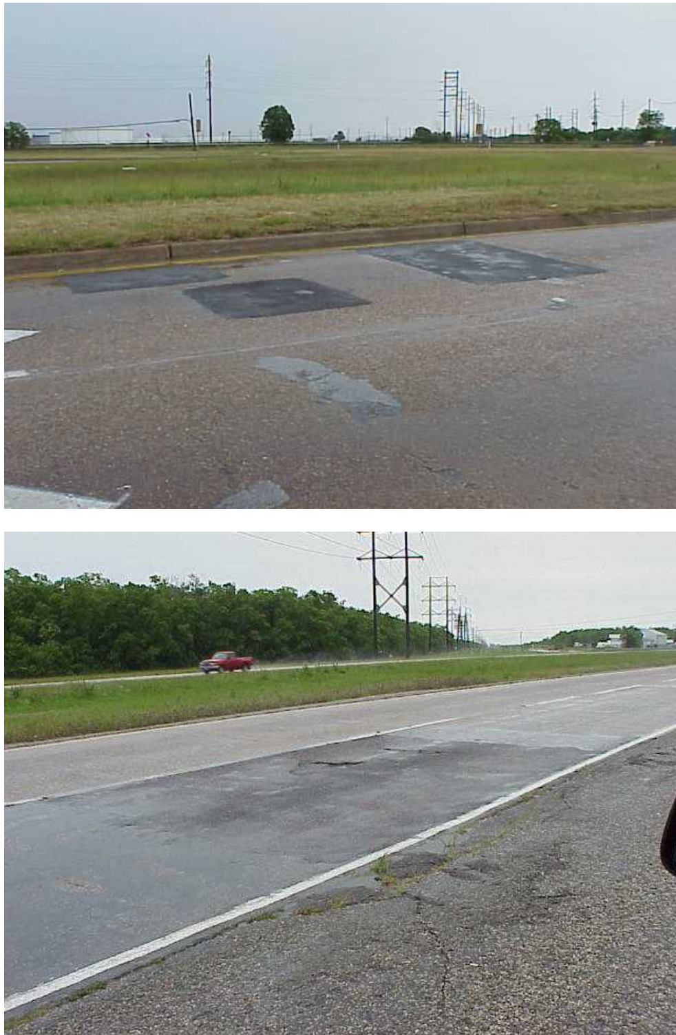
Figure 34 – Asphalt Patches
