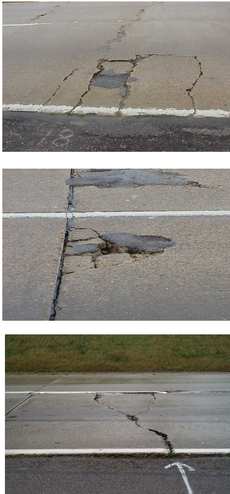
Figure 45 – Failures (punchouts)
