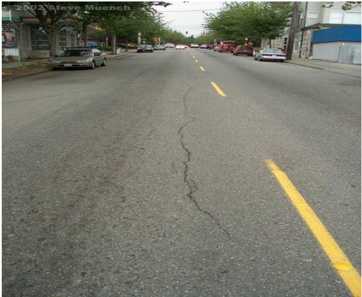
Figure 25 – Longitudinal Cracking
