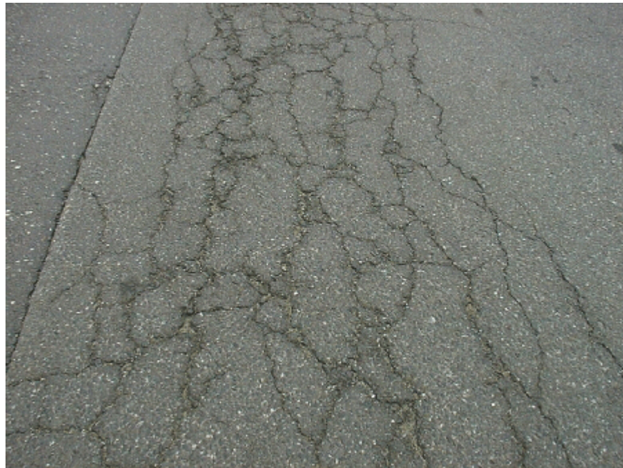
Figure 24 – Alligator Cracking
