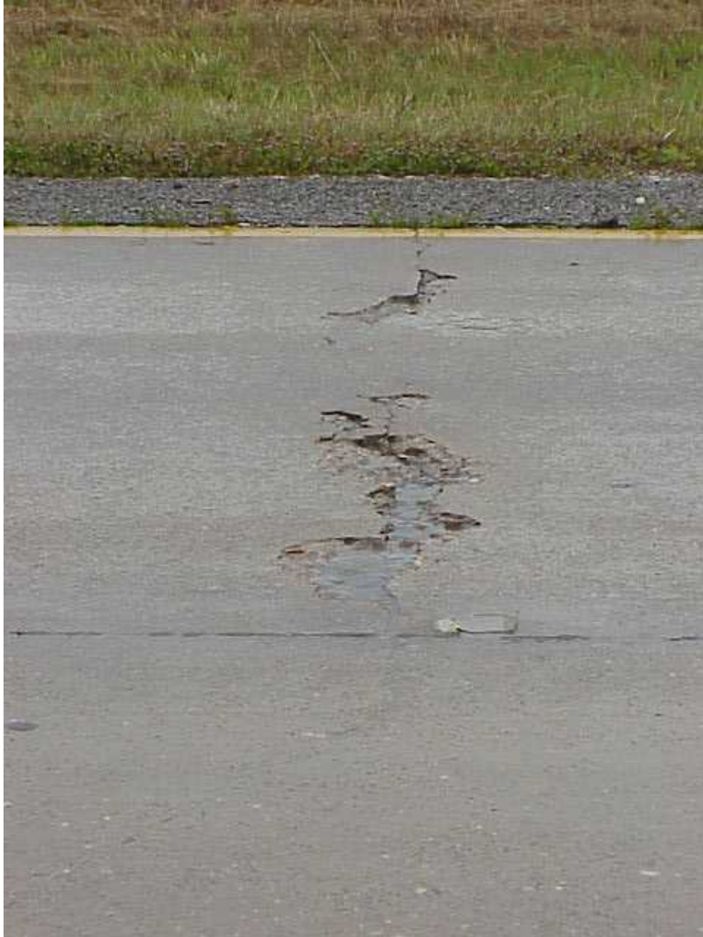
Figure 40 – Failed Crack and Failure
