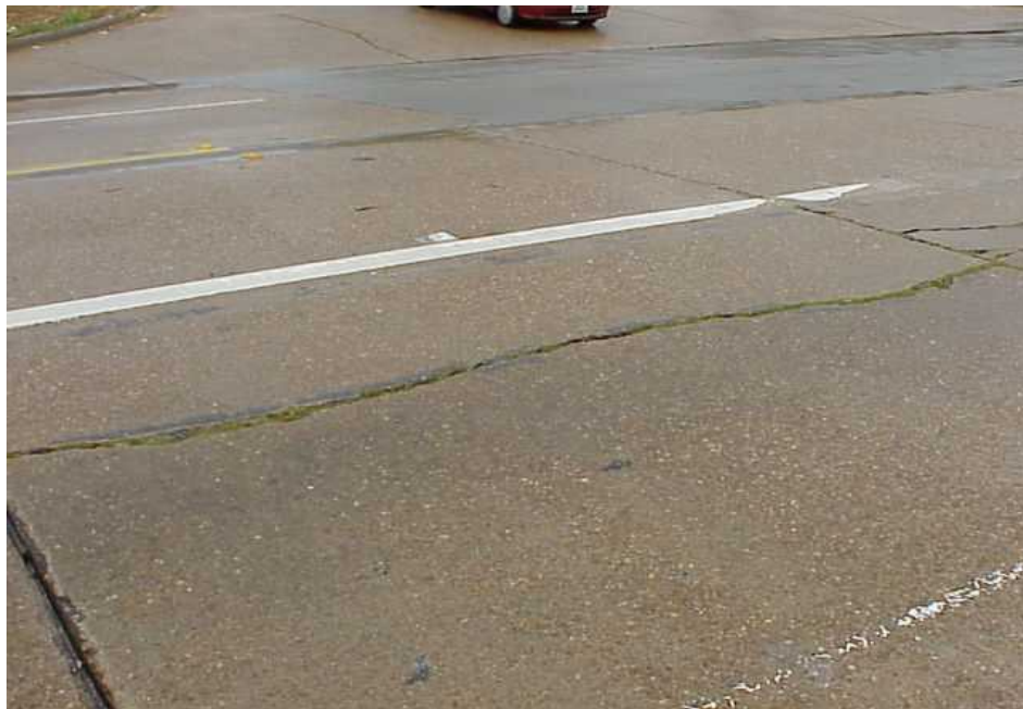
Figure 51 – Slab with Longitudinal Crack
