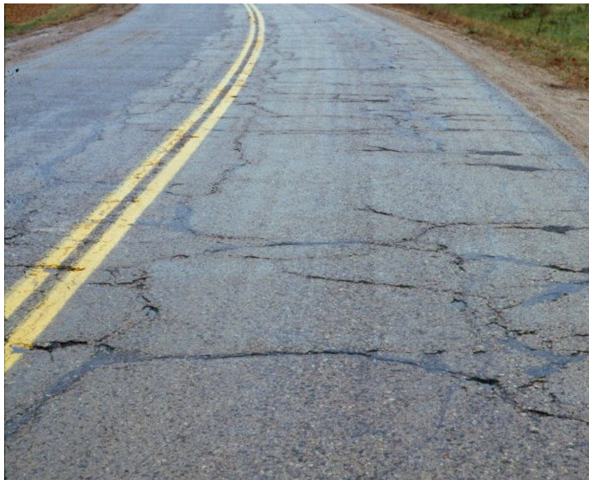
Figure 23 – More Block Cracking
