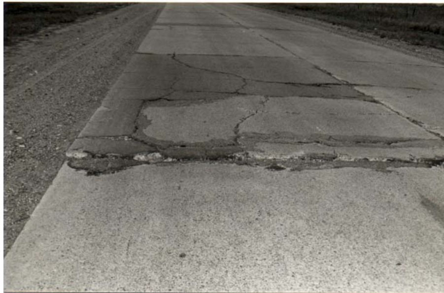
Figure 50 – Shattered Slabs
