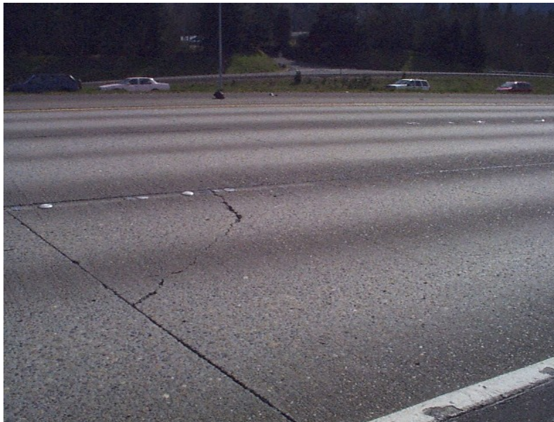
Figure 44 – Failures (corner breaks)
