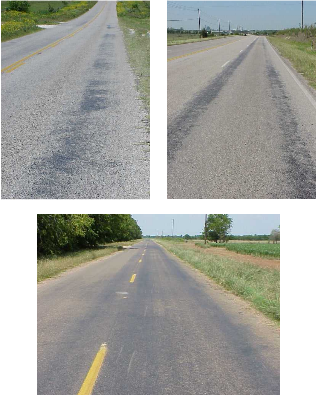
Figure 30 – Flushing
