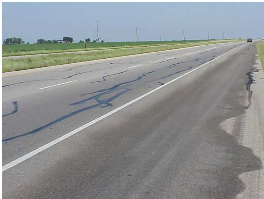
Figure 26 – Longitudinal Cracking
