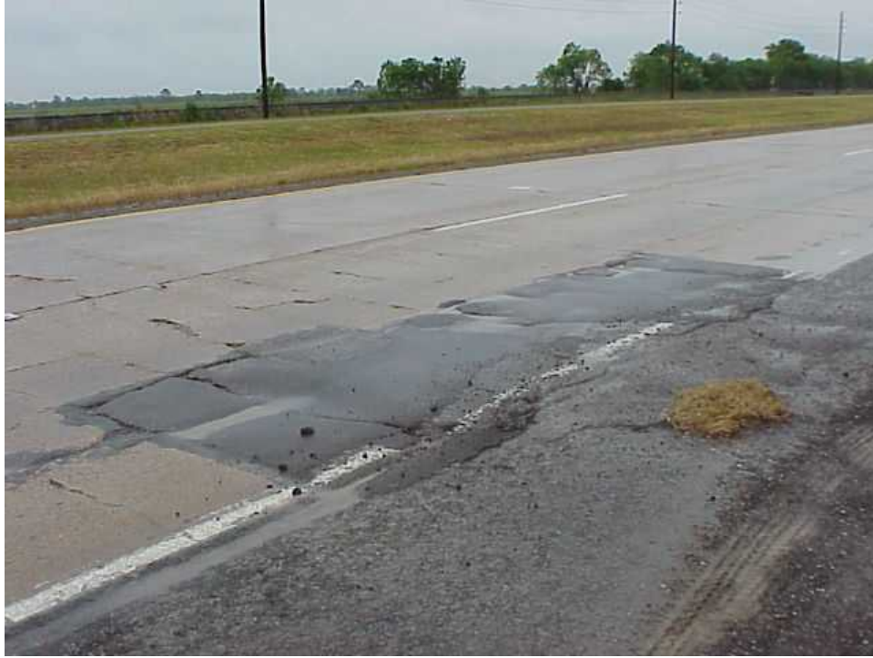
Figure 46 – Failures (asphalt patch)
