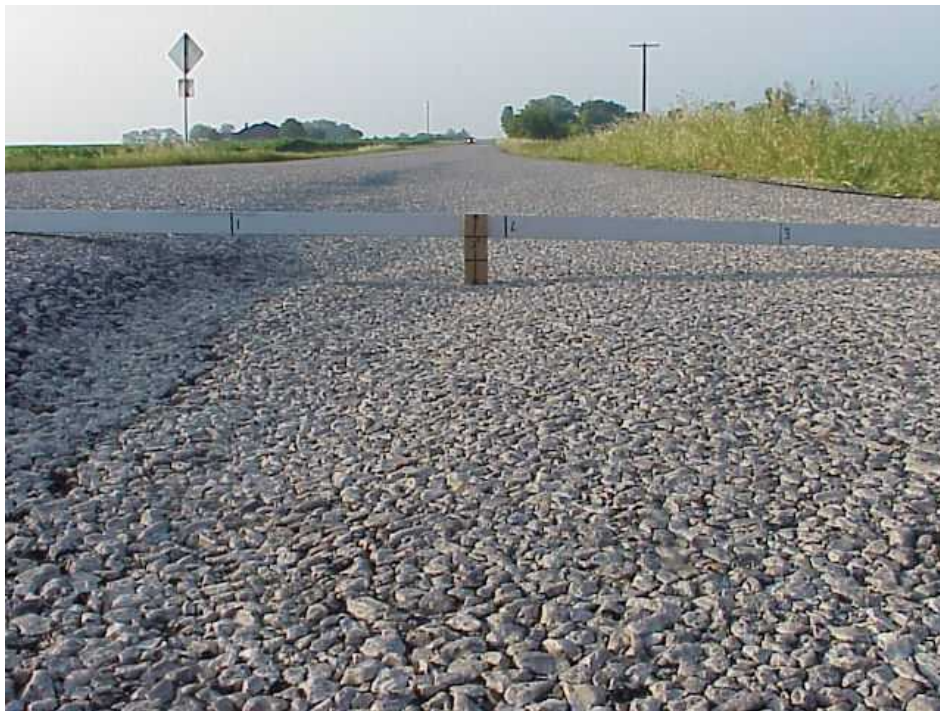
Figure 16 – Severe Rutting
