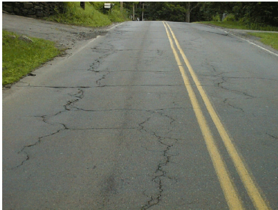
Figure 22 – Block Cracking
