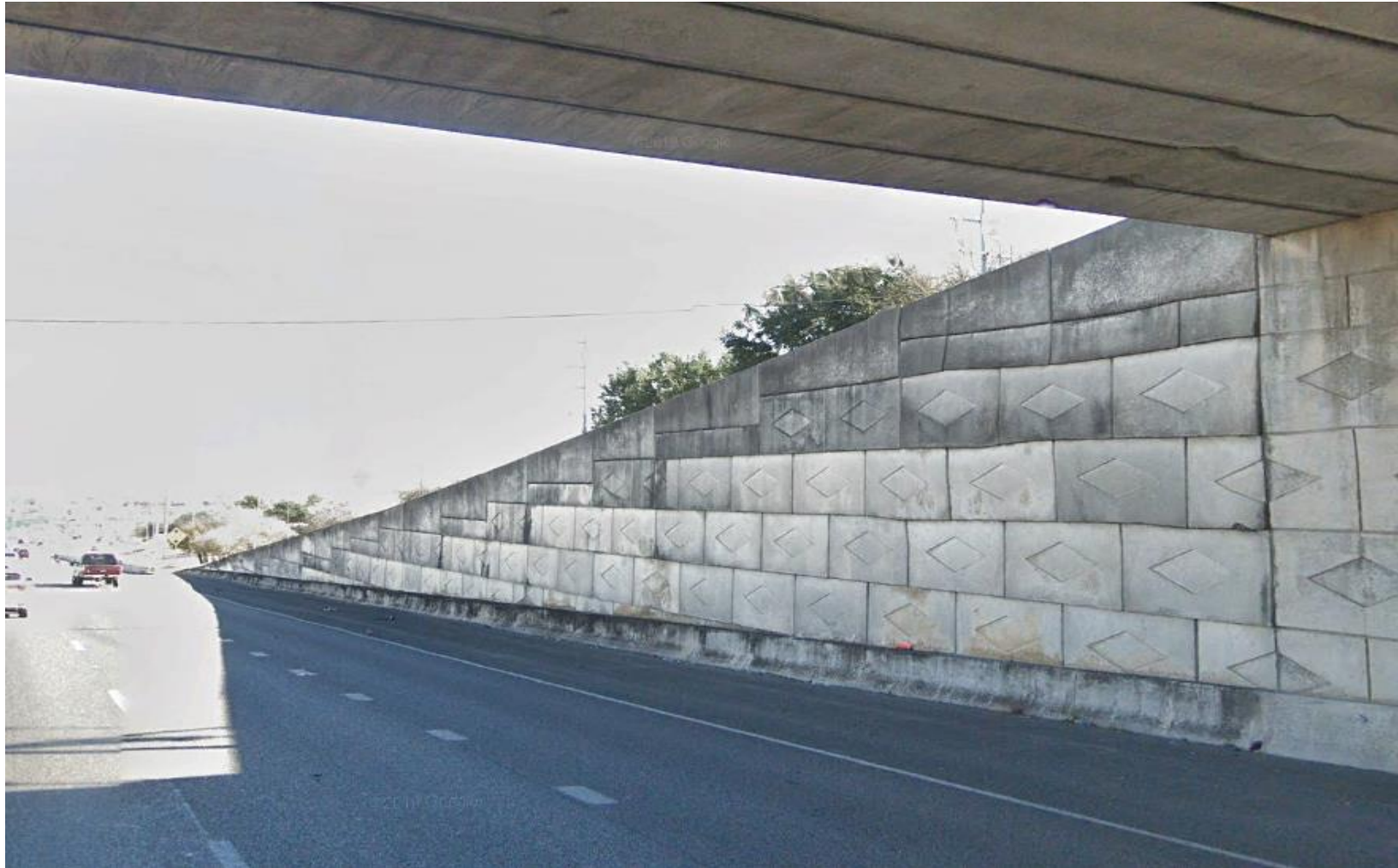
As-Built Plan Wall Type: Spread Footing CIP Cantilever In-Place Wall Type: Likely Doublewal
