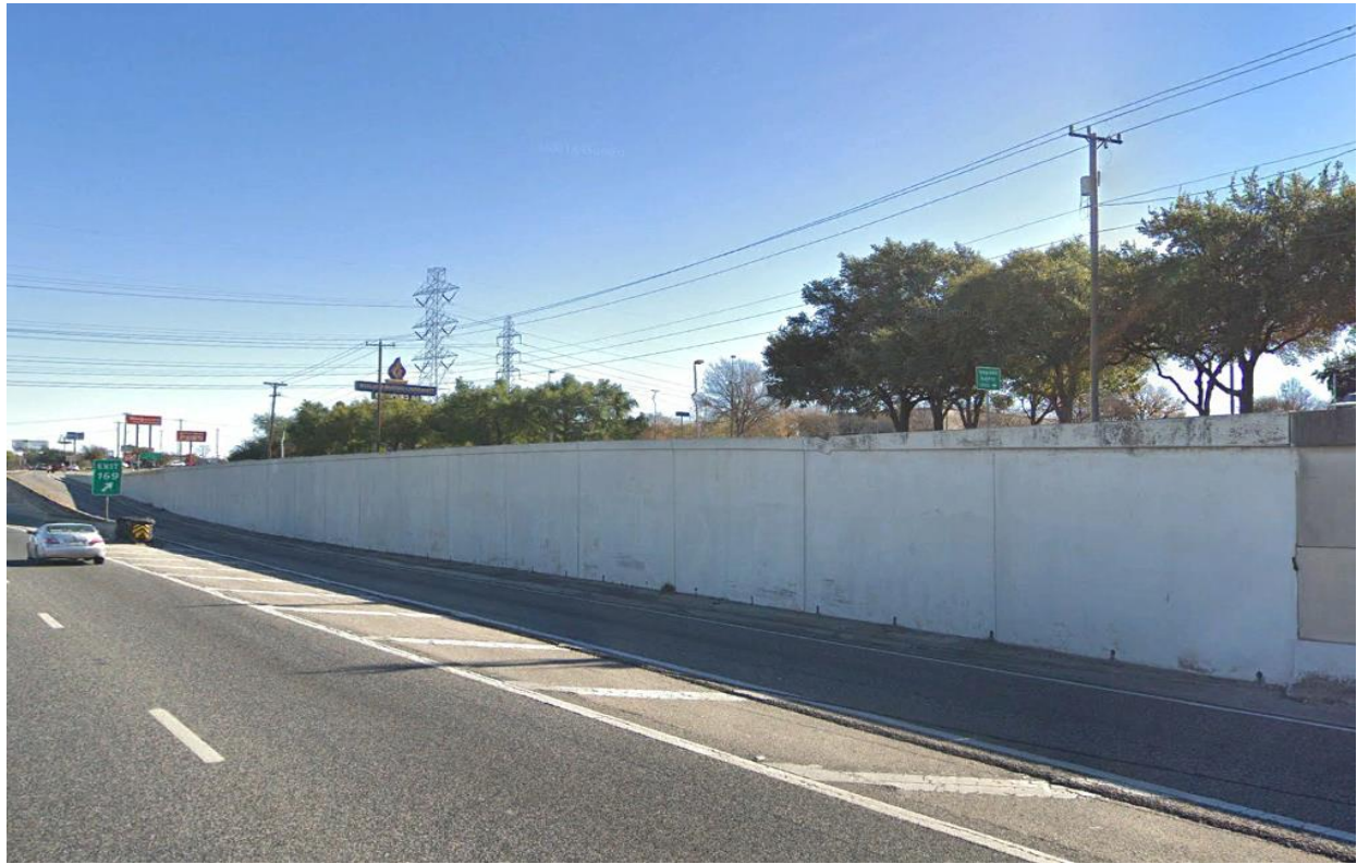
As-Built Plan Wall Type: Spread Footing CIP Cantilever In-Place Wall Type: Same as as-Built
