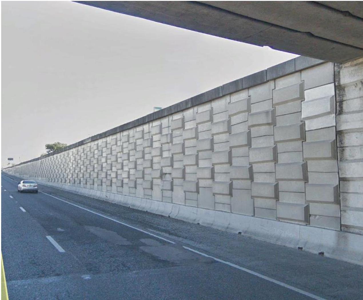
As-Built Plan Wall Type: Spread Footing CIP Cantilever In-Place Wall Type: Likely MSE Wall
