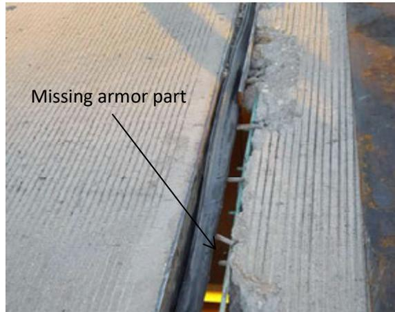
**Figure 3-10: Example of a failed joint.**
