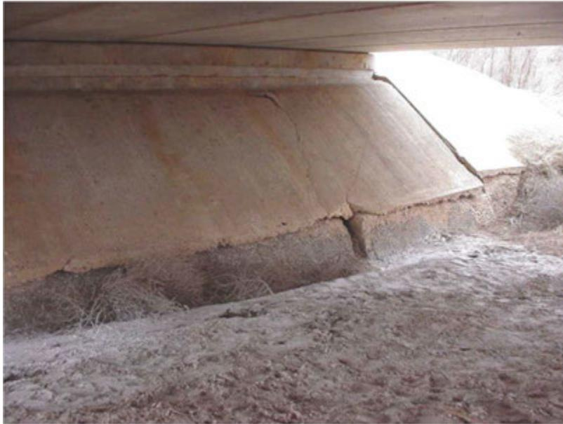
**Figure 13-4: Concrete Riprap – Undermining at Toe. Note that the current CRR standard required a deeper toe than shown here.**
