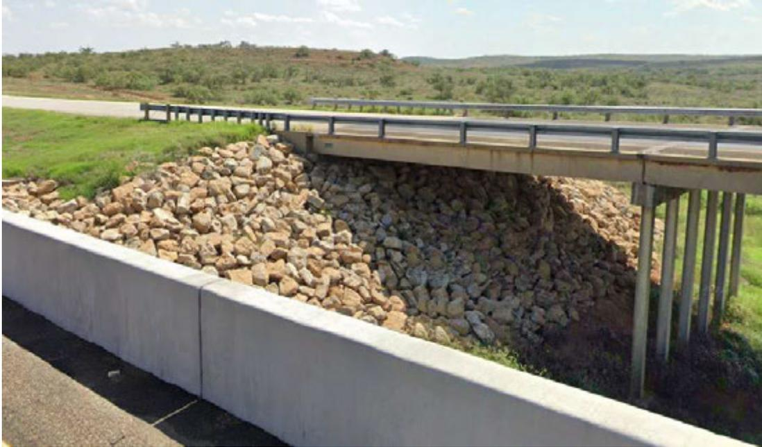
**Figure 13-24: SRR used to replace a failed CRR.**
