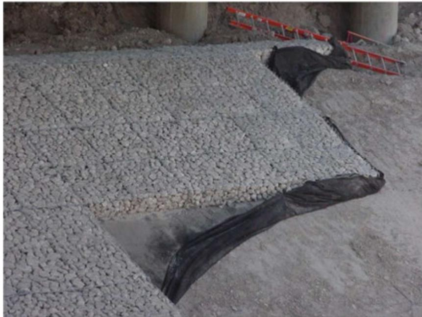
**Figure 13-15: Gabion Mattresses at Bridge Abutment**
