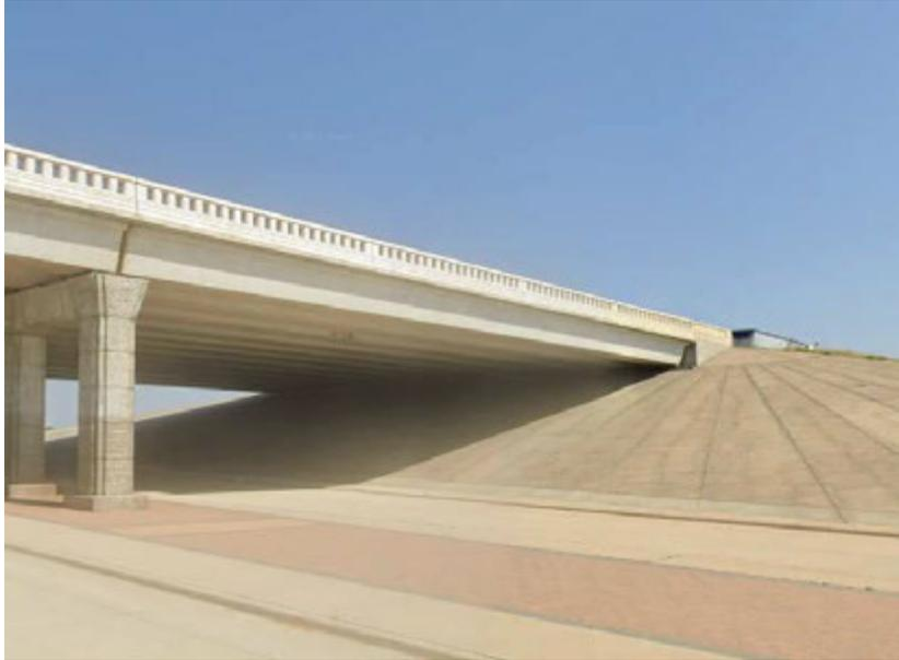
**Figure 13-1: Concrete Riprap under Bridge Abutment**
