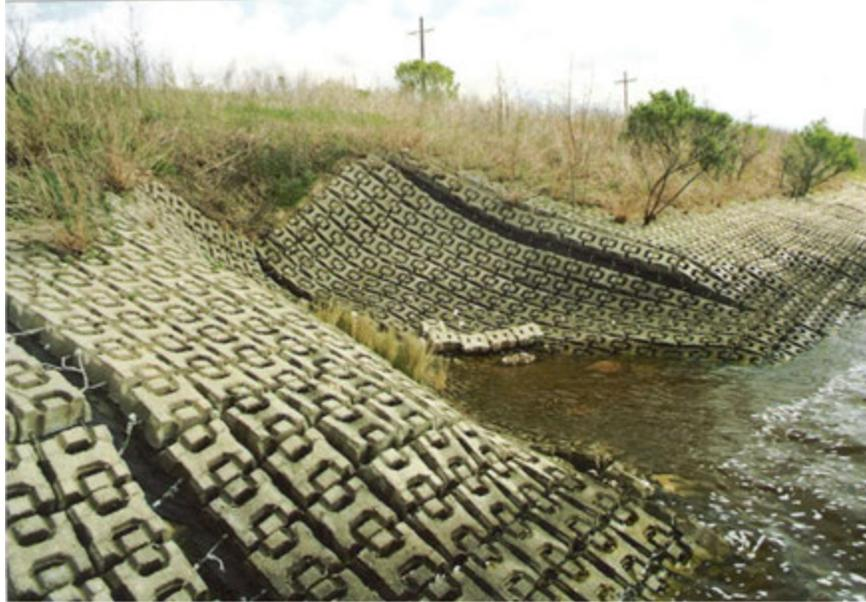
**Figure 13-22: Interlocking Articulated Concrete Blocks – Settlement**
