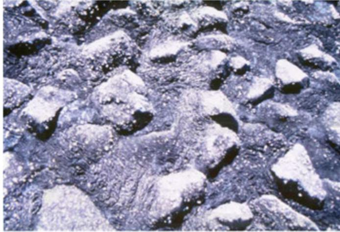
**Figure 13-2: Grouted Stone Protection – Rough Surface**
