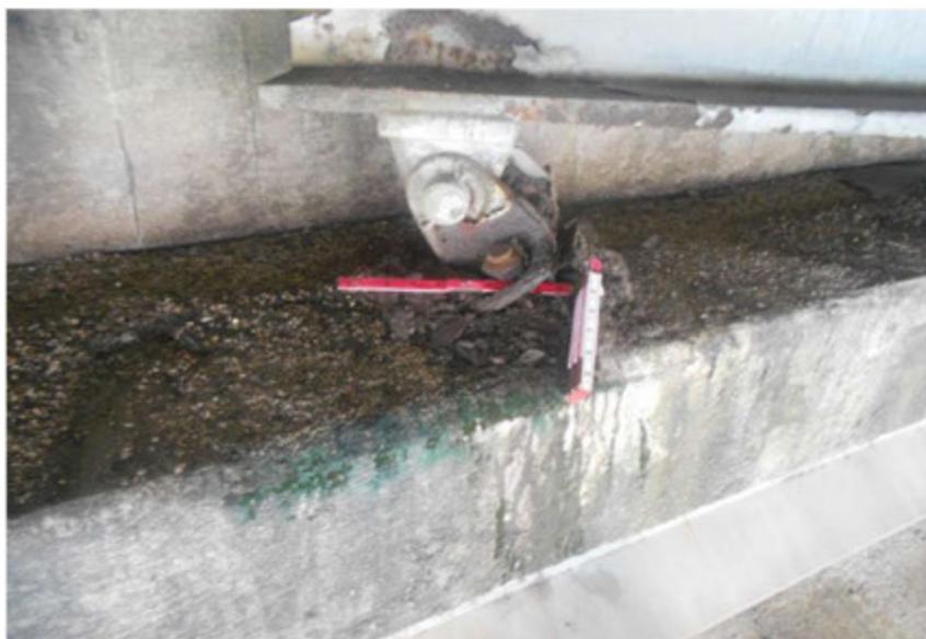
**Figure 6-13. Example of rocker bearing requiring replacement**
