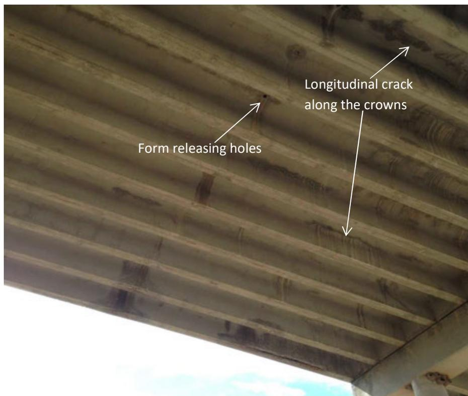
**Figure 4-5: Longitudinal Cracks on pan girders.**
