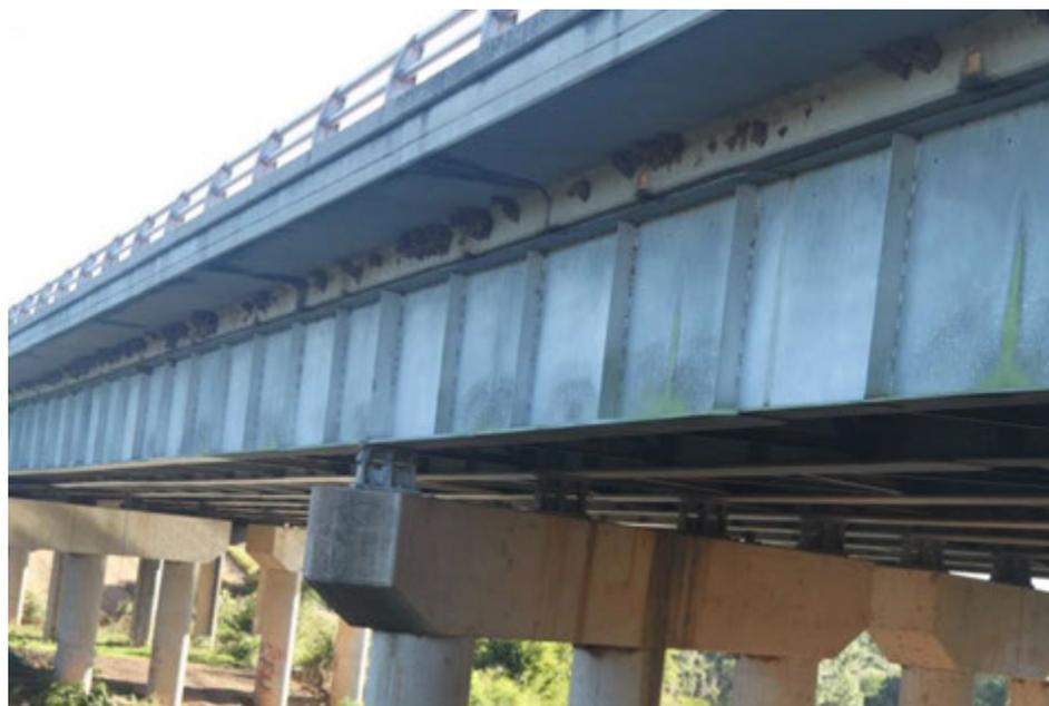
**Figure 6-7: Example of candidate steel superstructure for overcoating.**
