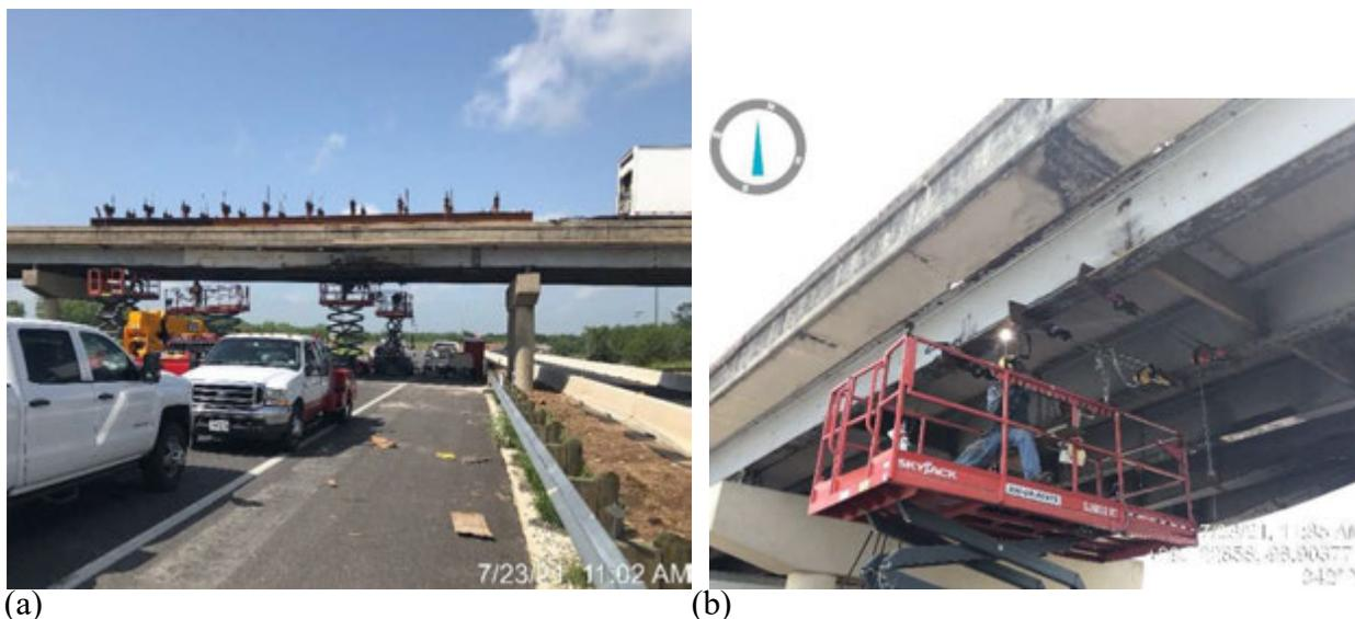
**Figure 6-6: Examples of Overheight Impact Damage Repair: (a) Beam replacement with a Beam strongback on SW exterior beam of a bridge on SB IH35 at FM 3176 (b) Heat straightening for beams of bridge on SB IH35 at FM 3176**
