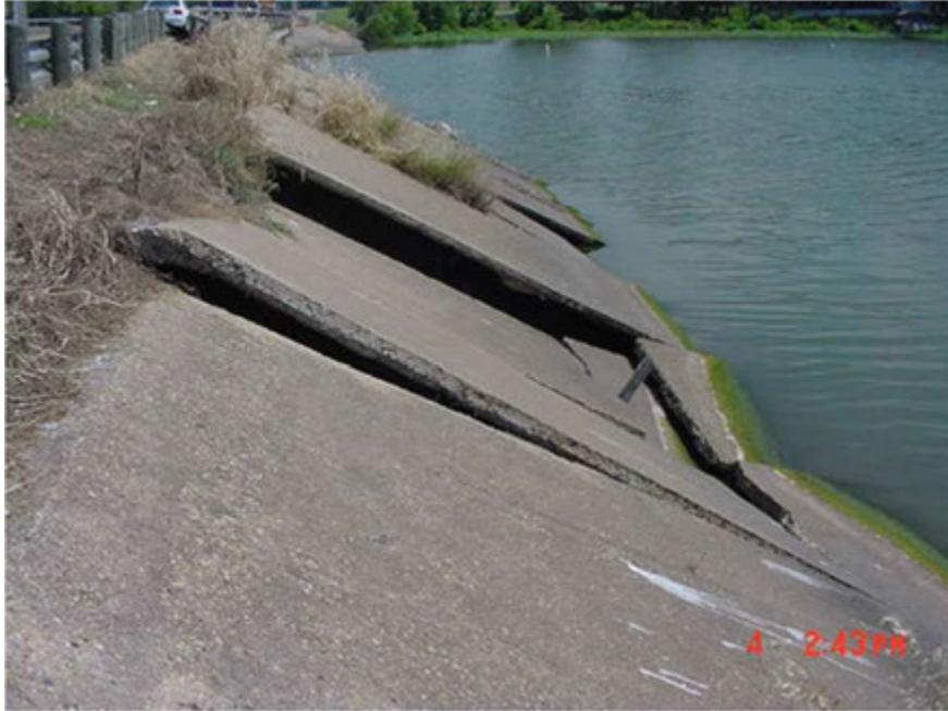
**Figure 13-5: Concrete Riprap - Undermining and Settlement**
