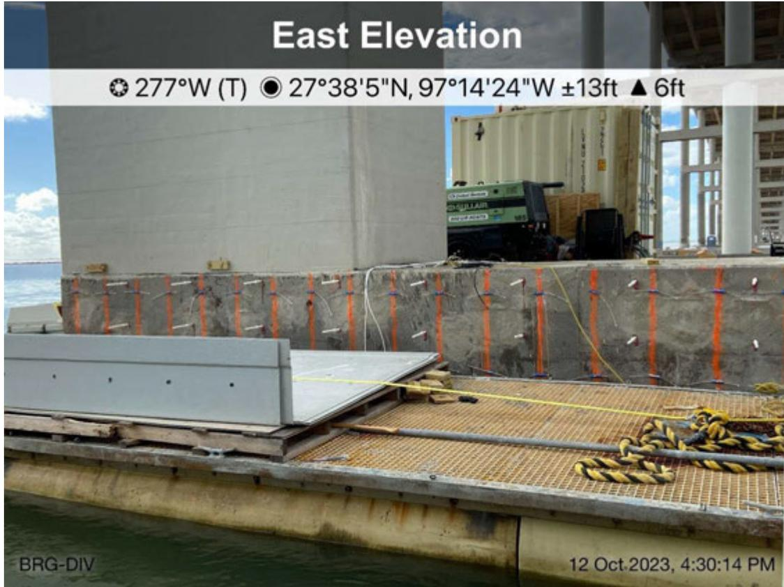
Figure 12-1: Installation of Cathodic Protection System on the substructure of the JFK Causeway
