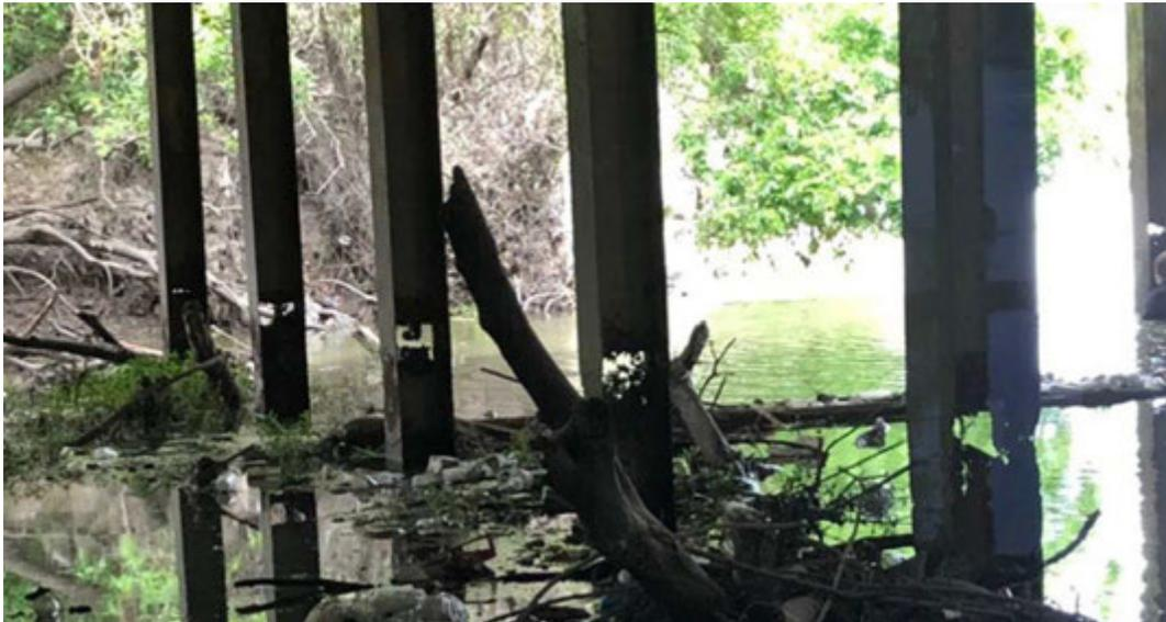
**Figure 8-1. Severe steel section loss on multiple piling triggering a critical finding requiring emergency repair contract work.**
