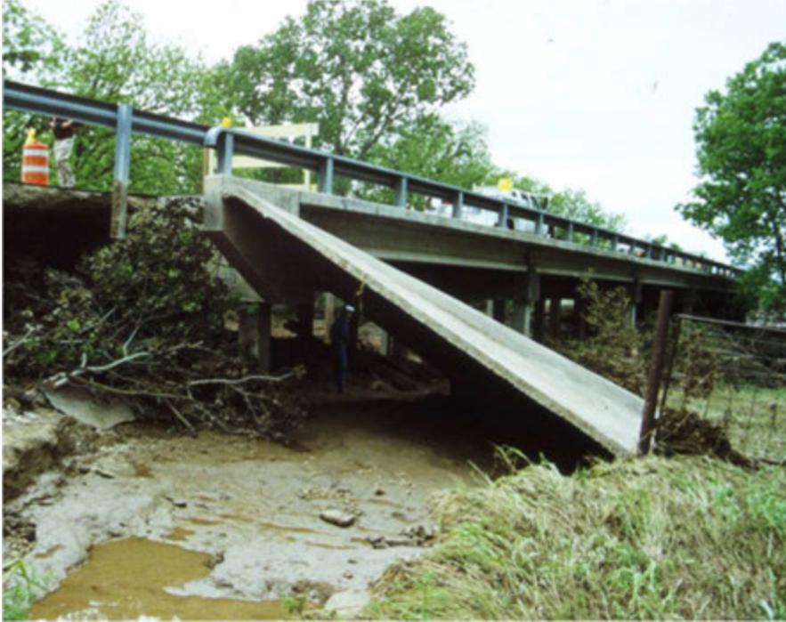
**Figure 13-7: Concrete Riprap - Loss of Supporting Soil**
