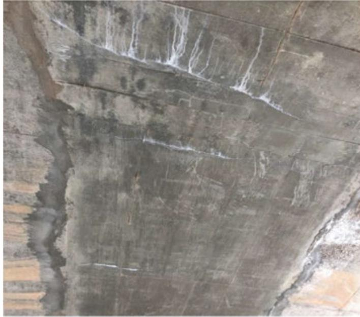
**Figure 4-1: Transverse cracks and white efflorescence on slab soffit.**
