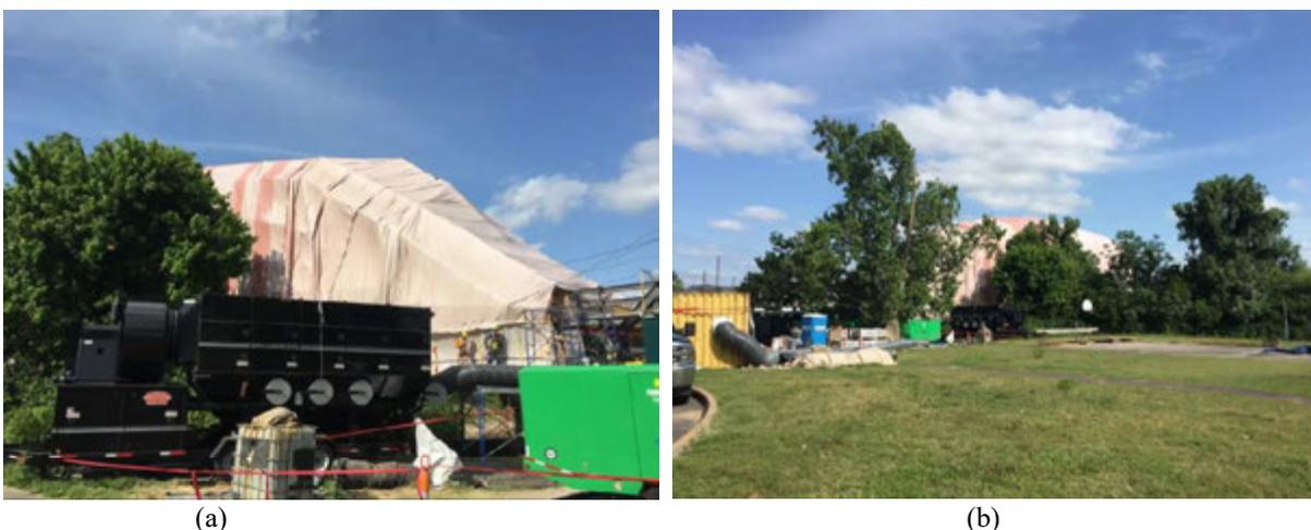
**Figures 6-9. Recycled abrasive media recycling (a) and containment (b) on Wharton Truss.**
