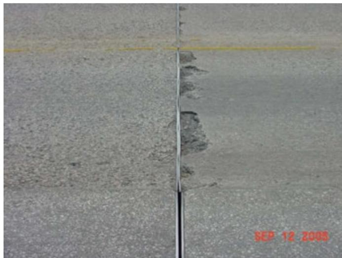
**Figure 3-11: Example of closed-up armor joint.**
