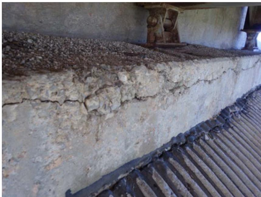
**Figure 6-12. Example of rocker shoes requiring resetting, but not replacement.**
