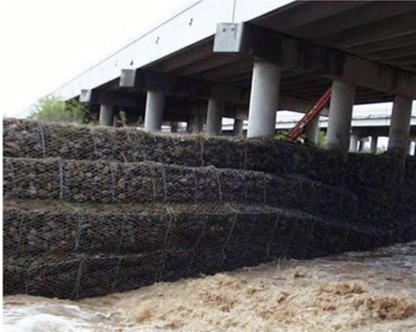
**Figure 13-23: Gabions – Undermining and Settlement**
