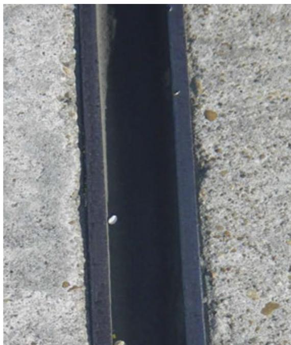
**Figure 3-6: Example of silicone seal.**
