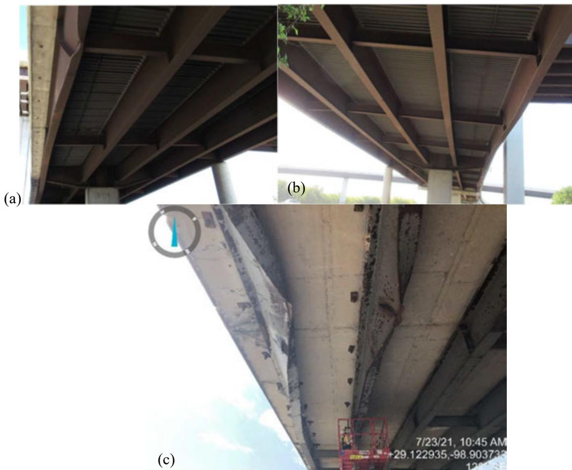
**Figure 6-5: Examples of Overheight Impact Damage on: (a) SW exterior beam for IH 610 EB (b) diaphragm on span 14 and 15 of IH 610 EB (c) exterior beams of bridge on SB IH35 at FM 3176**
