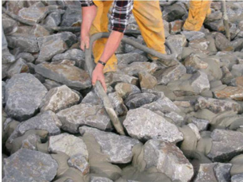
**Figure 13-9: Partially Grouted Riprap**
