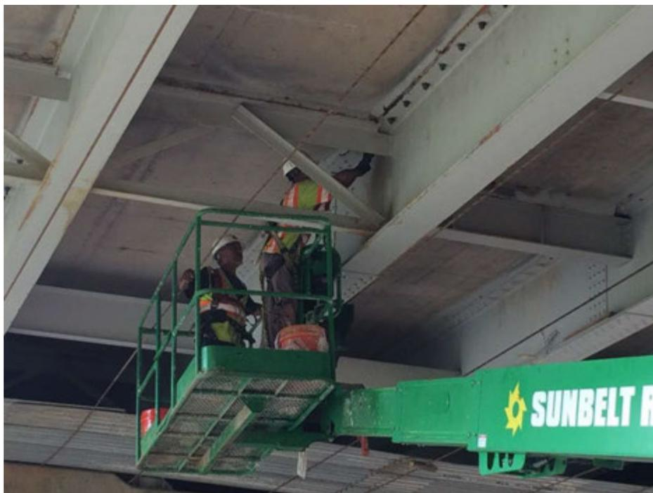
**Figure 6-11. Installation of Post-Installed Shear Connectors.**
