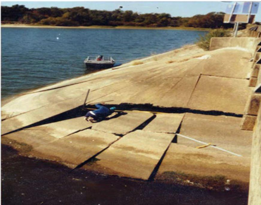
**Figure 13-6: Concrete Riprap - Settlement Cracks**
