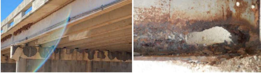
**Figure 3-1: (a) Cap face spalling due to restricted movement; (b) Severe web corrosion due to debris build up on cap.**
