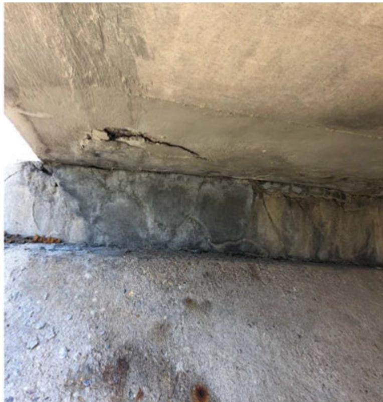
**Figure 4-2: Slab soffit spalling due to corrosion of steel reinforcement.**
