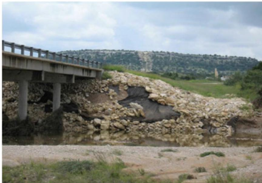
**Figure 13-21: Stone Protection Riprap Compromised**
