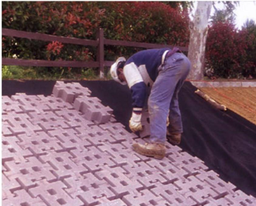
**Figure 13-11: Interlocking Articulated Concrete Blocks**
