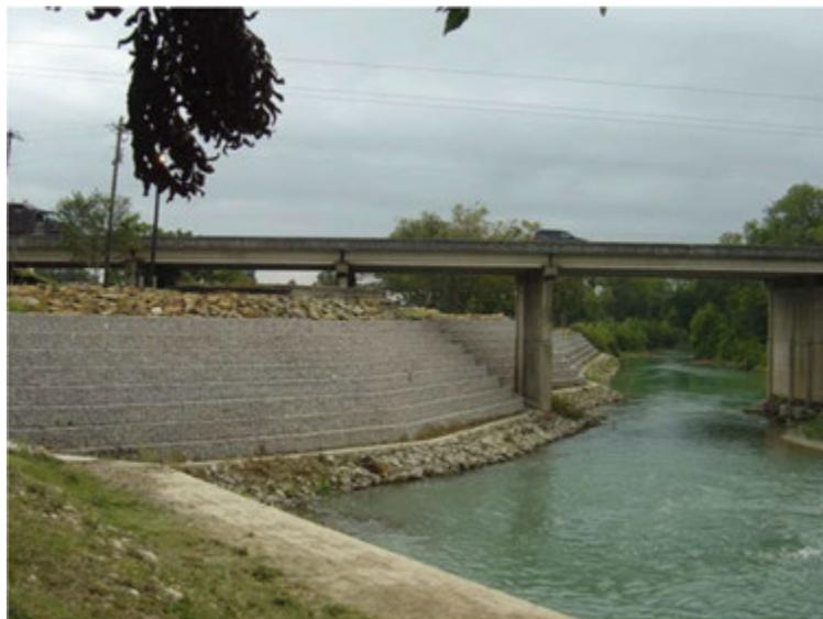
**Figure 13-13: Gabions - Channel Bank Protection**
