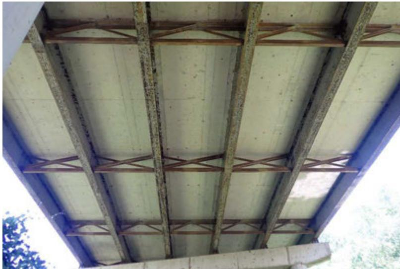
**Figure 6-2: Paint failure of steel beams.**
