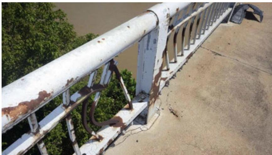
**Figure 9-1: Damaged Type PR-1 (MOD) railing.**
