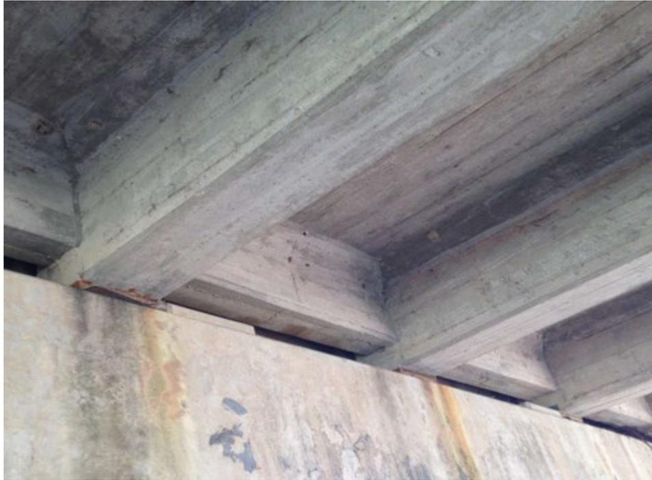
**Figure 4-6: Lead sheet Slip.**
