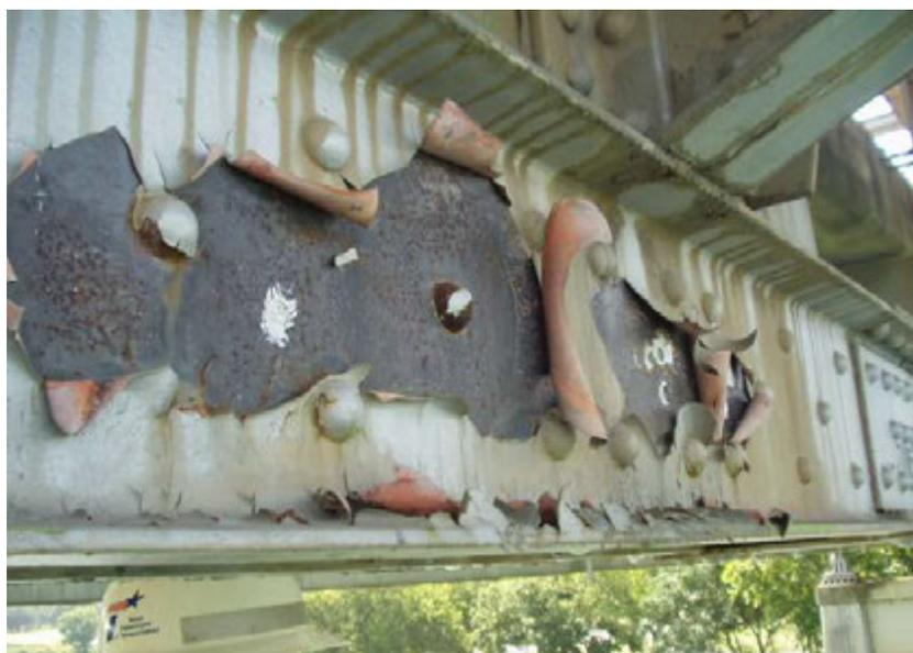
**Figure 6-8: Example of candidate for blast and repaint.**
