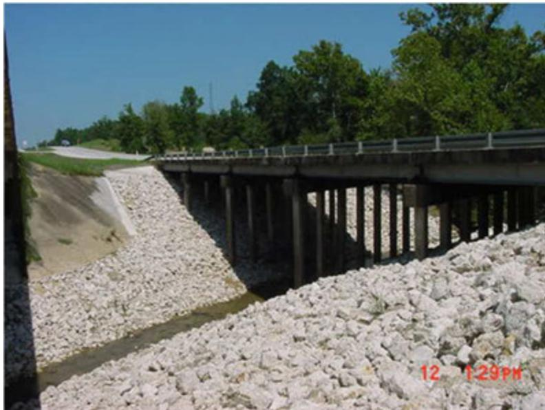
**Figure 13-8: Stone Protection Riprap at Bridge Abutment and Pier**
