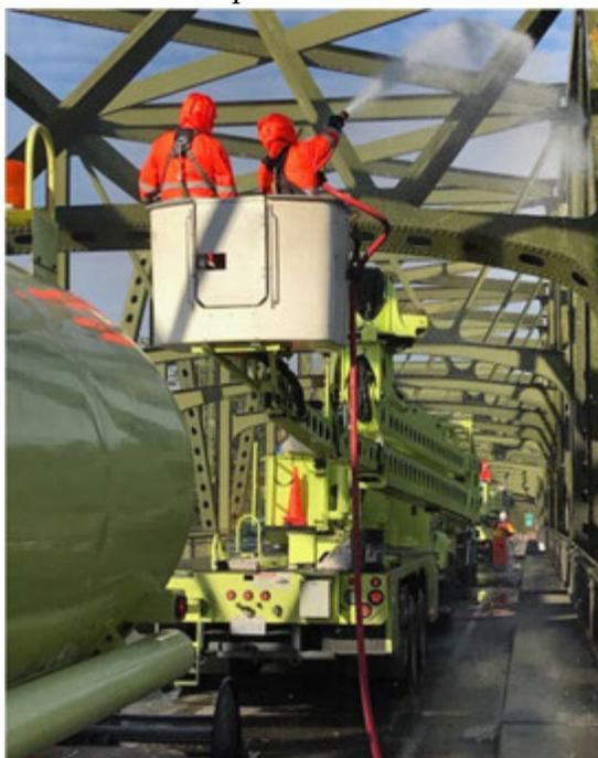
**Figure 2-5: Bridge Deck Washing (Source: FHWA Bridge Preservation Guide)**
