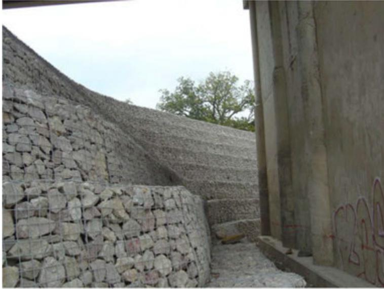
**Figure 13-14: Gabions at Bridge Pier *Gabion Mattress***
