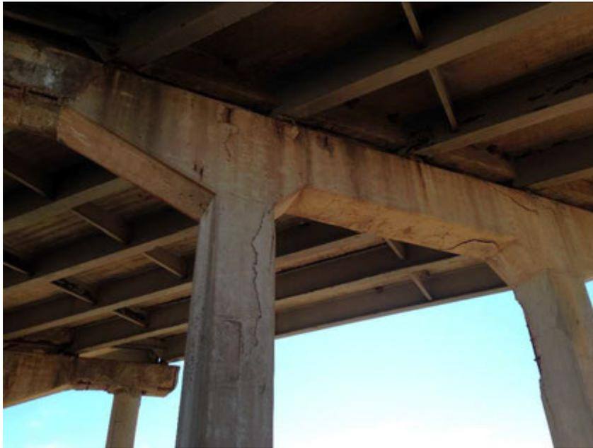
**Figure 7-1. Example of concrete substructure deterioration.**
