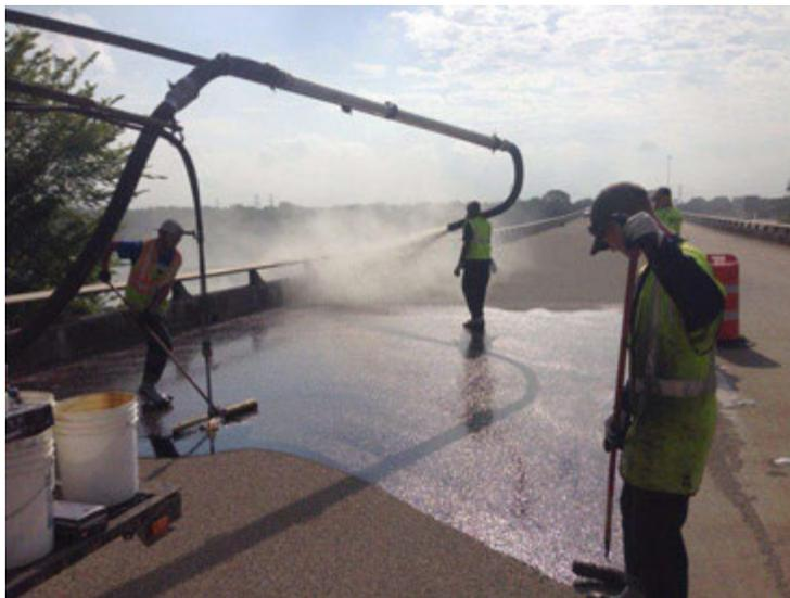
**Figure 2-3: Application of overlay on SH 31 WB over Trinity River.**
