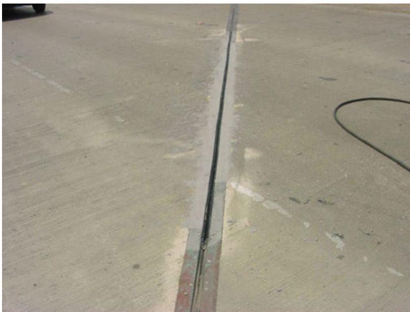
**Figure 3-12: Example of partial elimination of armor joint.**
