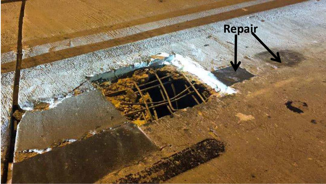
**Figure 2-1: IH35 Bridge Deck Failure**
