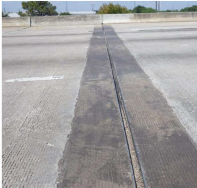
**Figure 3-4: Example of retrofitted strip seal joint.**
