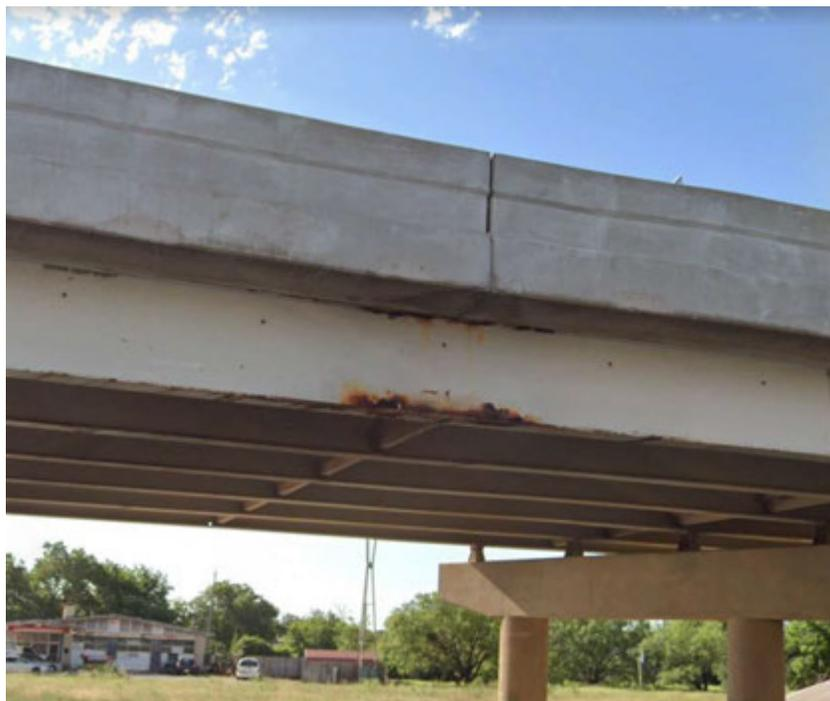
**Figure 3-13: Example of opened construction joint.**
