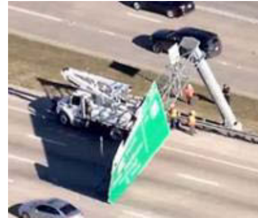
Collapse of Cantilever Structure—Hwy 75, Allen, TX
