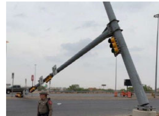
Collapse of Cantilever Structure—Odessa, TX
