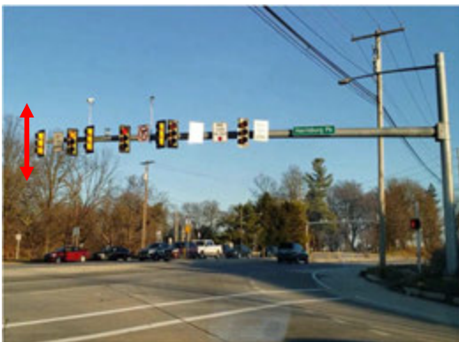
Mast arm vibration (TSS/COSS)
