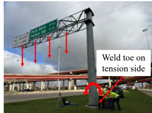
Common crack location of COSS
