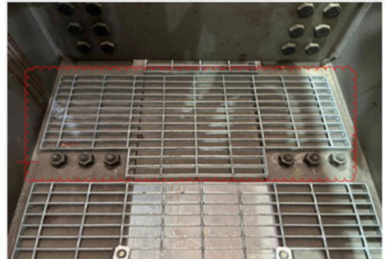
Grating fabricated over a bearing sole plate where it is not needed.
