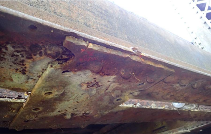
Bottom batten plate at midspan with 1- 3/4 inch long crack.
