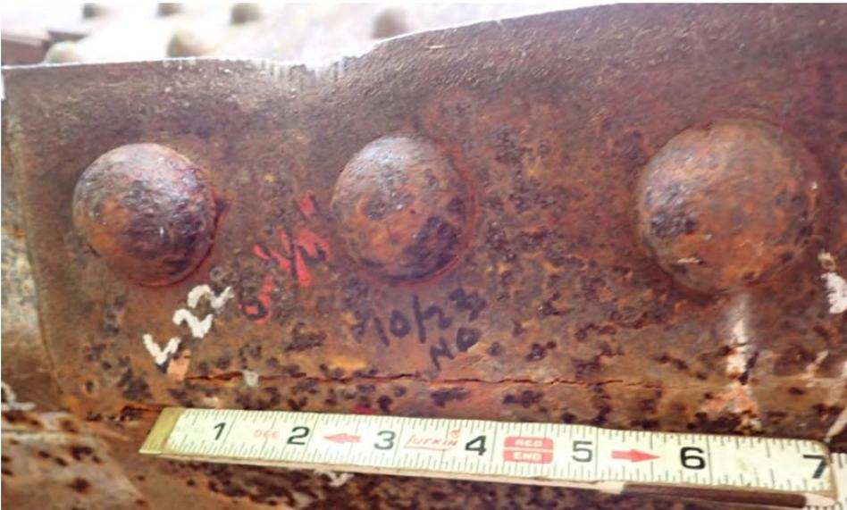
Underside of cover plate at L5 with 6- 1/8 inch long crack.
