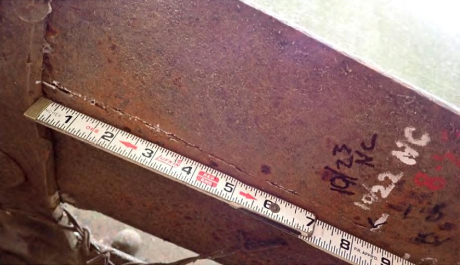
Underside of exterior angle with 8- 1/4 inch long crack.
