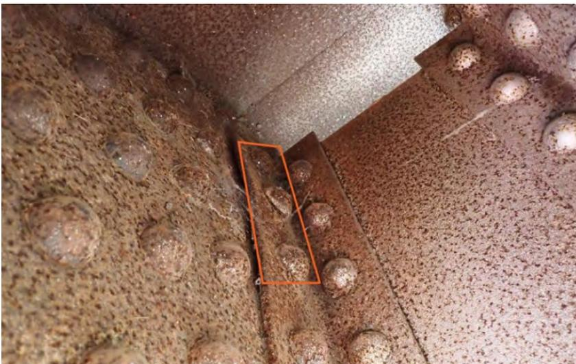
Three poorly seated rivets show corrosion with section loss at the vertical angle and gusset plate on the East truss. This repair can be completed after moving the truss and can be deferred further if needed. However, corrosion will continue until addressed by cleaning, painting, and sealing areas of deformation where water will collect. TxDOT highly recommends cleaning and painting the entire structure.
