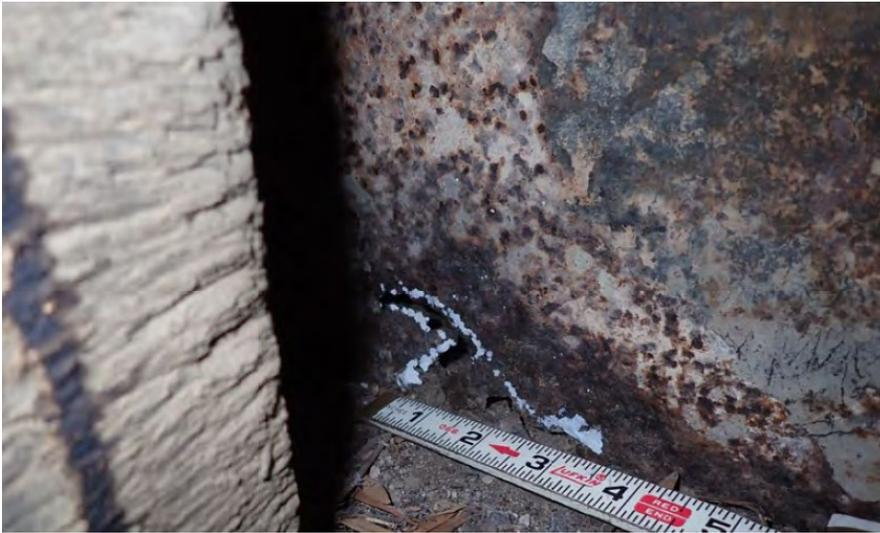
Underside of exterior angle with 1- 3/16 inch long crack.
