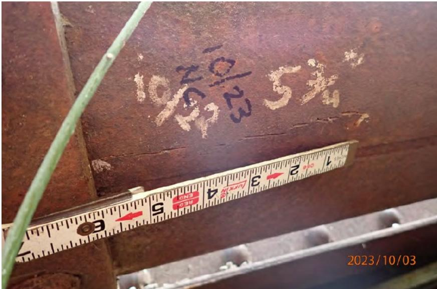
Bottom flange angle at midspan with 5- 3/4 inch long crack.
