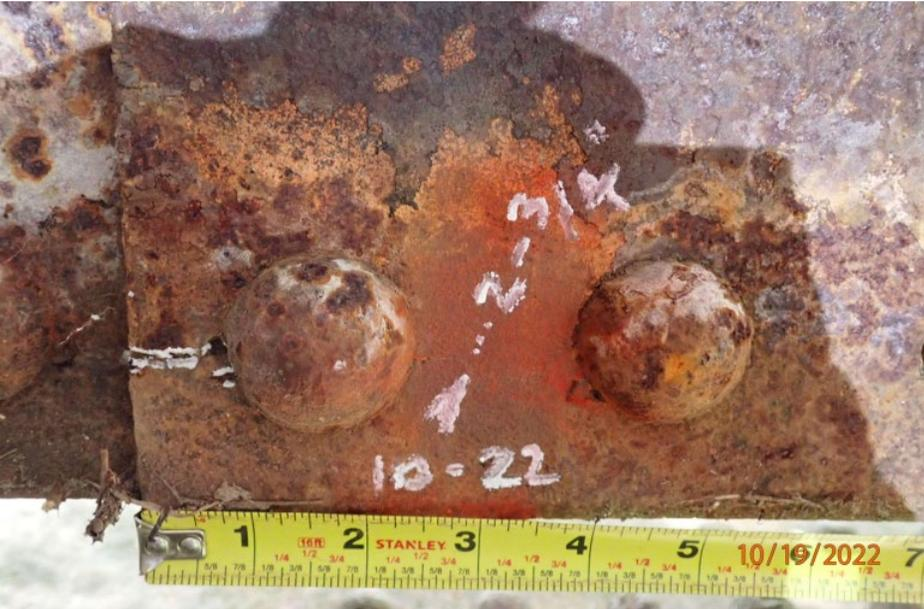
Underside of bottom flange splice plate near L2 with 2- 3/4 inch long crack.
