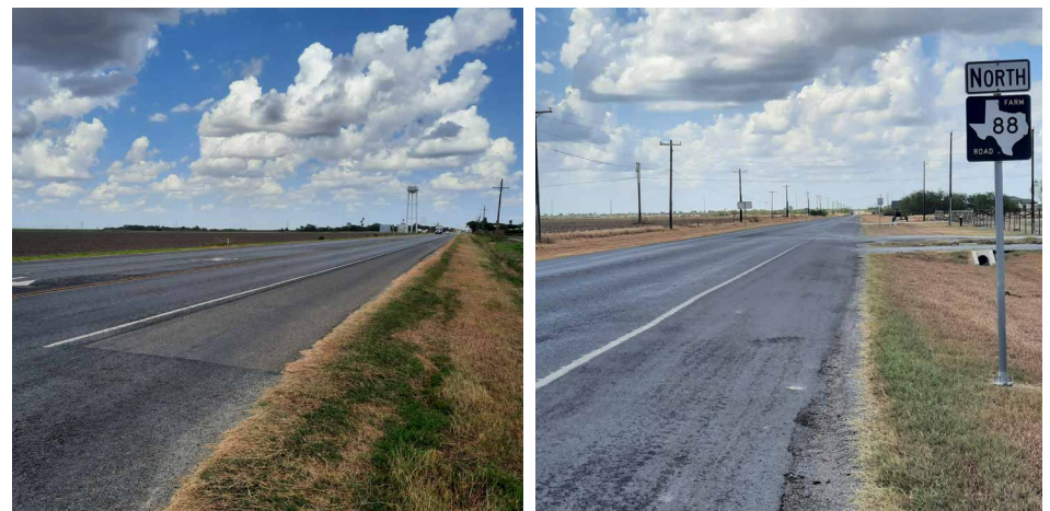
Figure 1. Bikeable shoulders along U.S. Highway (US) 281 Near the Santa Ana National Wildlife Refuge (Left) and Farm to Market Road FM 88 (Right)
