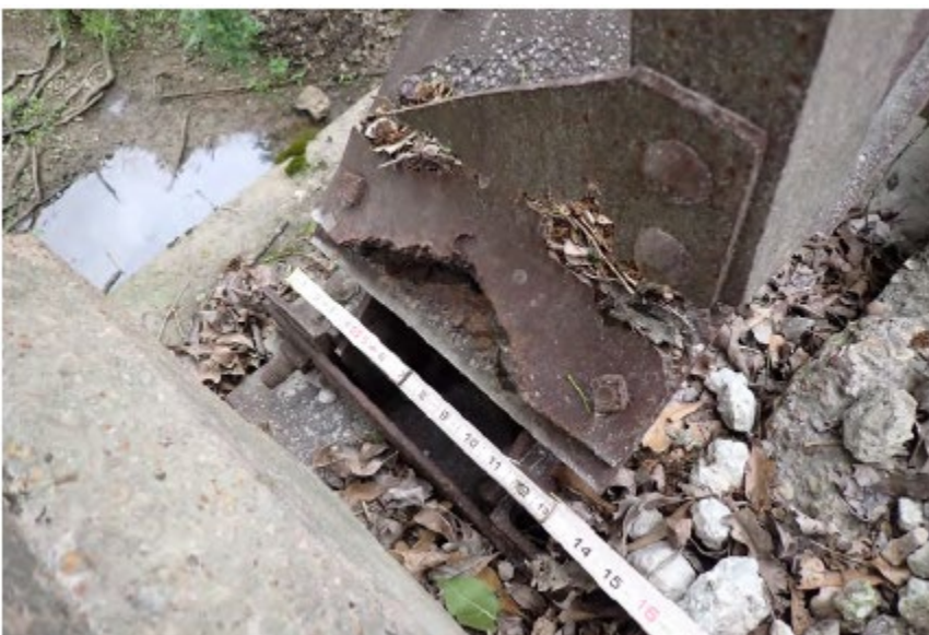
Photo 5: Truss End Cover Plate
