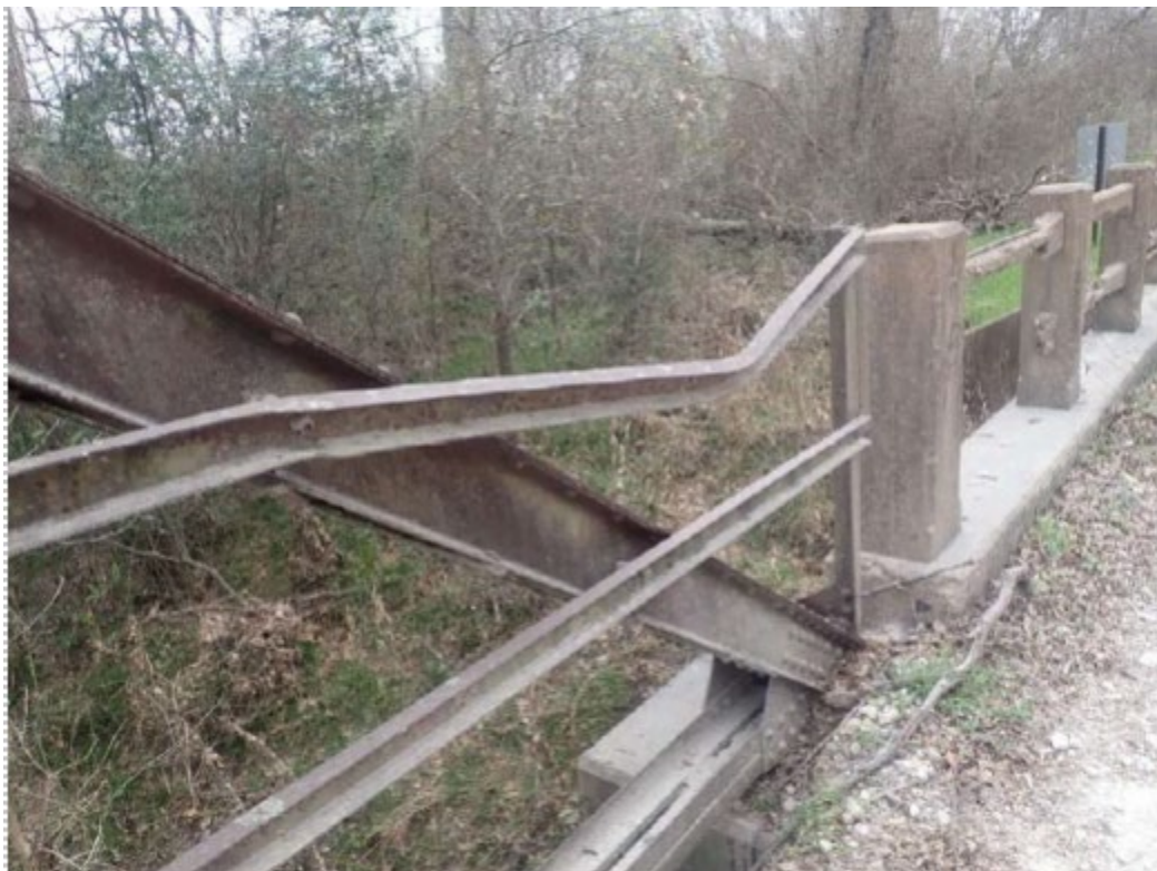
Photo 6: Existing truss railing
