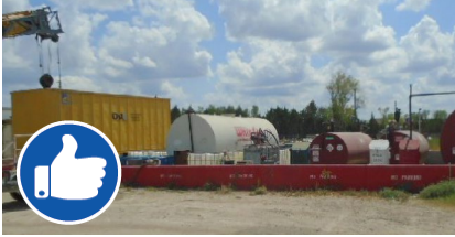
Proper use of secondary containment.
