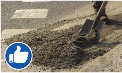
Remove sediment from road.
