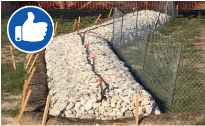
Properly installed check dam using a rock filter dam.
