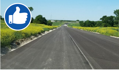
Properly installed vegetation – root system is well established.
