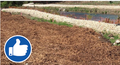
Properly laid mulch – uniform layer with appropriate depth.
