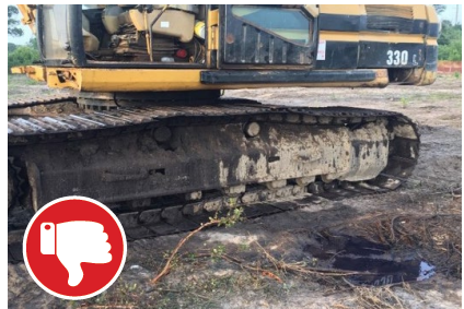
An obvious leak has not been addressed – clean up should already be in place. Always address spills as soon as possible. Drip pans can be placed under the vehicle overnight while parked as a secondary containment.
