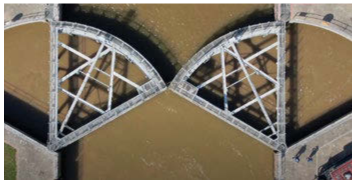
Top and Bottom: Brazos River Flood Gates (Photo credits: TxDOT)
