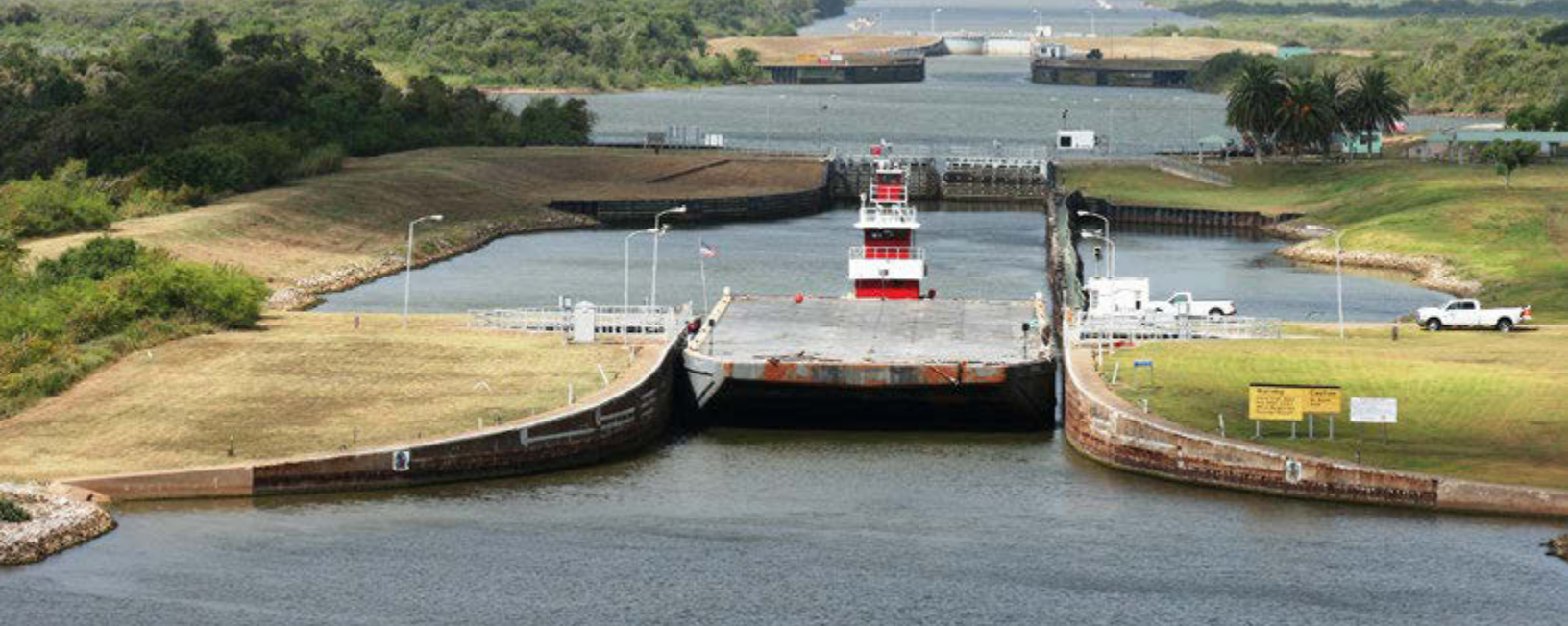
A 72-foot-wide barge navigates through the USACE Galveston District's 75-foot-wide Colorado River Locks in Matagorda, Texas. (Photo credit: USACE)
