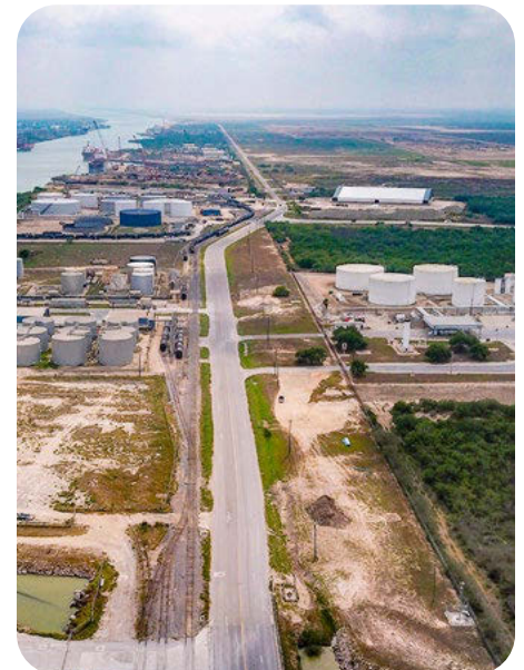
East Ostos Road at the Port of Brownsville
