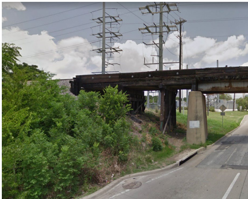
Figure 3-19: TRE Bridge over Inwood Road
