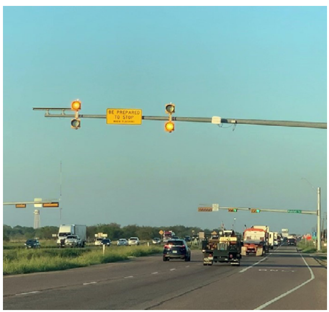
Figure 1. Installation of overhead W3-4 sign and flashing beacon.
