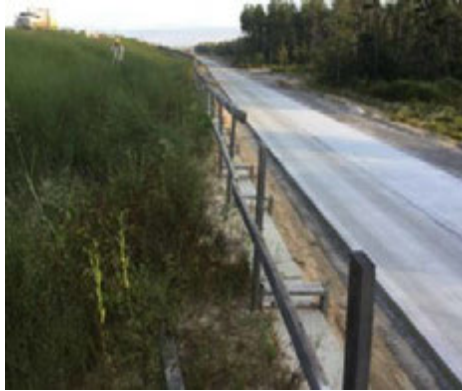
Figure A.1: Cement Treated Base in Segment H1B
