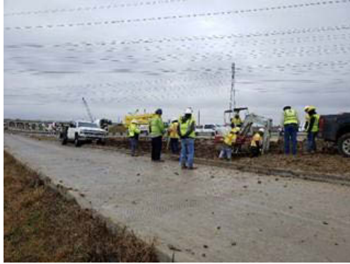
Figure A.10: Drilling for ITS Pole in Segment I2B1
