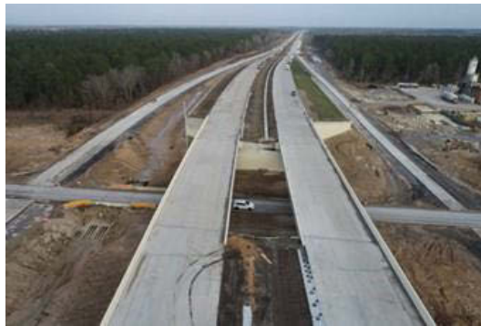
Figure A.2: View of Completed Bridges in Segment H1C
