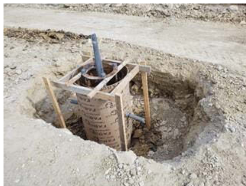
Figure A.9: Illumination Foundations in Segment I2A1
