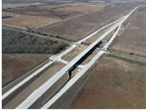
Figure A.7: Completed Pavement of Ramps 13C and 13A in Segment I1A
