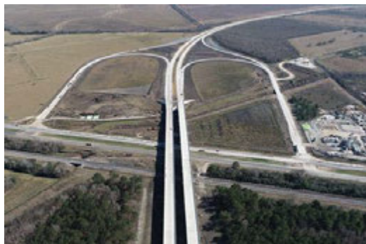
Figure A.6: US90 Ramps in Segment I1A
