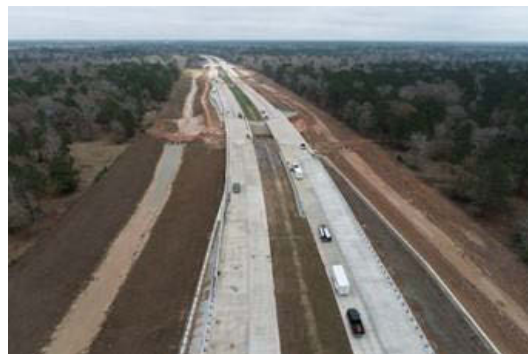
Figure A.3: Metal Beam Guardfence Installation in Segment H1C
