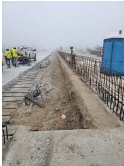
Figure A.11: CRCP in Segment I2B2
