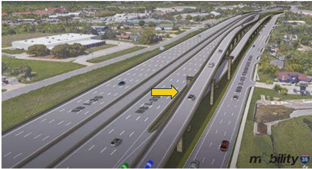
Figure 2- Braided ramp on Mobility35 project
