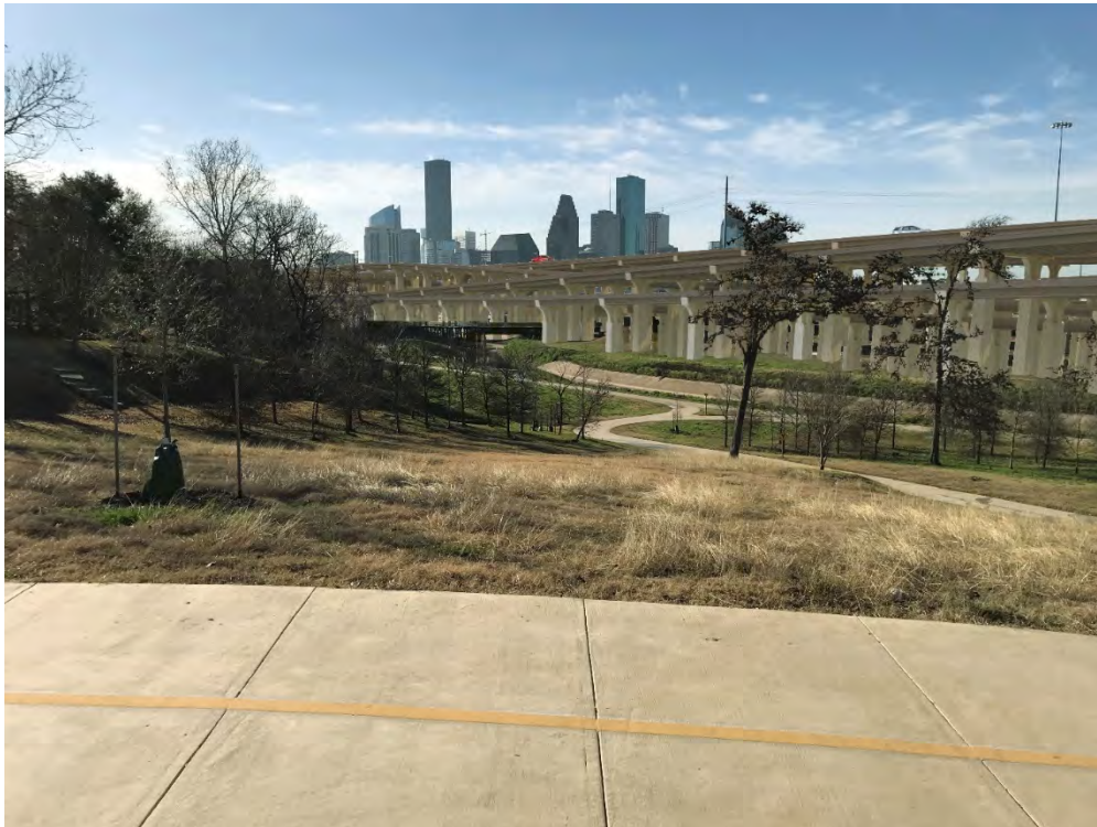
Figure 10: Hogg Park at White Oak Bayou Greenway Trail – Proposed NHHIP (130 foot average bridge spans)
