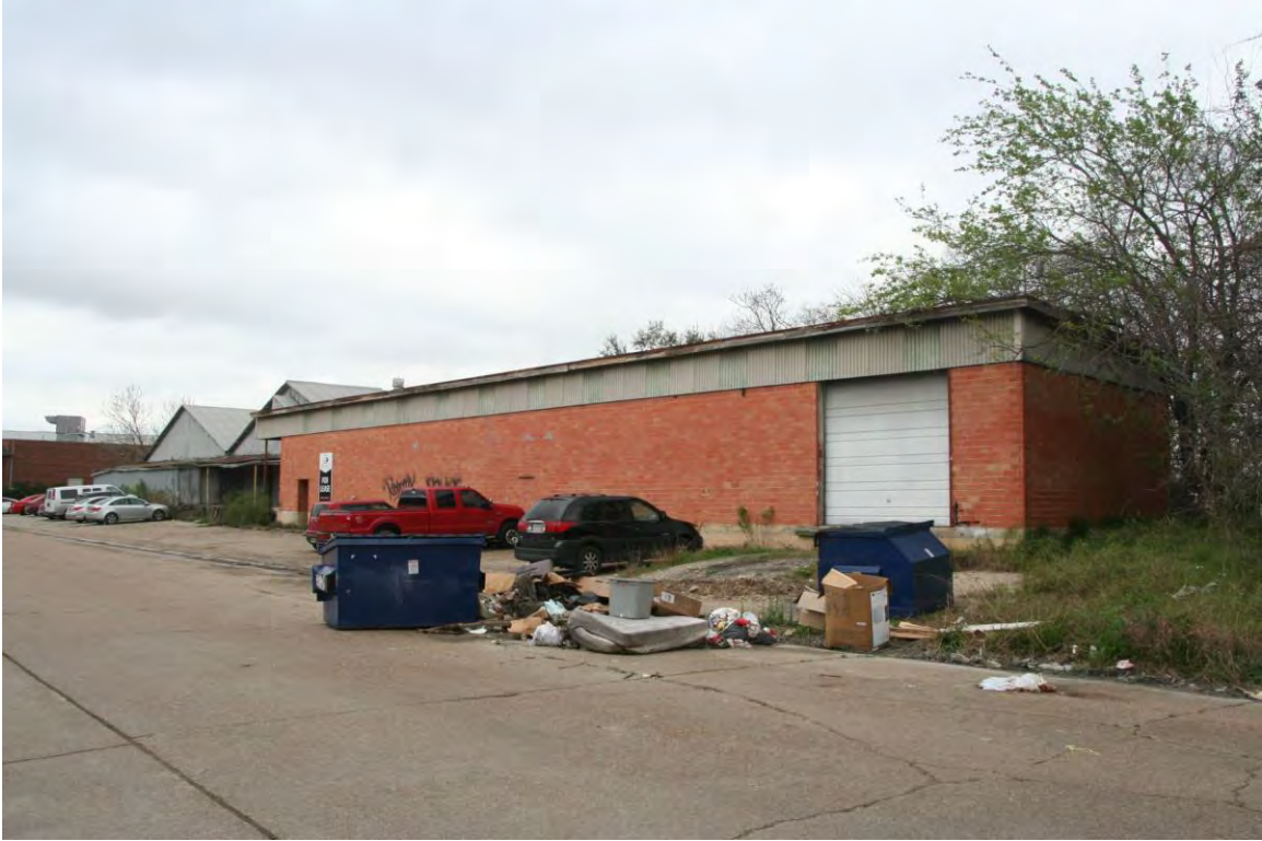
View facing northeast, showing Carlisle Plastic South Warehouse. North warehouse in left background.
