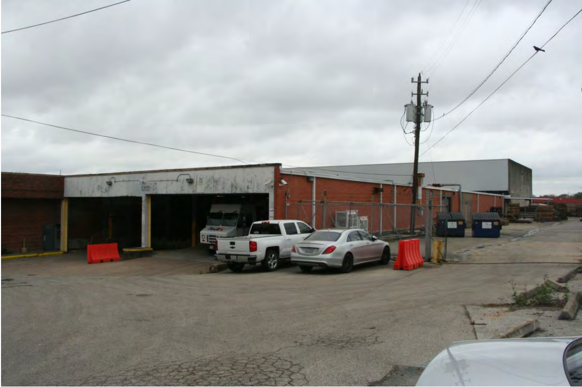
View facing north-northwest, showing loading docks on southeast corner of Readers Warehouse. Note 1998 rear addition in background of frame.
