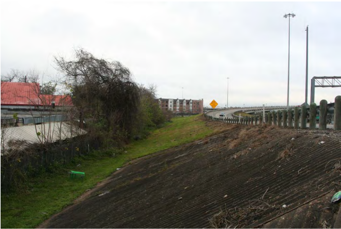
View facing east-northeast, showing existing northbound SH 288-to-southbound IH 69 ramp at right and east edge of Rossonian Cleaners property at left.
