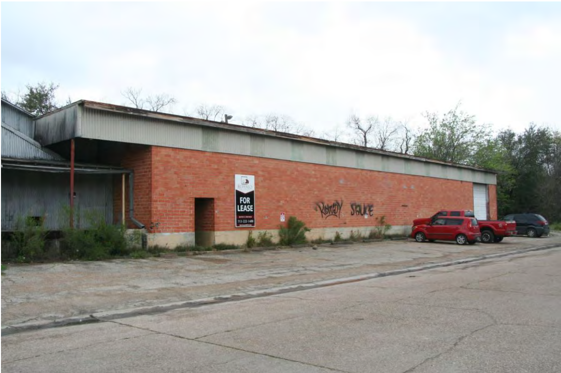
View facing southeast, showing north side of Carlisle Plastics South Warehouse.
