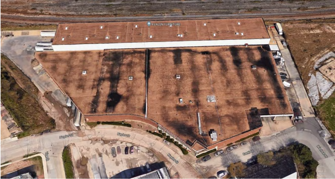
Birds-eye view of Readers Warehouse facing north. Image courtesy Google.
