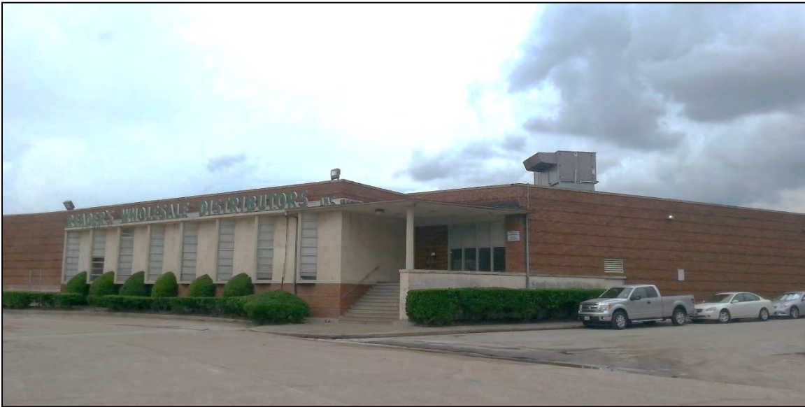
Photo 3-2. Readers Distributors Warehouse, Front (south) facade facing northeast.
