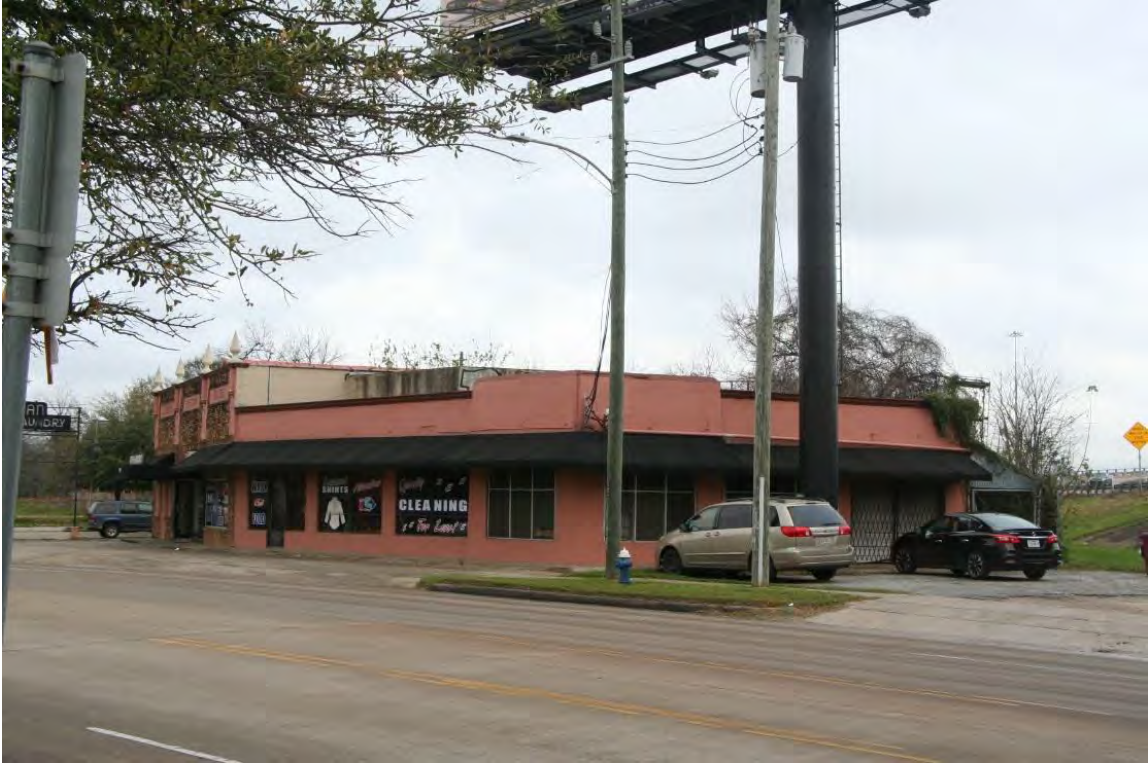
View facing northeast, showing Rossonian Cleaners building and adjacent parking.
