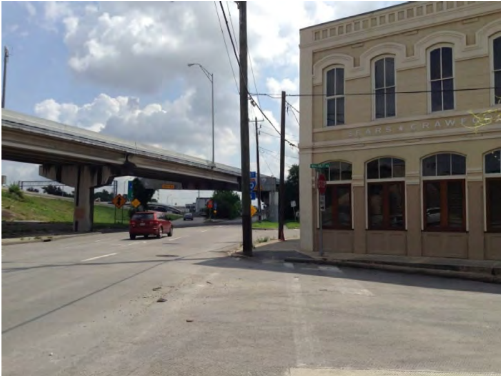
View facing east at intersection of Rothwell Street, Walnut Street, and Nance Street. Existing IH 10 at left of frame.
