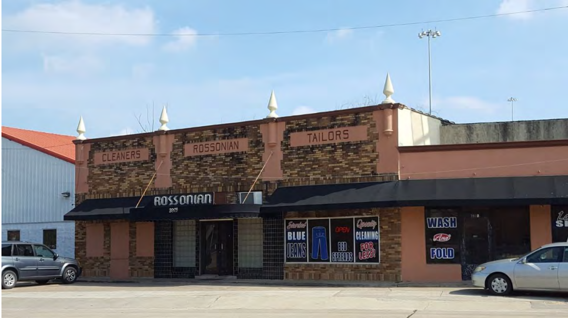
View facing east-northeast, showing 1928 portion of Rossonian Cleaners building.
