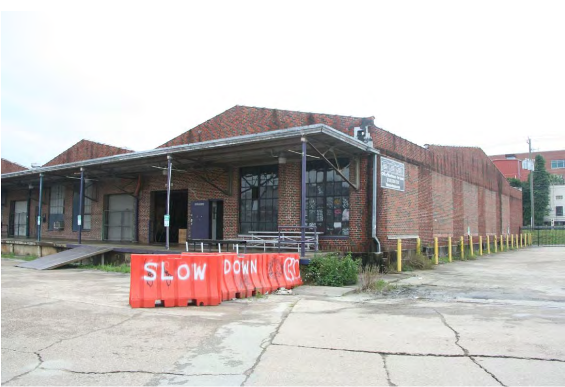
View facing southwest, showing north portion of San Jacinto Warehouses at 1125 Providence Street.
