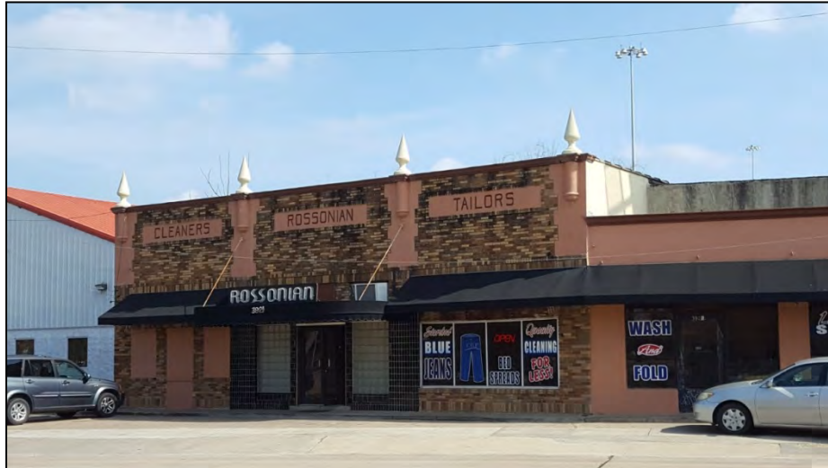
Photo 3-5. Rossonian Cleaners building (1928 portion); View facing east-northeast
