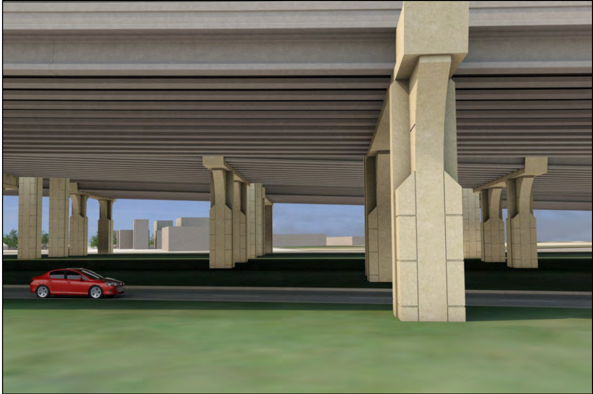
Figure 4-4: Digital rendering of the proposed new elevated roadway of the Proposed Action looking north where Readers Distributors Warehouse currently sits.
