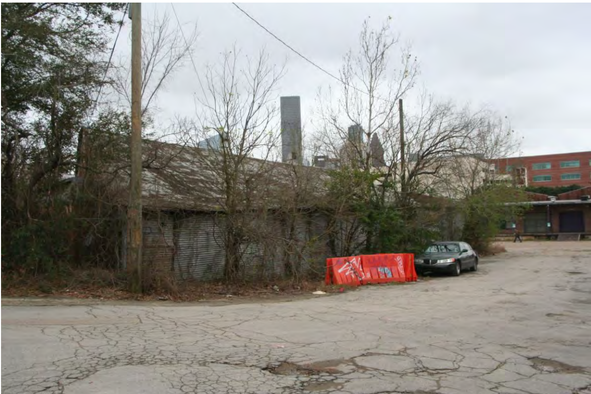
View facing south, showing north side of Carlisle Plastics North Warehouse.
