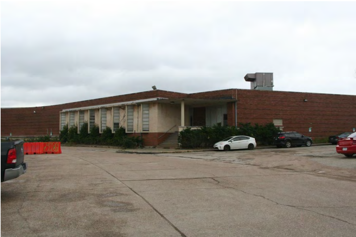
View facing north, showing Readers Warehouse main entry and exterior near office/showroom area.
