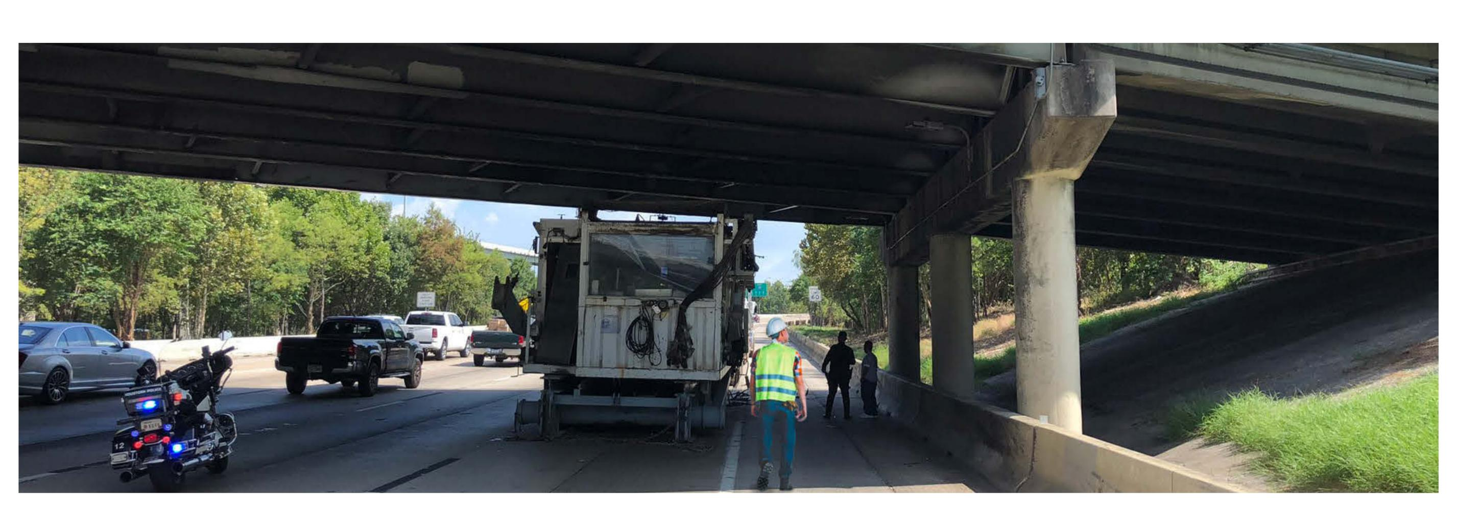
By raising the height under bridges along the interstate and frontage roads to 18.5 feet, we ensure that large freight trucks can pass through without any restrictions. This makes transportation more efficient and safer for everyone.
