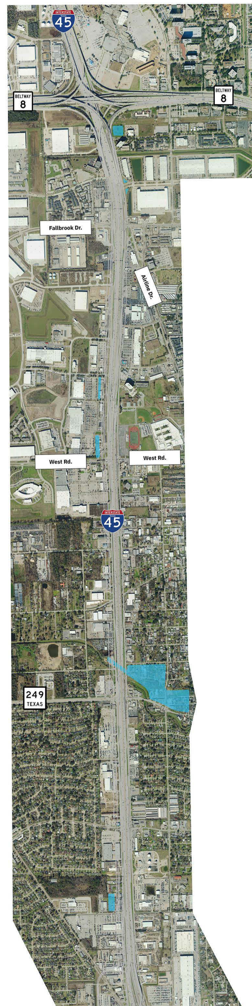
A sample of Segment 1 detention ponds is shown in blue in the graphic above.
