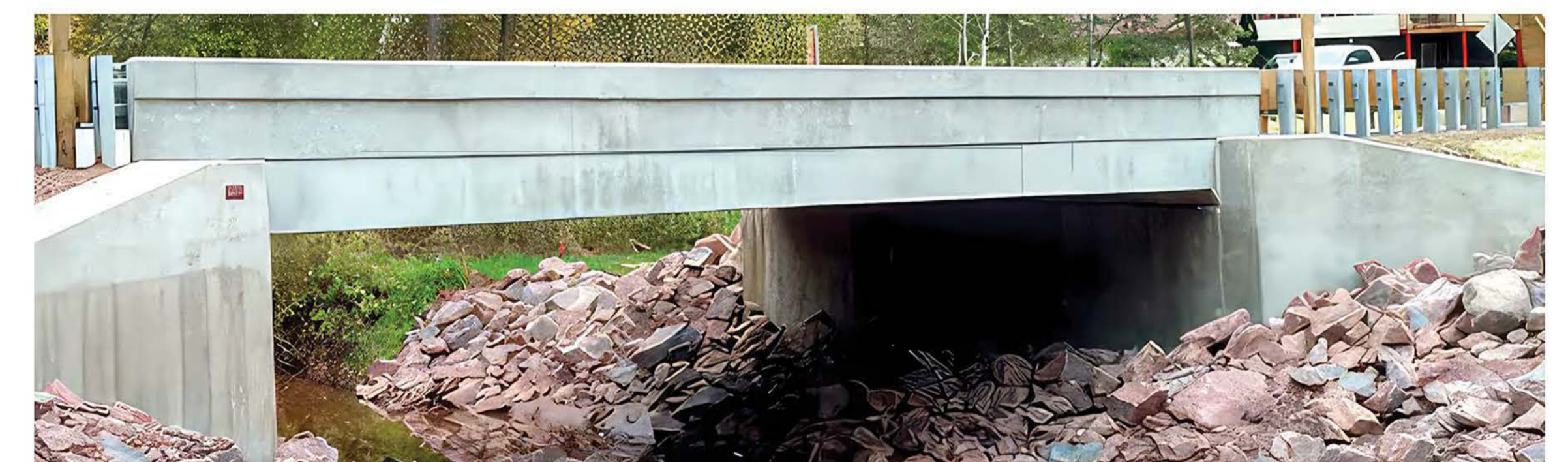
Replacing concrete drain culverts with bridges will allow more stormwater to flow away from the Independence Heights neighborhood near I-45 and I-610.
