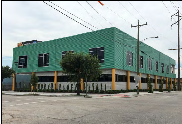
Figure 6-10 SEARCH facility under construction in 2017
