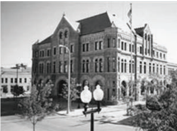
US District Courthouse, Sioux Falls, SD
