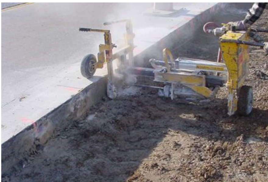
Figure 9-80. Marking and drilling holes at widening joint.
