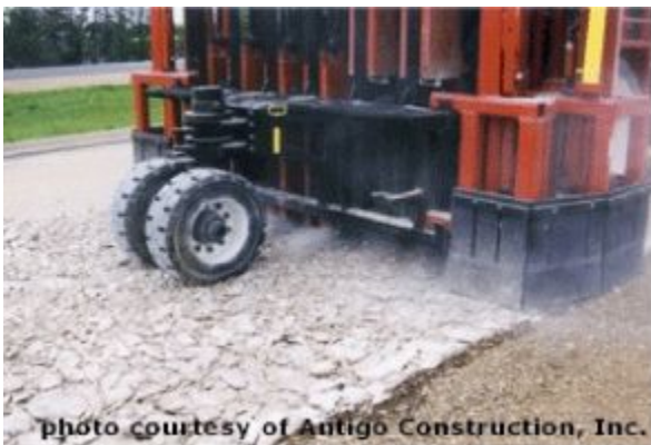
Figure 7-8. Multi-head Pavement Rubblizer. © Copyright 2006 University of Washington
