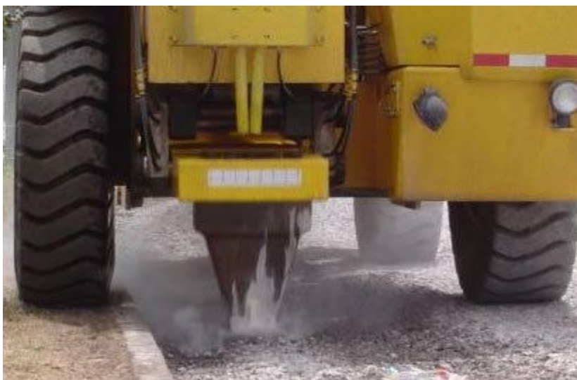
Figure 7-6. Resonant Pavement Breaker. © Copyright 2006 University of Washington
