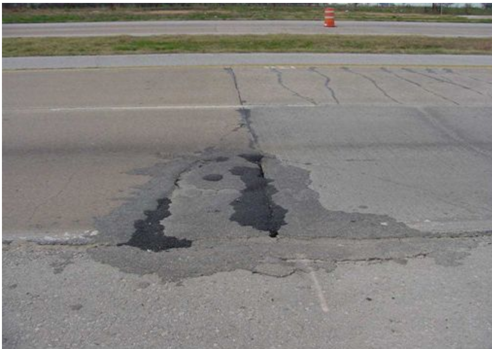
Figure 10-3. Full depth repair of punchouts in CRCP.
