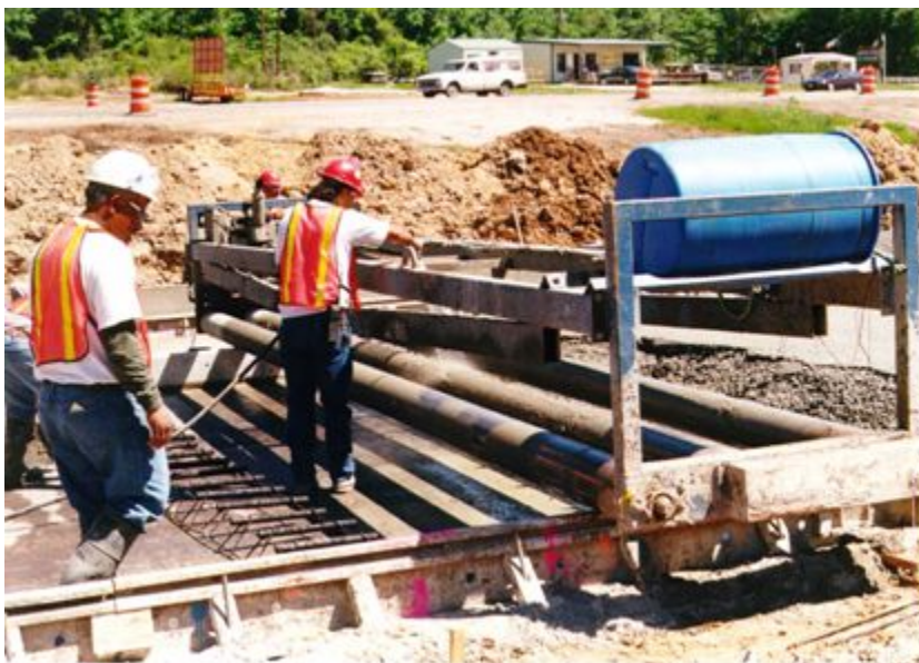
Figure 9-29. Cleaning screed between haul trucks.
