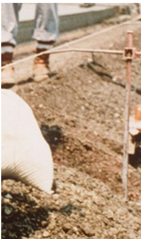
Figure 9-39. Guide wire controls.
