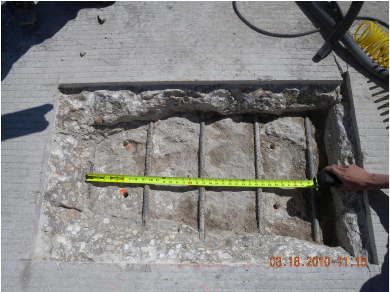
Figure 10-11. Clean repair surfaces.
