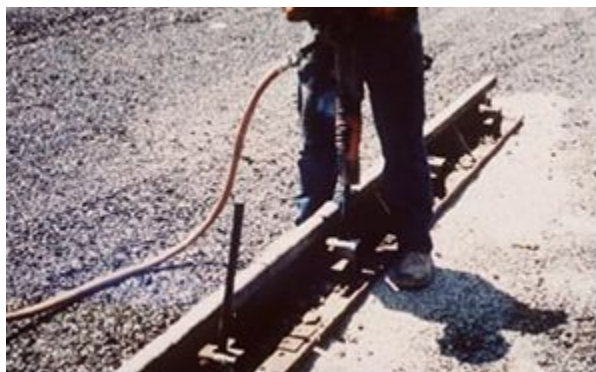
Figure 9-22. Using jackhammer to set staking pin.
