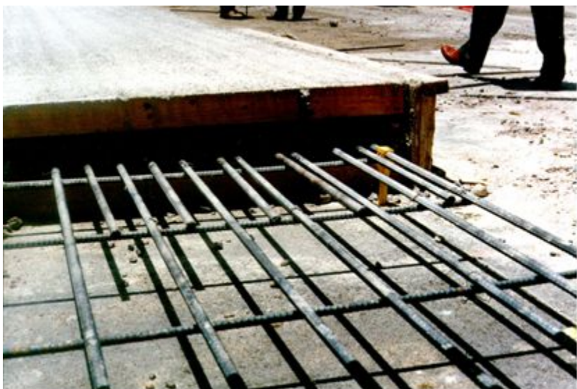
Figure 9-76. Additional steel is required at header.
