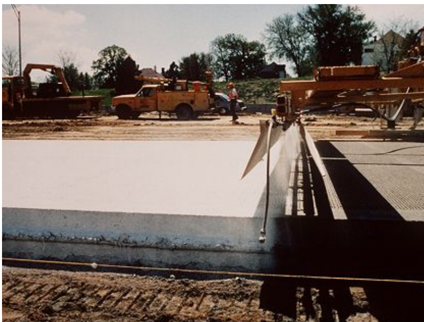
Figure 9-64. Mechanized spraying unit.
