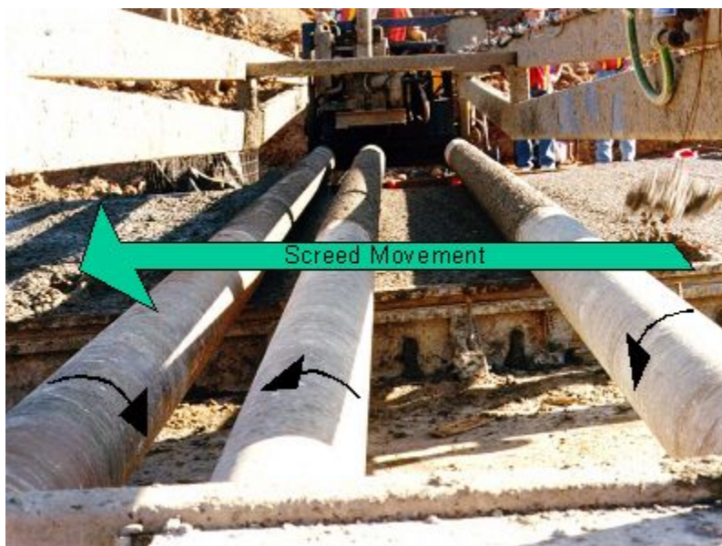
Figure 9-27. A Clary or roller screed.
