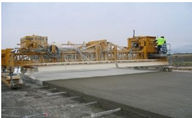
Figure 9-63. Mechanized spraying unit.
