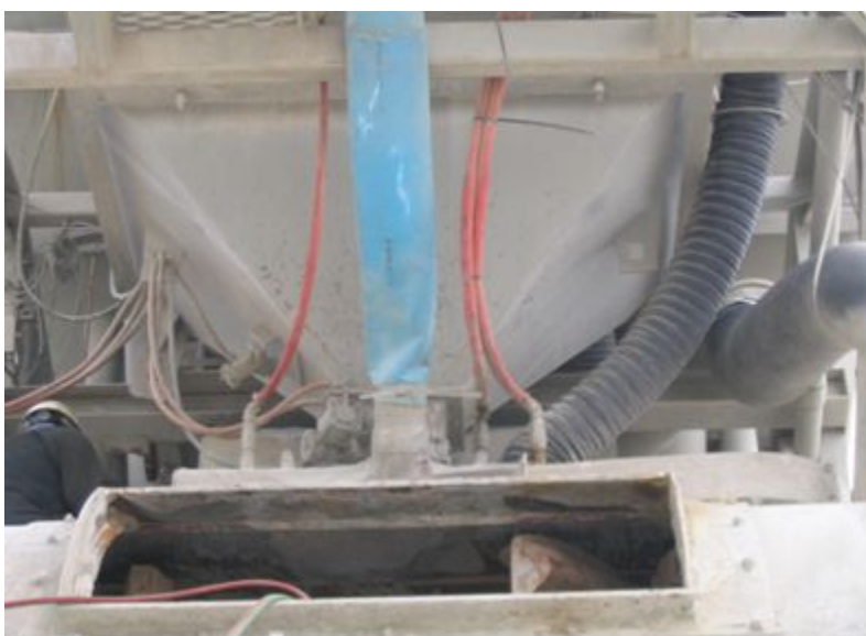
Figure 9-5. Water and admixture supply system.
