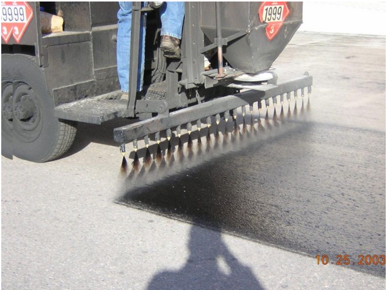
Figure 6-10. Tack coat application showing nozzle coverage area. © Copyright 2006 University of Washington
