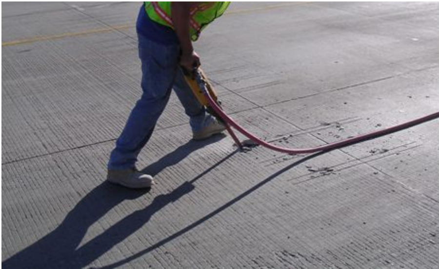
Figure 10-20. Removing concrete fins.
