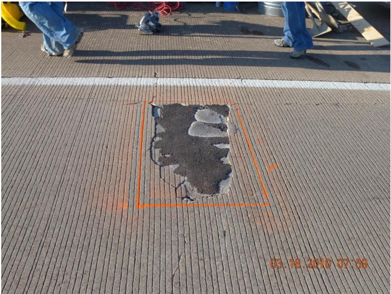
Figure 10-8. Identify the repair limits.
