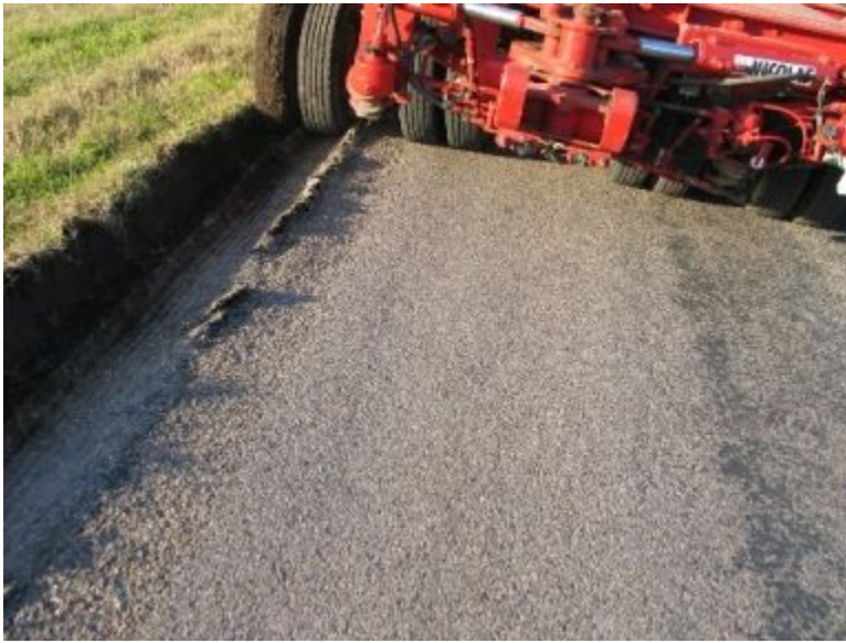
Figure 13-10. Lateral shear failure at the pavement edge (2nd photo).
