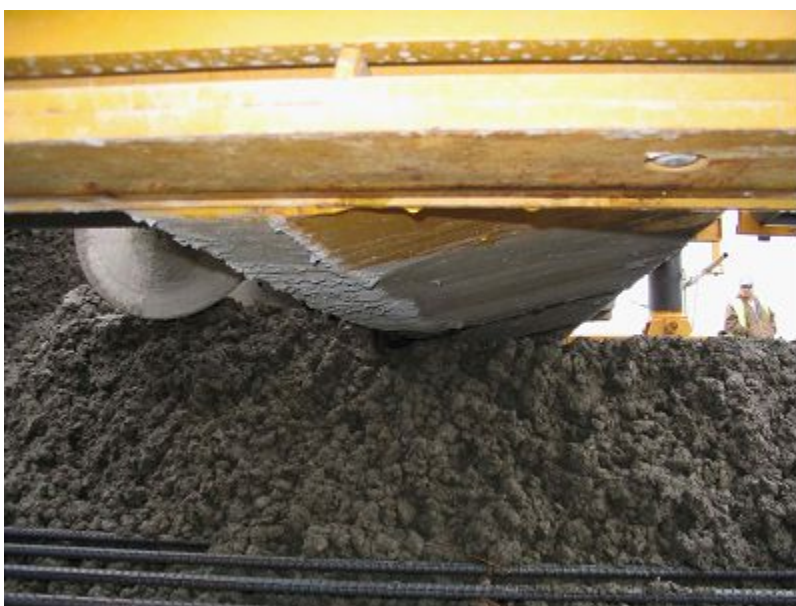
Figure 9-43. Auger and strike-off spreading the concrete.
