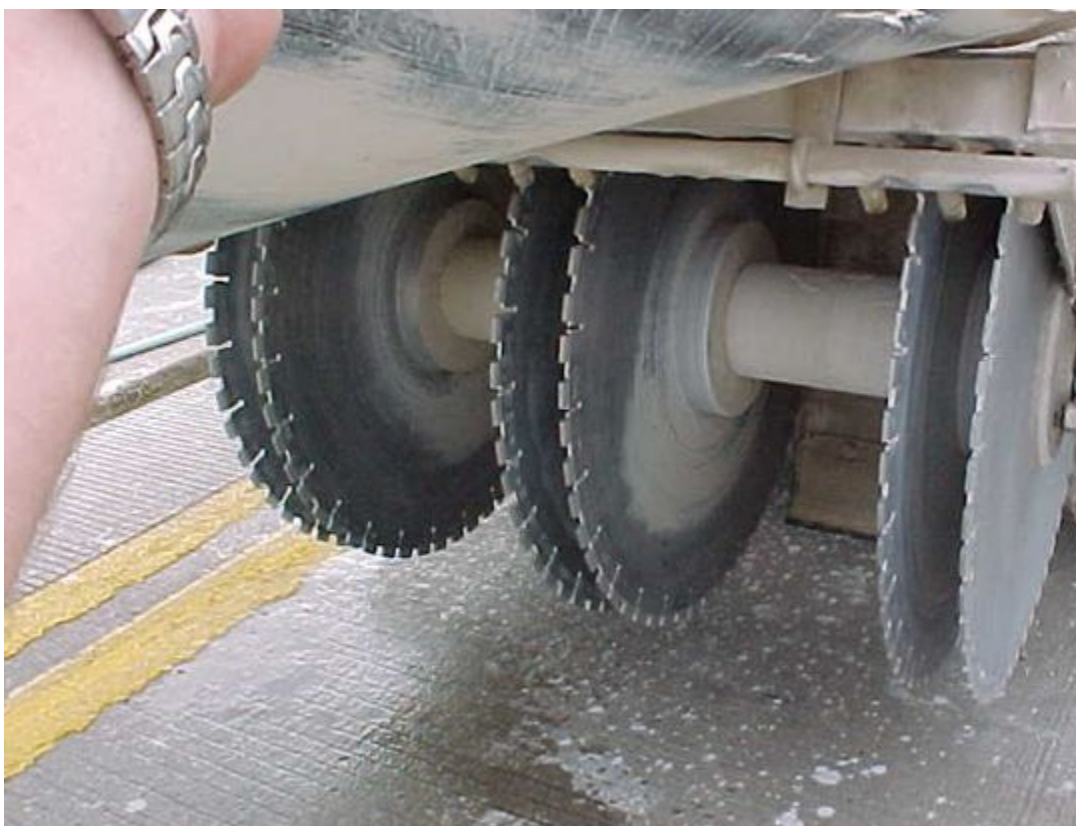
Figure 10-18. Diamond saw slot cutter.
