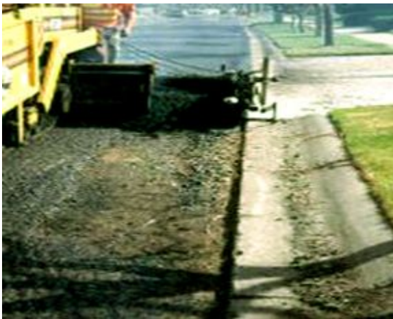
Figure 6-37. Screed Extension. © Copyright 2006 University of Washington
