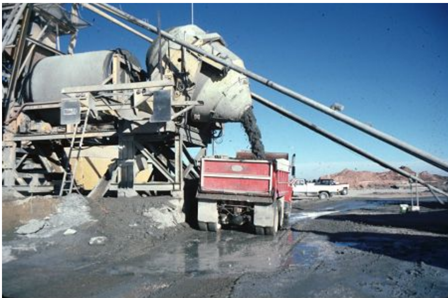
Figure 9-8. Discharging concrete into a dump truck.
