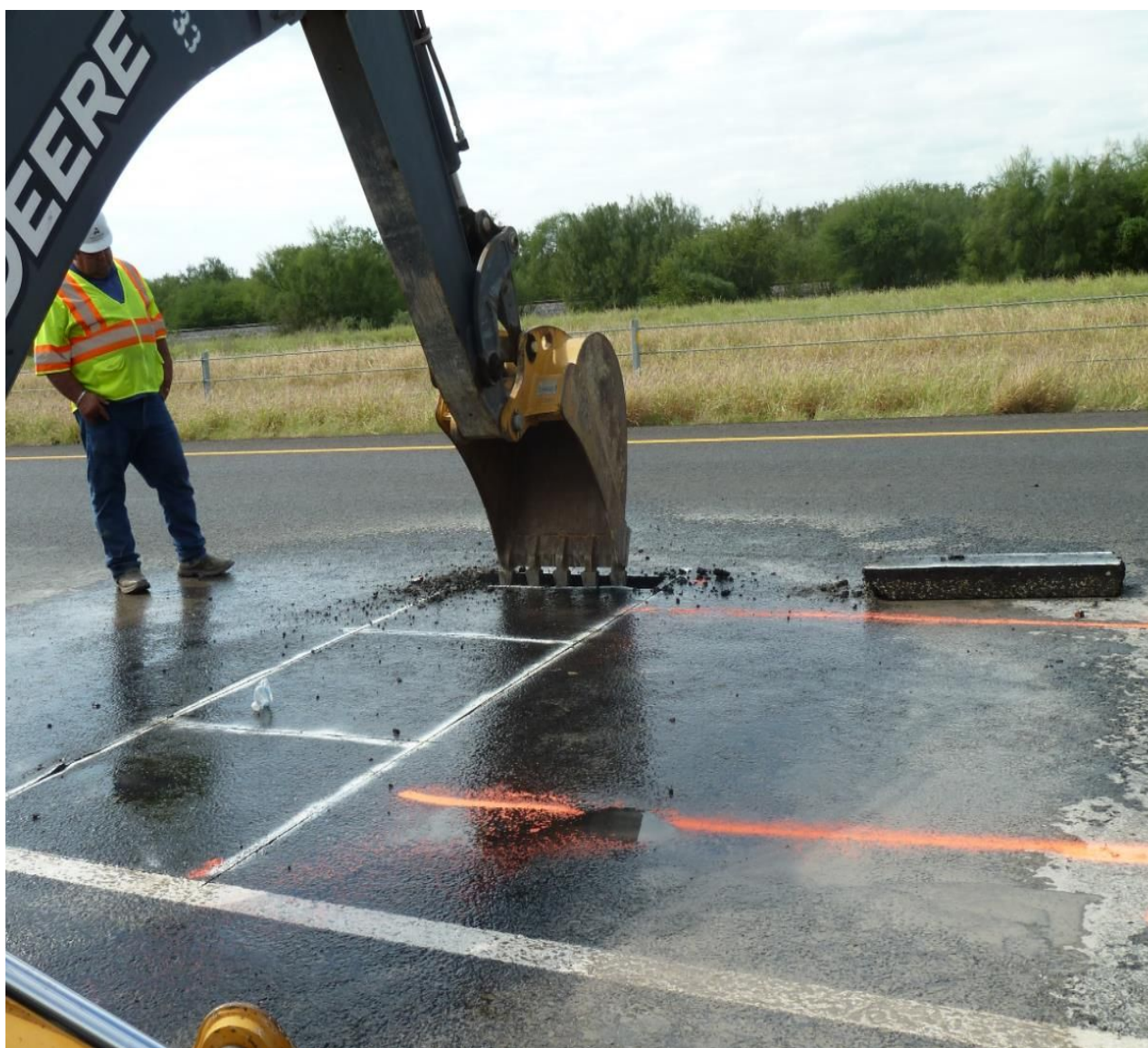
Figure 4-19. Removing hot-mix asphalt (HMA) block with backhoe.
