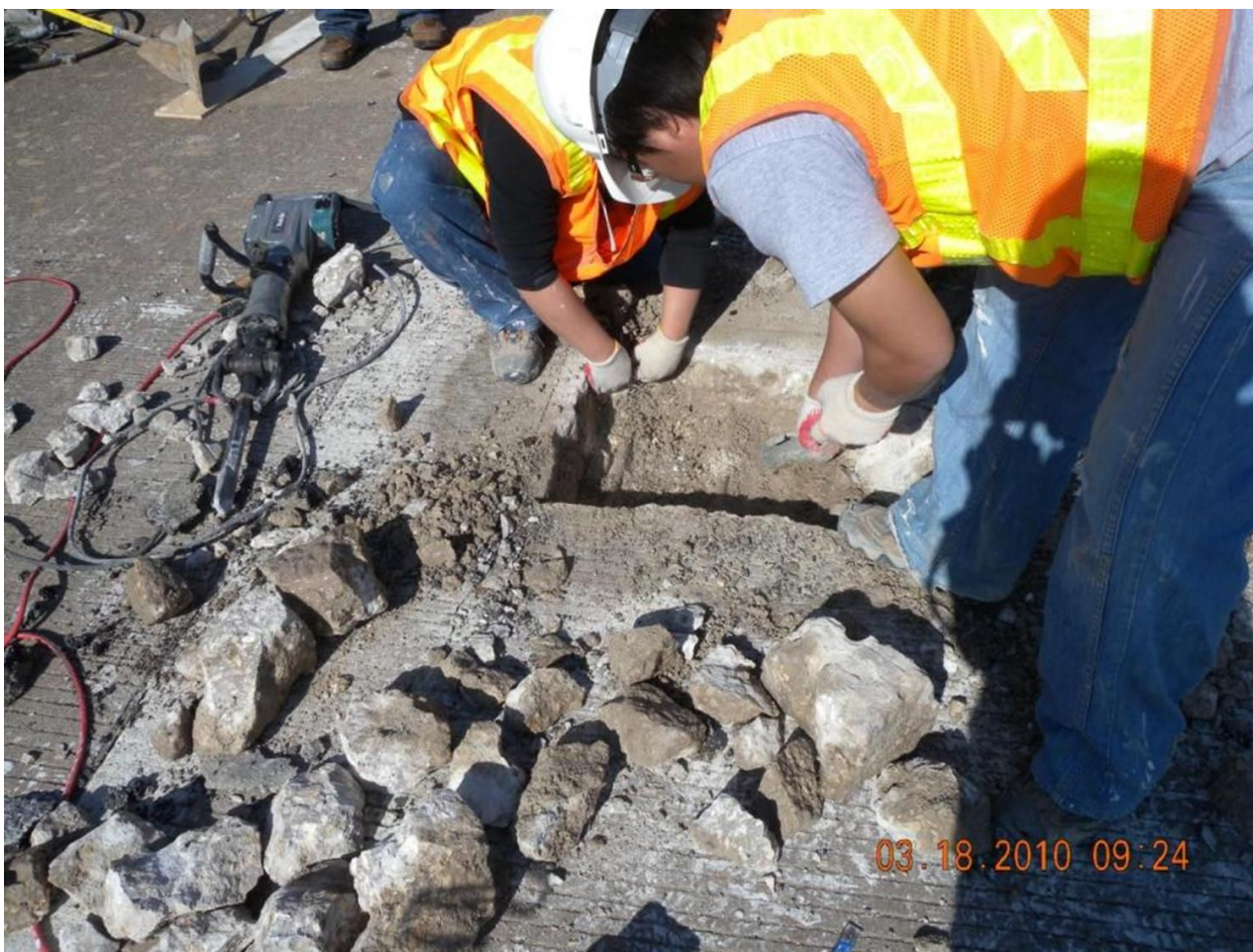
Figure 10-10. Removing deteriorated concrete.
