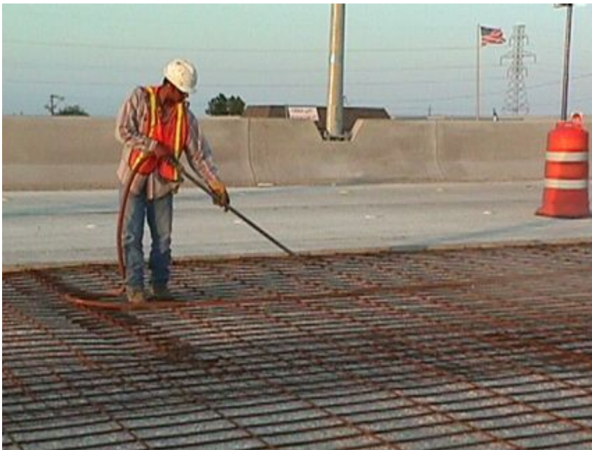
Figure 10-15. Airblasting to clean the concrete surface.
