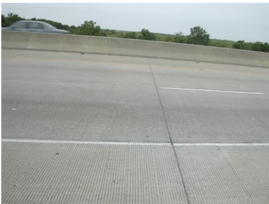
Figure 9-69. Transverse contraction joint.
