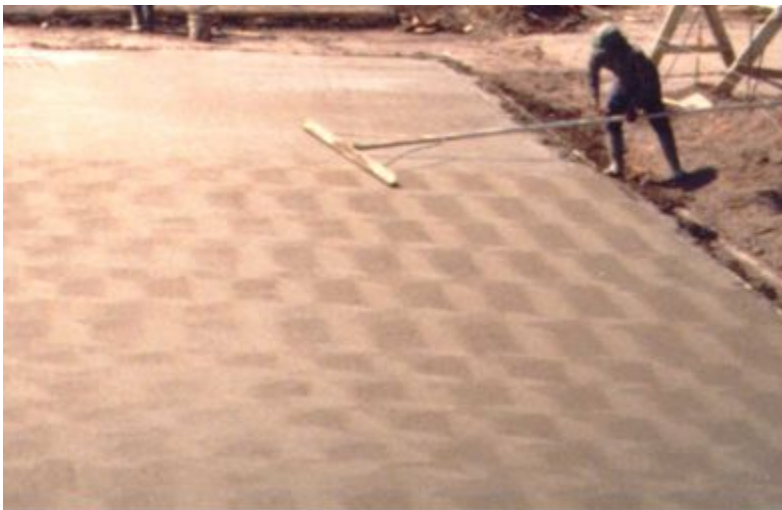
Figure 9-56. Straightedge finishing behind a longitudinal float.
