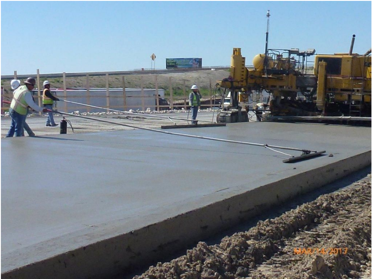
Figure 9-55. Straightedge finishing.
