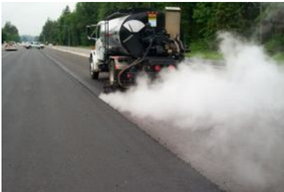
Figure 6-9. Tack coat application. © Copyright 2006 University of Washington
