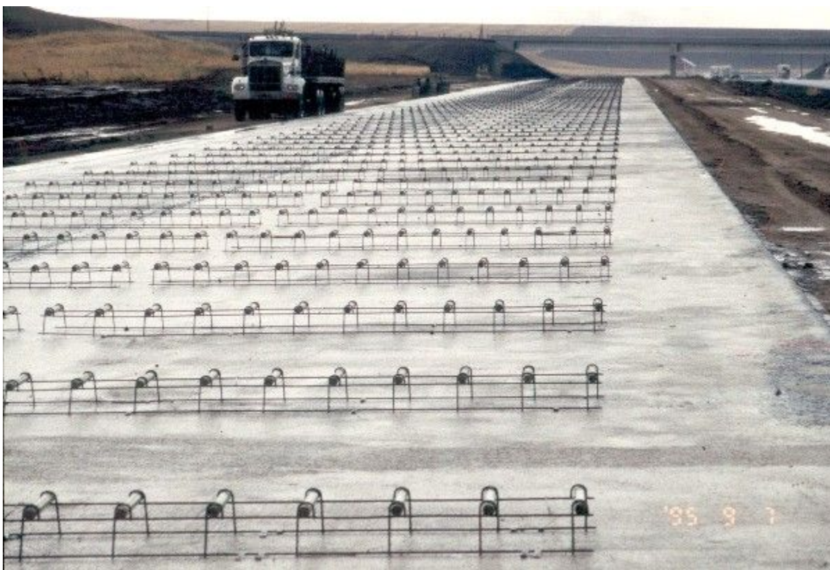
Figure 9-70. Dowel bars.
