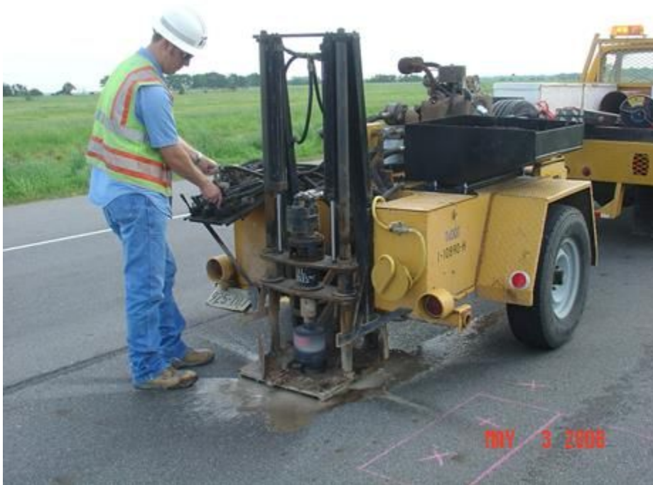
Figure 4-21. Coring using a water-cooled barrel.
