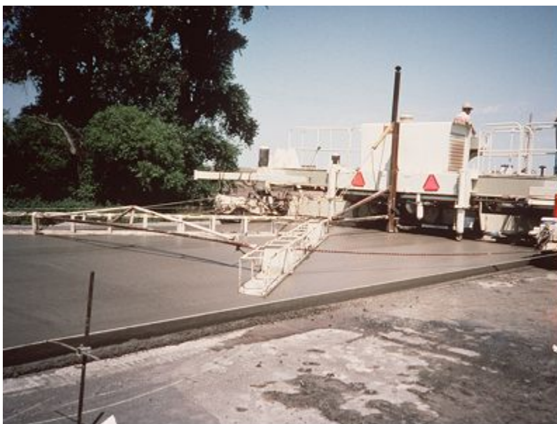
Figure 9-52. "V" shaped drag float pulled by paver.
