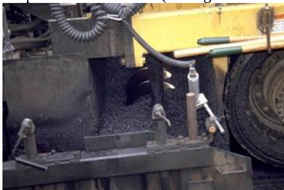
Figure 6-29. Augers distributing HMA. © Copyright 2006 University of Washington
