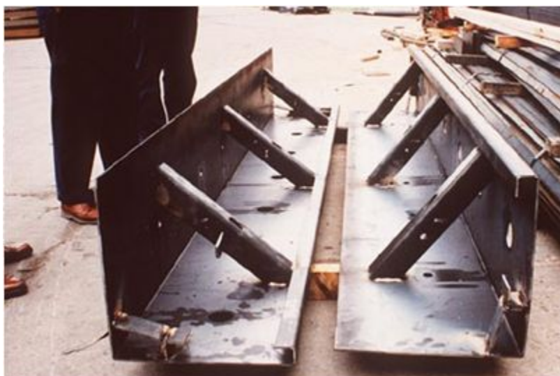
Figure 9-21. Forms ready for setting.
