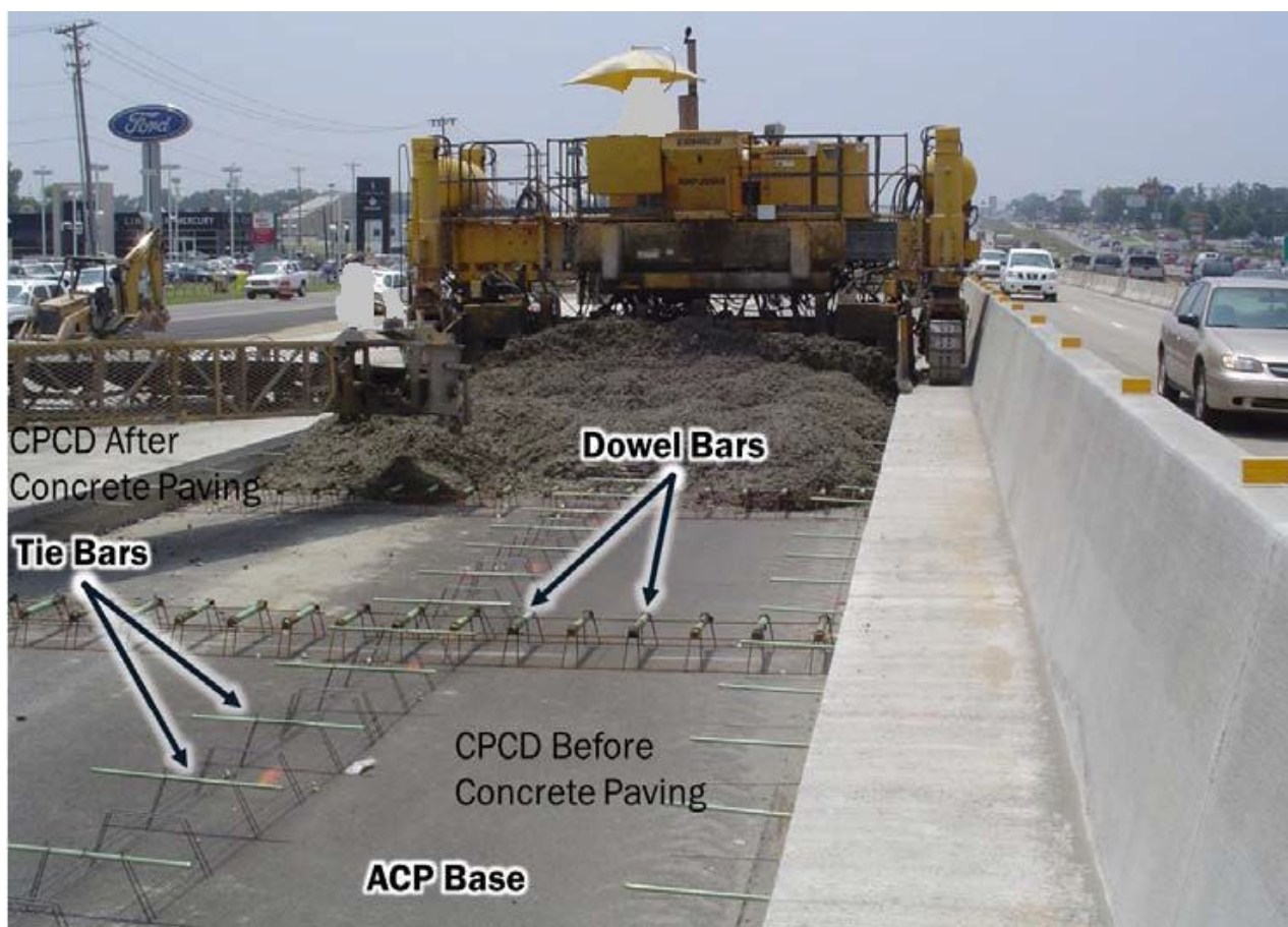
Figure 8-2. Concrete Pavement Contraction Design.
