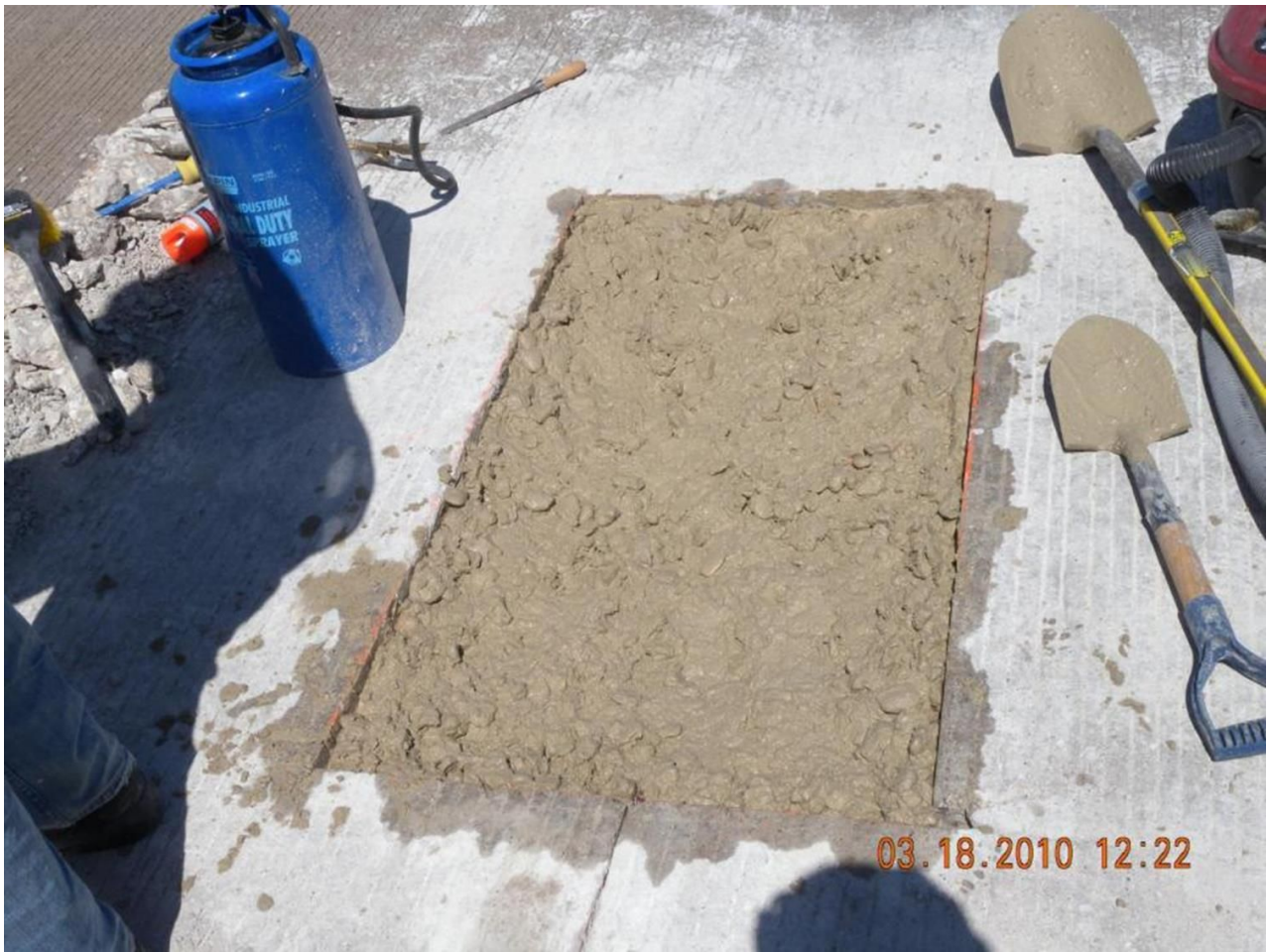
Figure 10-12. Place repair materials.
