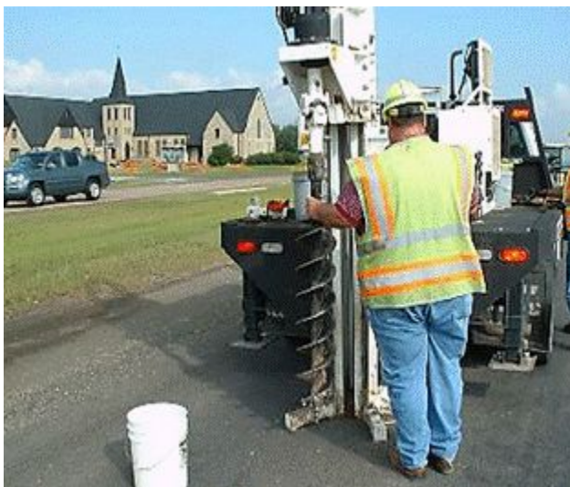
Figure 4-23. Augering a pavement for material samples.
