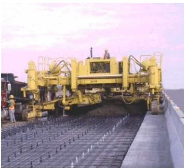
Figure 9-33. Paver machine on tracks.
