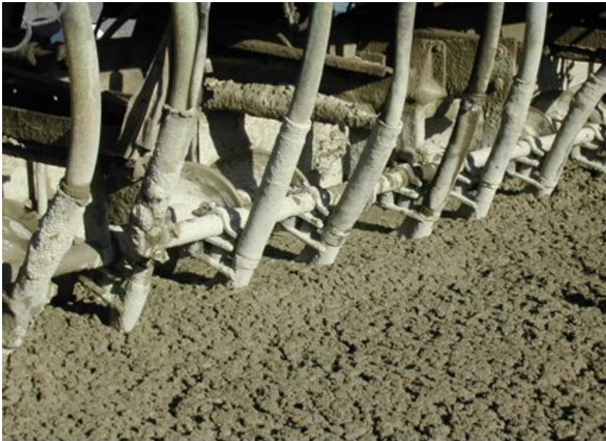
Figure 9-44. Immersion vibrators.
