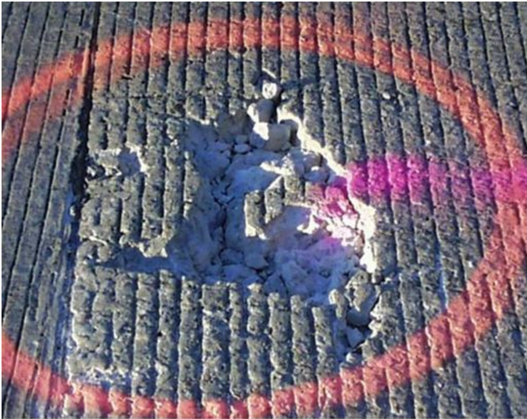
Figure 10-2. Deep spalling.
