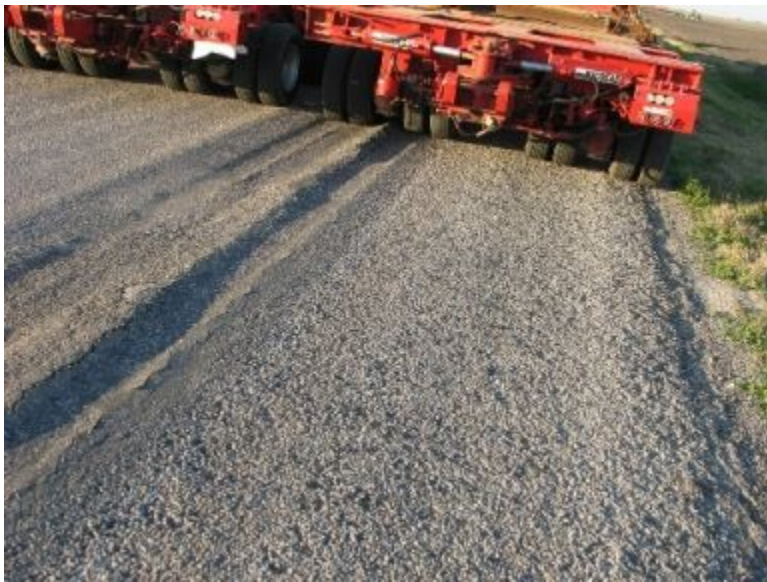
Figure 13-5. Rutting or cracking due to overload of the pavement structure. Recent rainfall or poor drainage conditions resulting in weak or wet subgrade or base materials are often associated with structural damage of this type.
