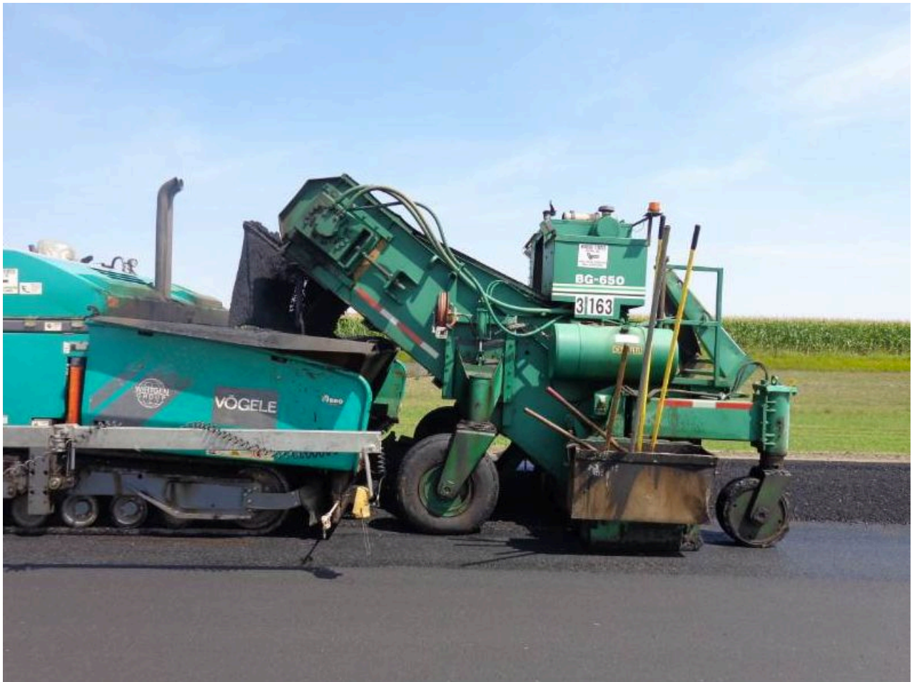
Figure 6-45. Windrow paving. © Copyright 2006 University of Washington
