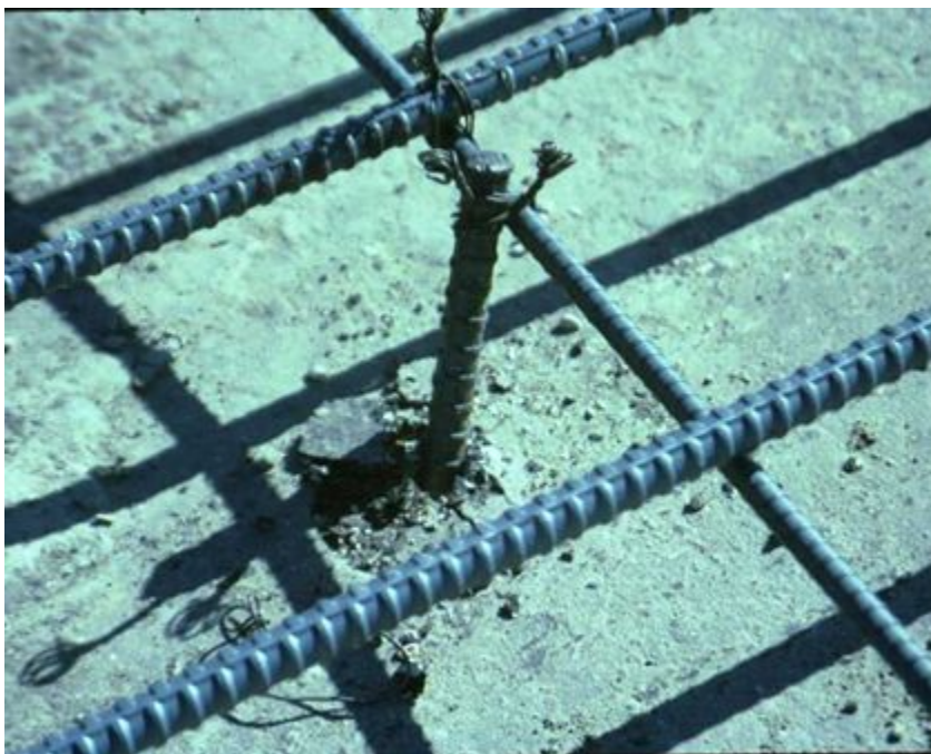
Figure 9-19. Pinning the mat.
