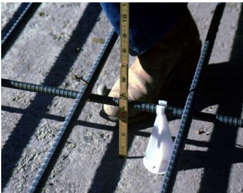
Figure 9-20. Checking steel location.
