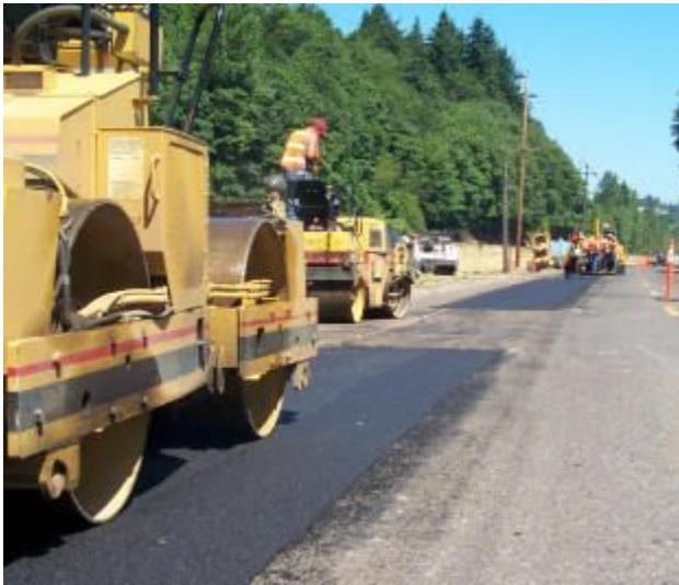
Figure 6-2. Repairing Failed Pavement Sections before Overlay.
