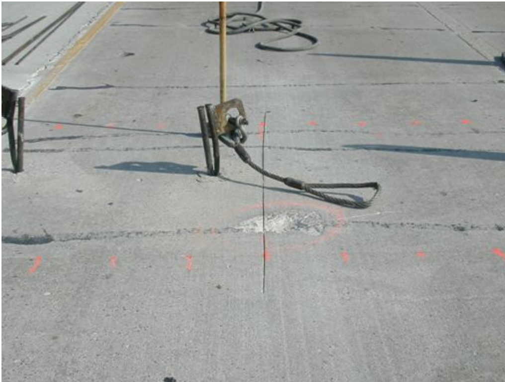
Figure 10-4. Slab ready for lifting.
