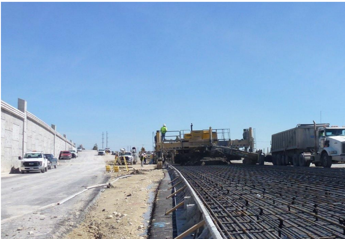
Figure 9-24. Side forms used for paving.
