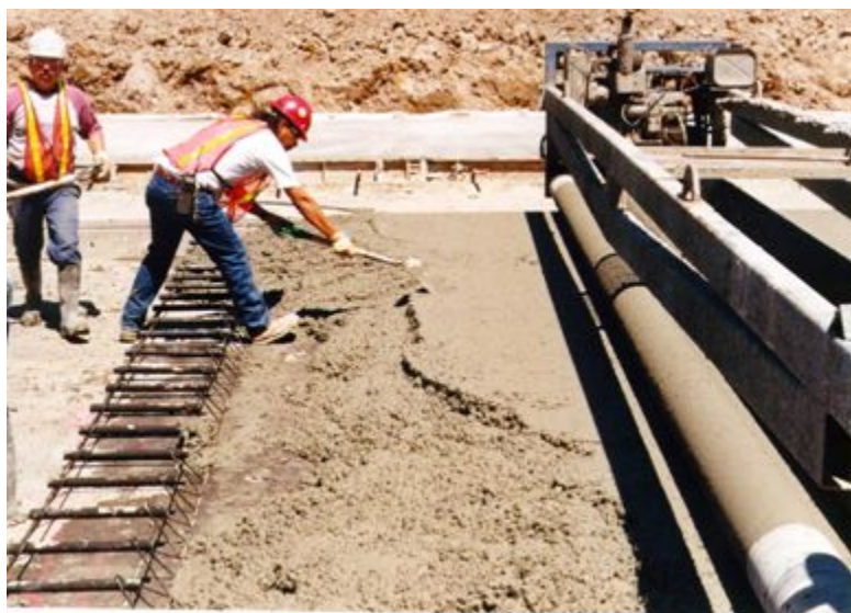
Figure 9-28. Knock down the ridge of mortar formed by the Clary screed.
