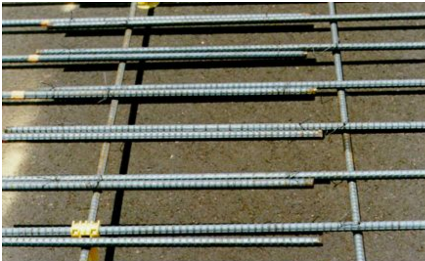
Figure 9-14. Spliced or lapped longitudinal steel.
