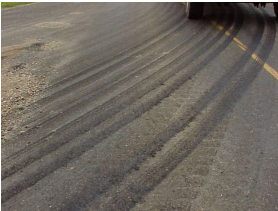
Figure 13-4. Shearing of the pavement surface during turning movements.
