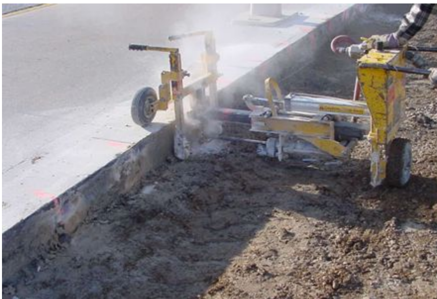
Figure 10-5. Drilling holes at longitudinal joint.
