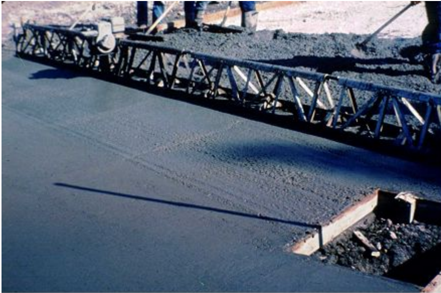
Figure 9-26. Vibrating screed.
