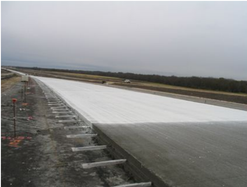
Figure 9-67. Preventing curing compounds from dropping on tie bars.
