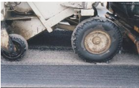
Figure 6-3. Tack coat tracking resulting in no tack coat in the wheel path. © Copyright 2006 University of Washington
