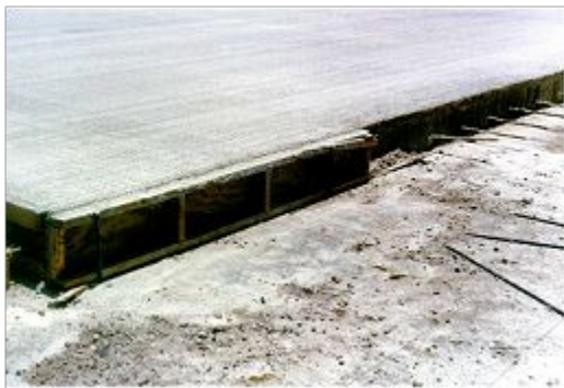
Figure 9-78. Wood side form at a transverse construction joint.
