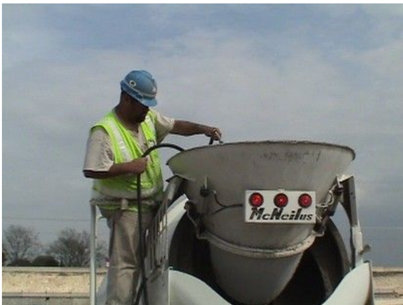
Figure 9-12. Washing the mixer drum.
