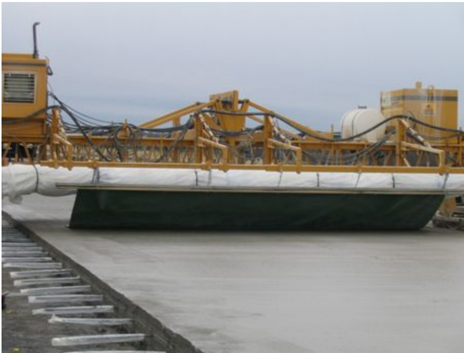
Figure 9-60. Mounting of artificial carpet.
