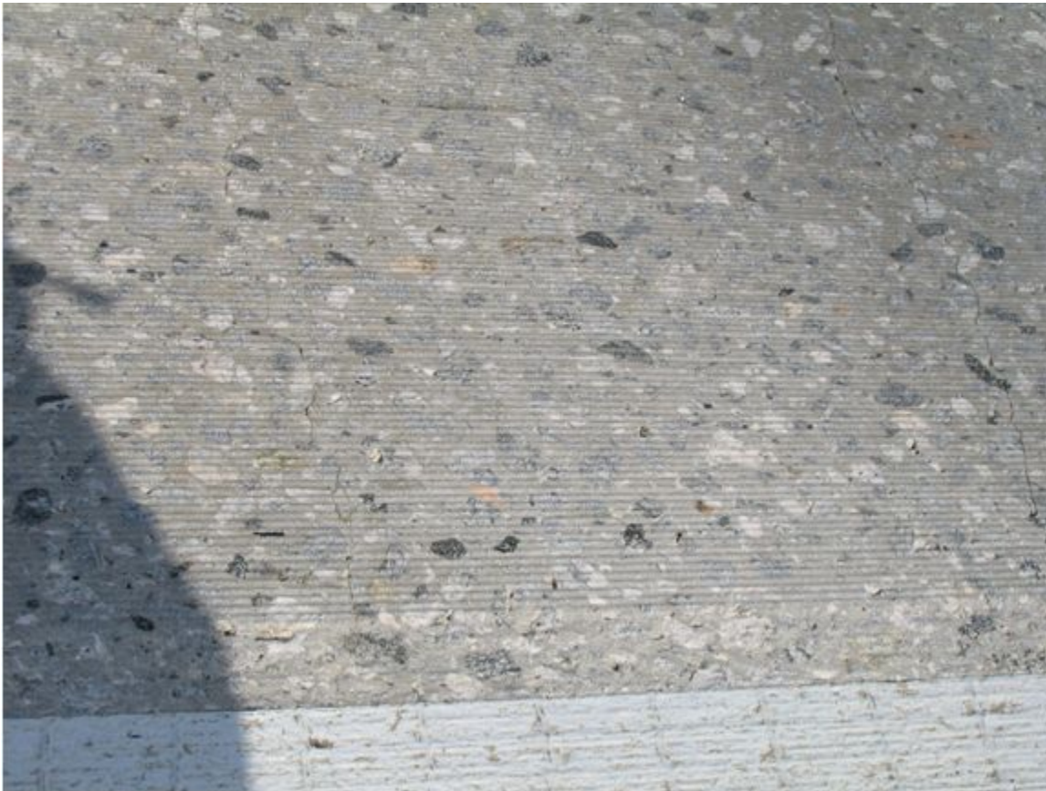
Figure 10-28. Close-up view of diamond ground surface.
