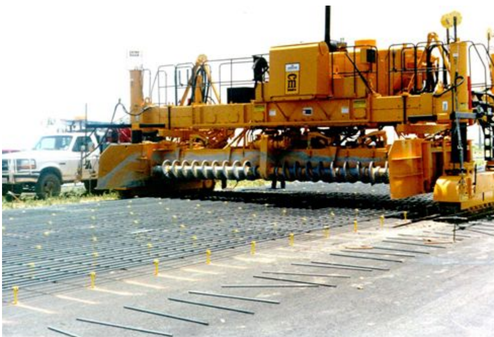
Figure 9-32. Slip-form paver with two augers (idle).
