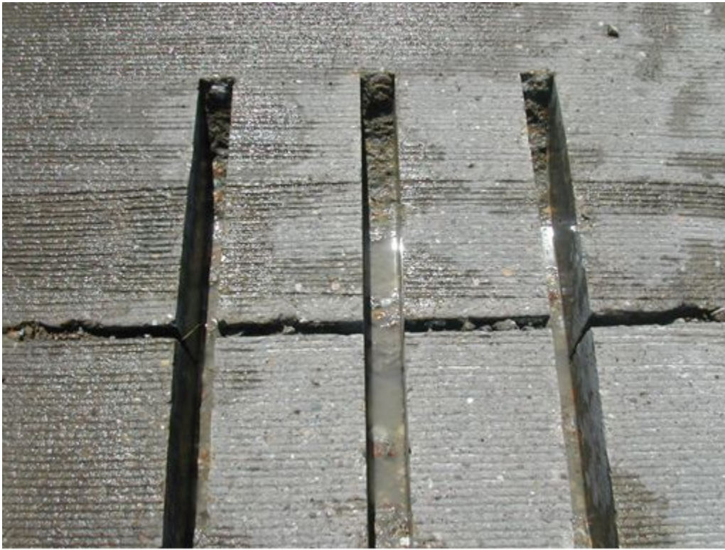
Figure 10-22. Flat bottom after being water cleaned.
