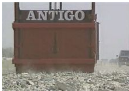
Figure 7-4. Drop hammer breaking slab for break and seat operations. © Copyright 2006 University of Washington
