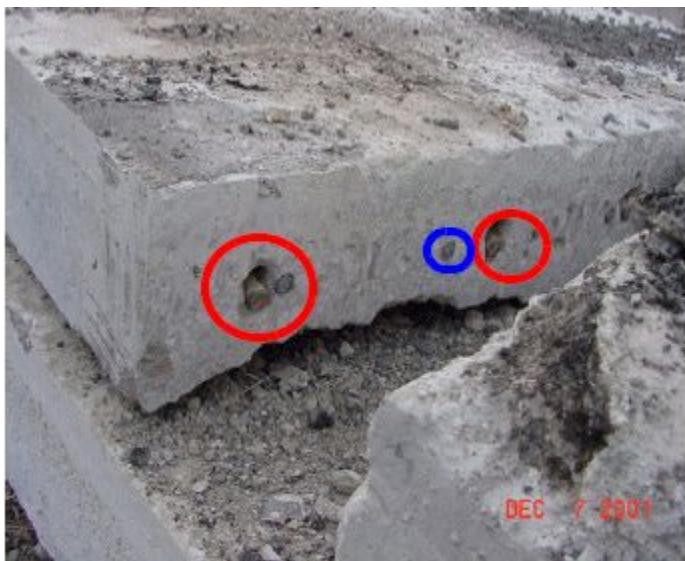
Figure 10-6. Previously repaired slab.
