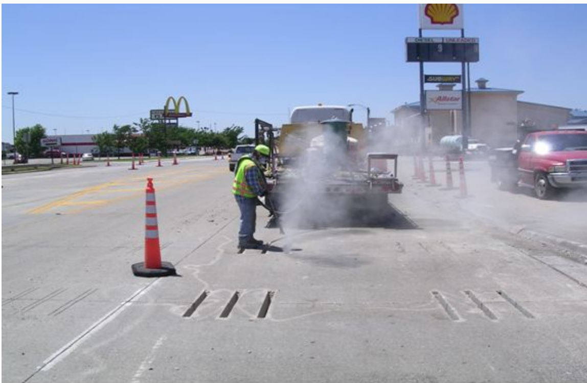
Figure 10-21. Sandblasting the slots.
