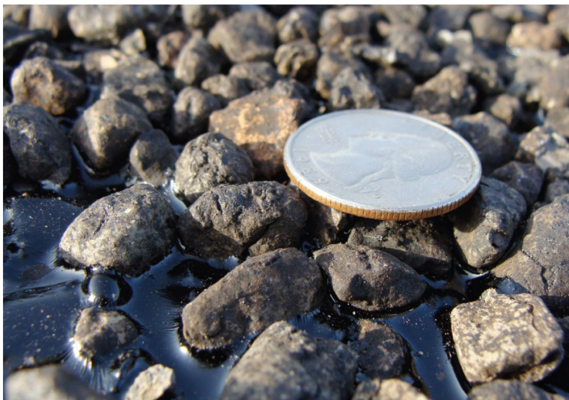
Figure 4-12. Wheel Path Aggregate Embedment Close-Up.
