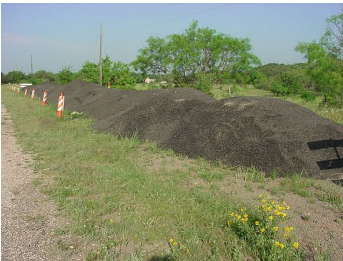
Figure 6-1. Properly Placed Aggregate Stockpiles.
