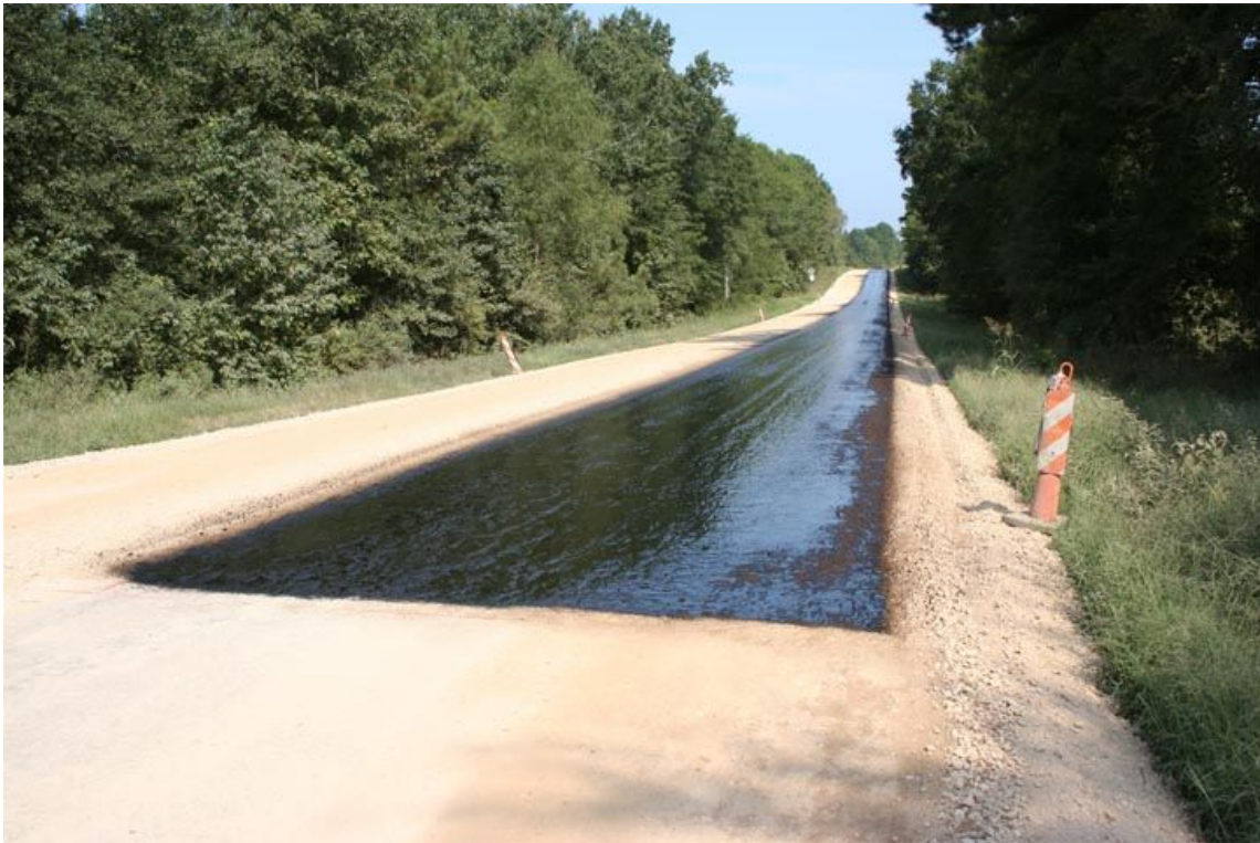
Figure 1-5. Spray-applied prime (MC-30 or AEP).
