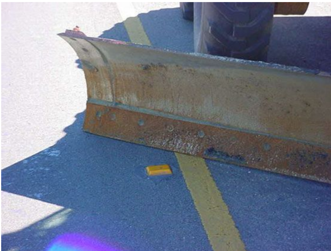
Figure 8-2. Removal of Raised Pavement Markers.
