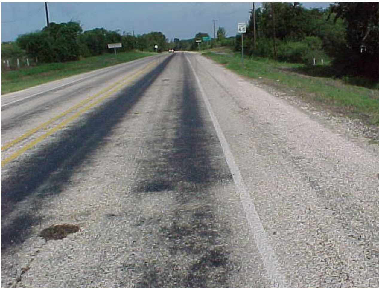
Figure 1-3. A seal coat pavement surface exhibiting flushing in the wheelpaths.
