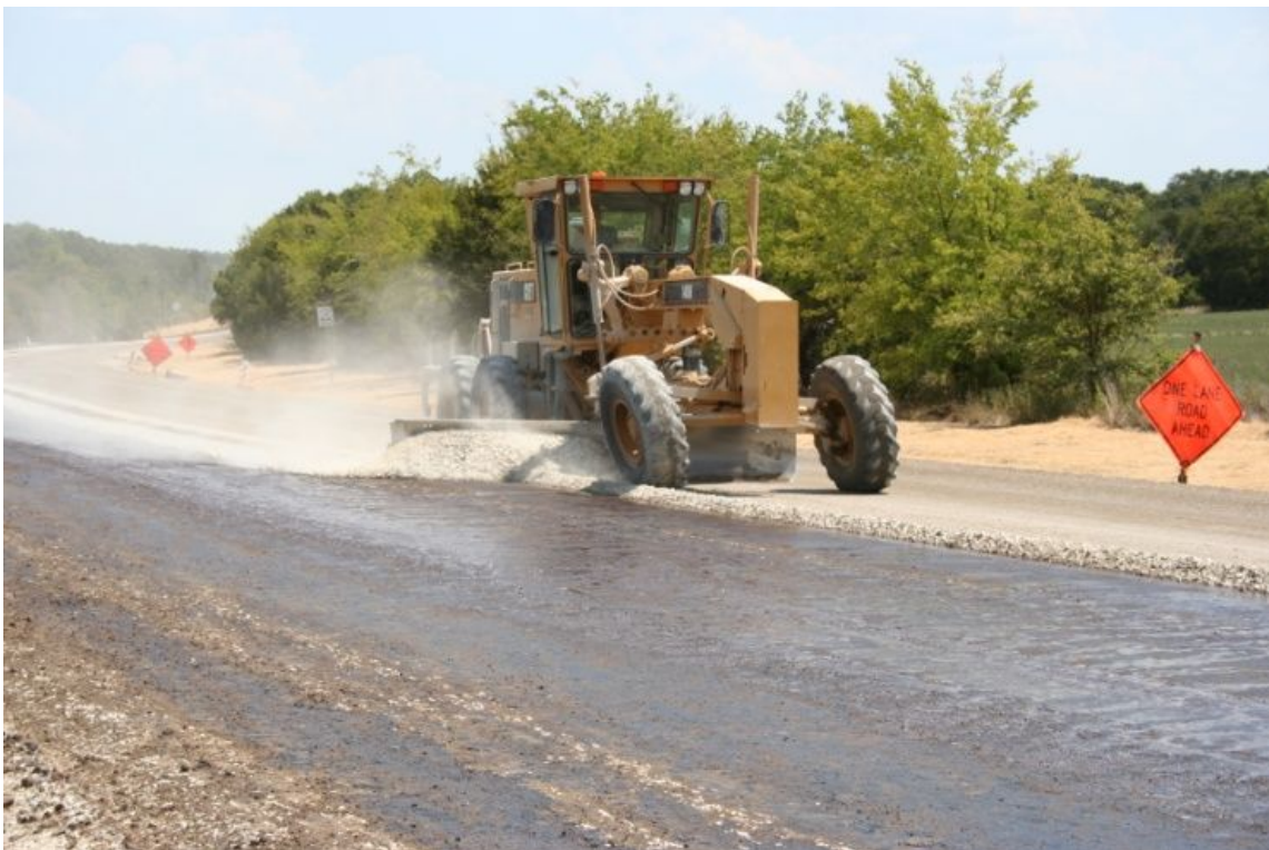
Figure 1-6. Worked-in (cut-in) prime.
