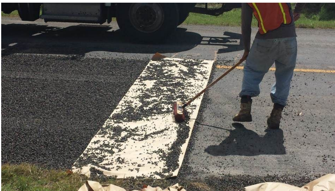
Figure 8-4. Paper Joint in Place at Beginning of Second Shot.
