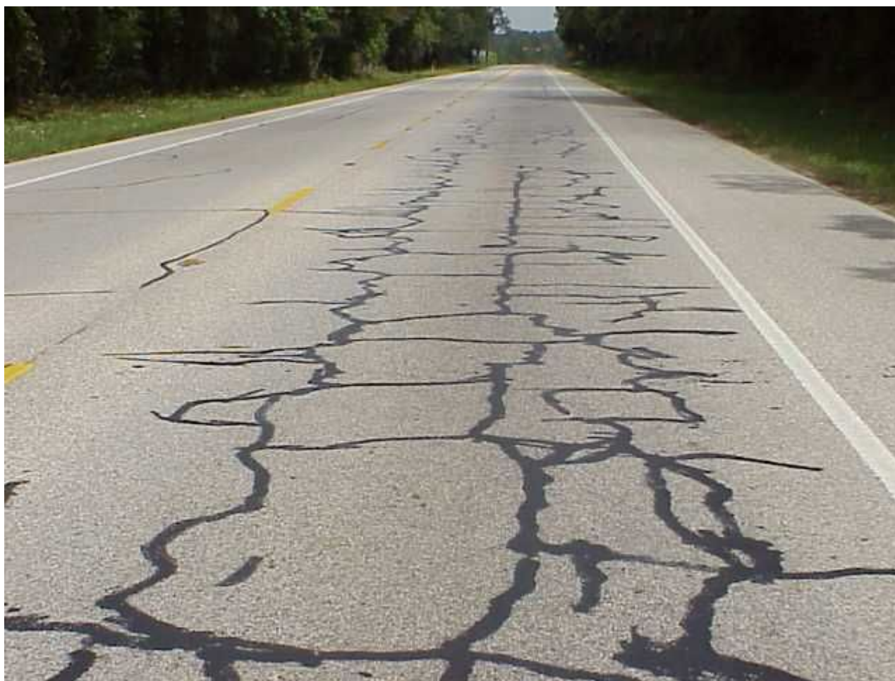
Figure 2-2. Good candidates for seal coat.
