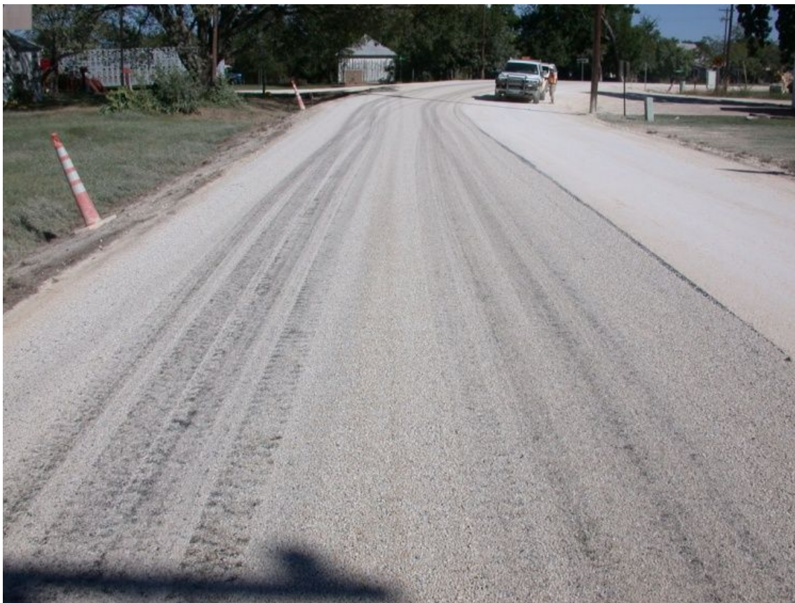
Figure 1-7. Covered (inverted) prime.◆
