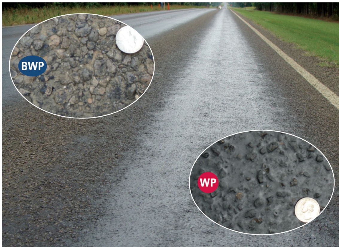
Figure 4-3. Lane with severe flushing. ♦
