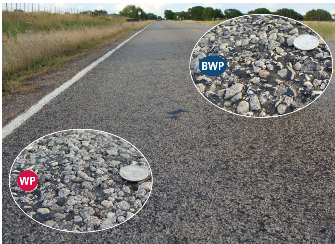
Figure 4-7. Lane with mild flushing.
