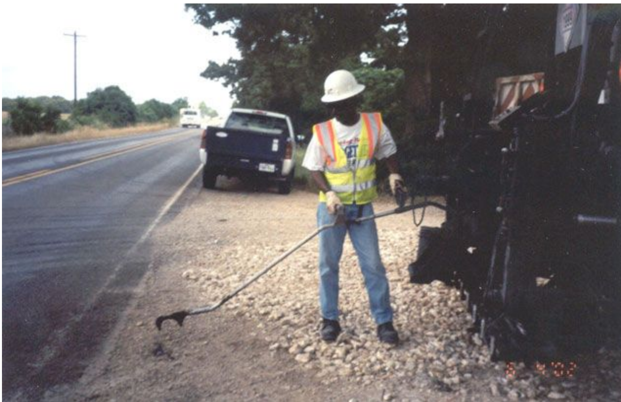
Figure 7-22. Typical Hand Sprayer on Asphalt Distributor.
