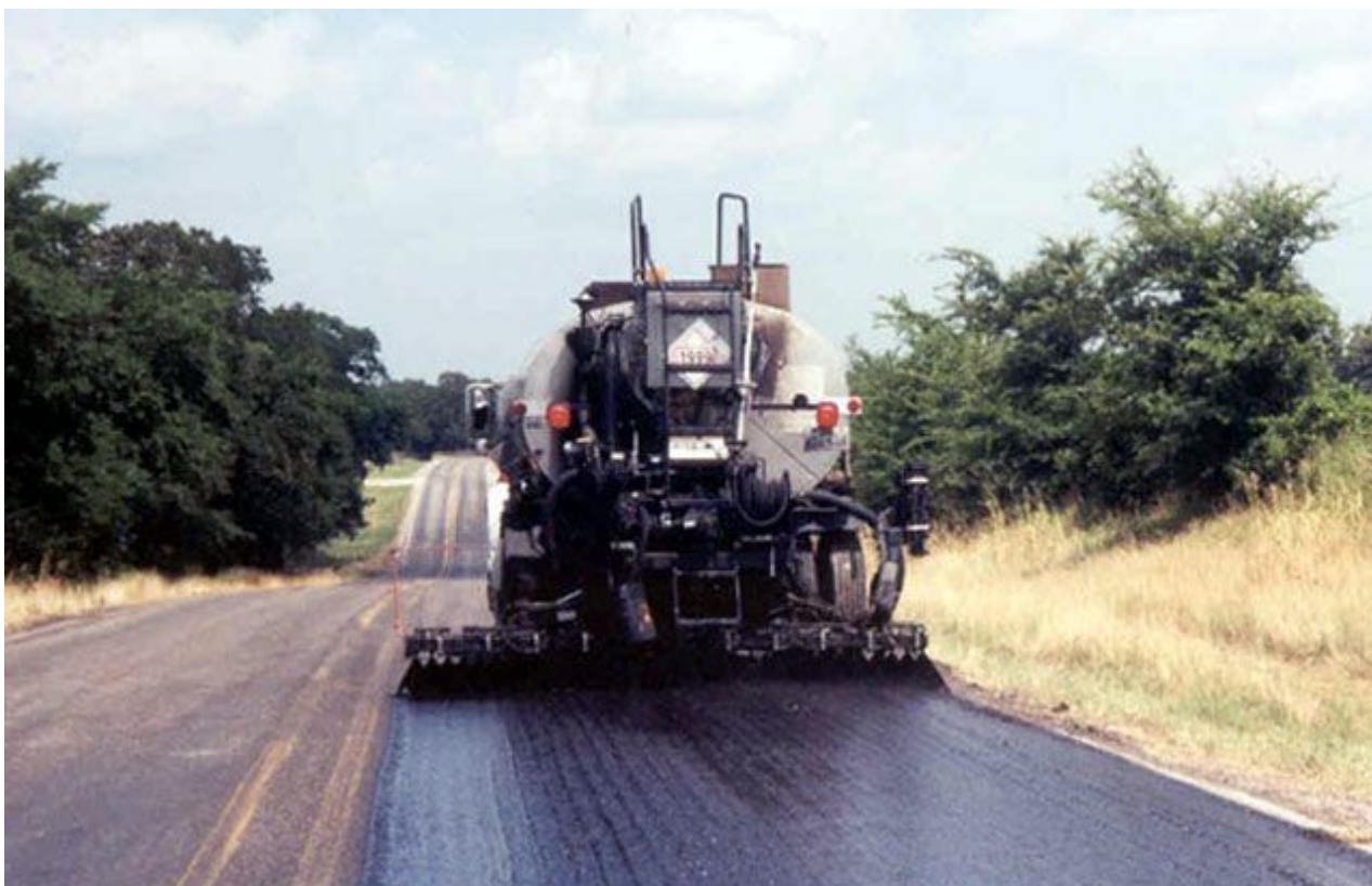
Figure 7-3. Typical Asphalt Distributor.
