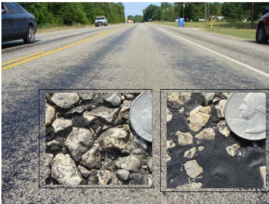
Figure 4-2. Pavement texture varying across a pavement.
