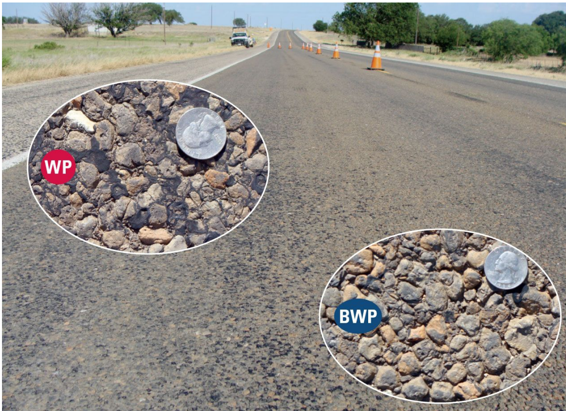
Figure 4-6. Lane with mild to moderate flushing.
