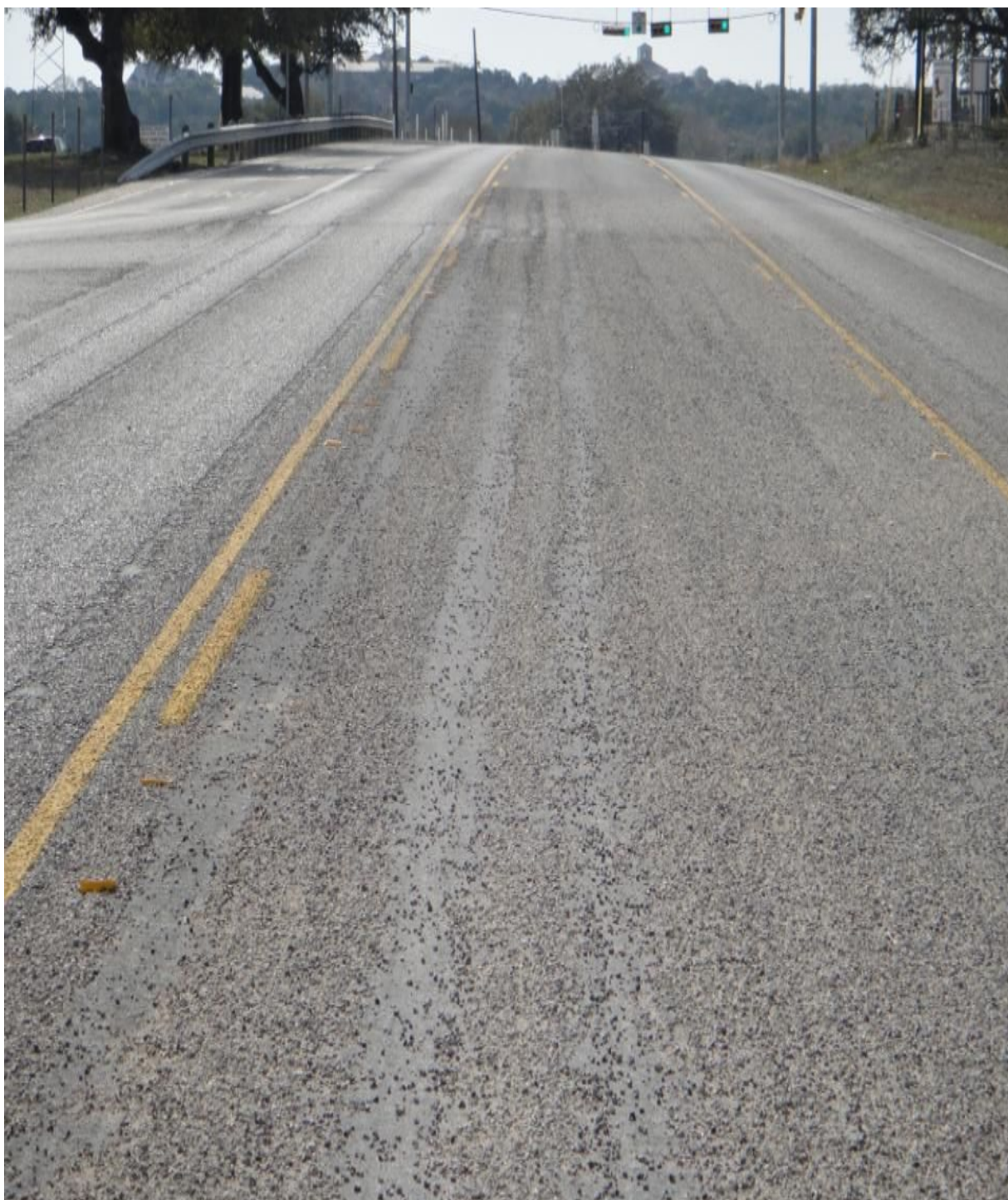
Figure 1-2. Seal coat pavement surface exhibiting aggregate loss.
