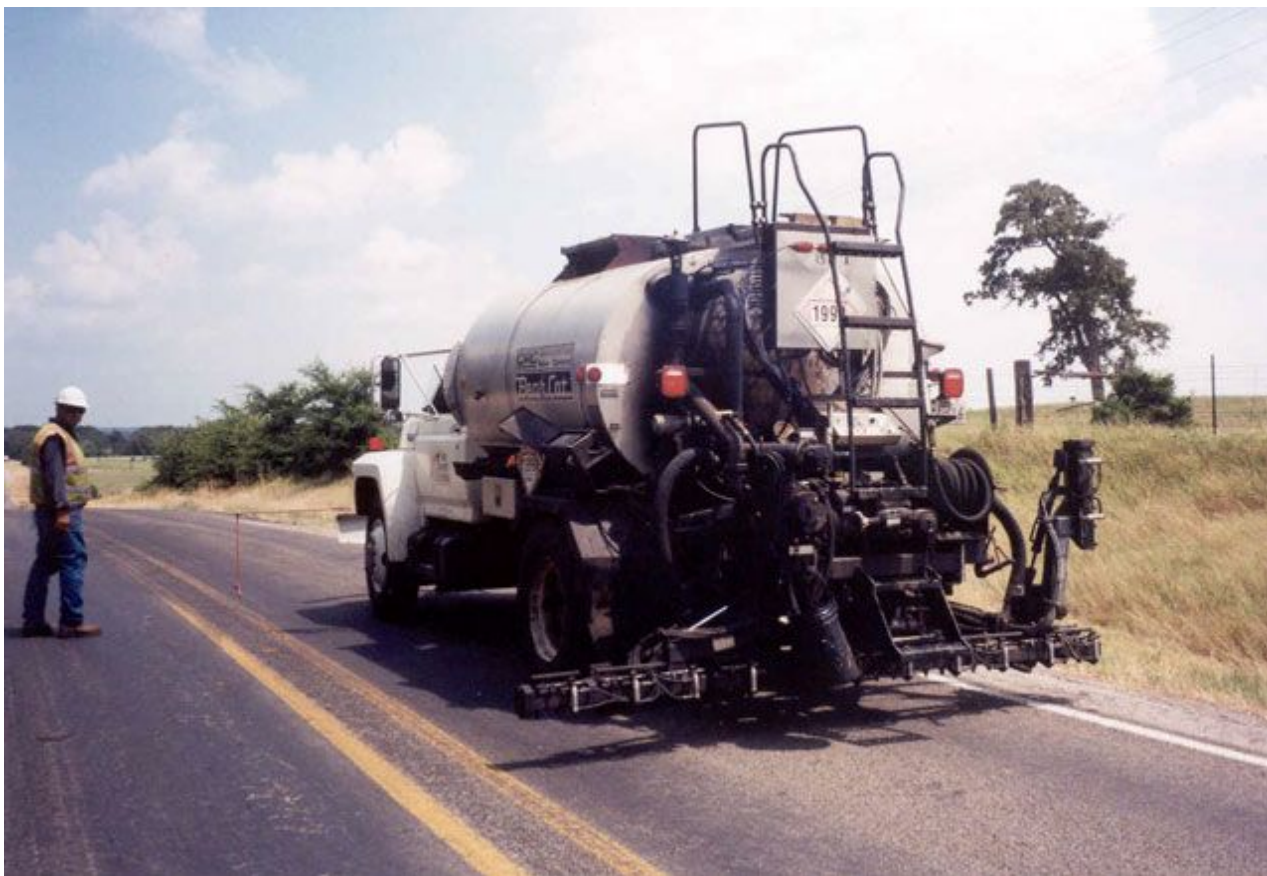
Figure 7-11. Typical Distributor Spray Bar.
