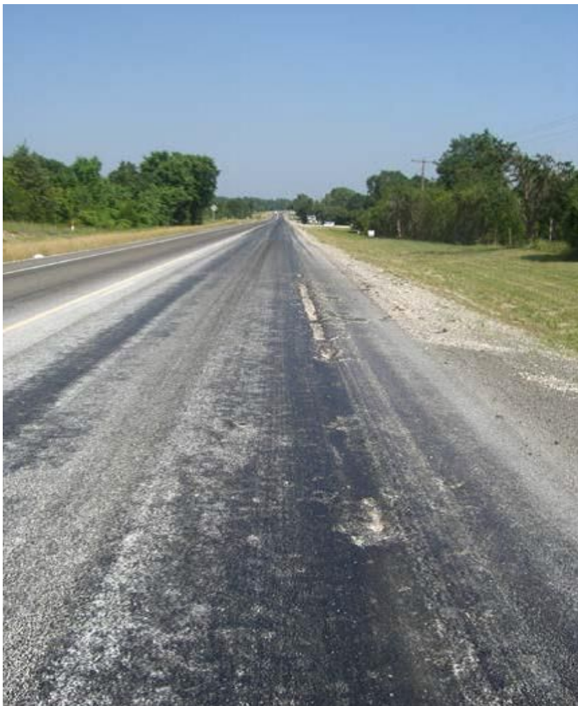
Figure 1-4. Potholes forming due to poorly bonded surface treatment.
