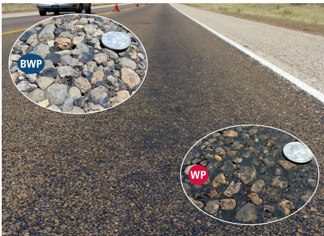
Figure 4-5. Lane with moderate flushing.
