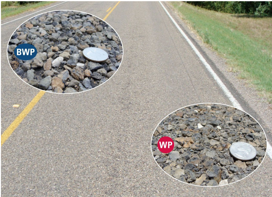
Figure 4-8. Lane with slight wheel path color difference.
