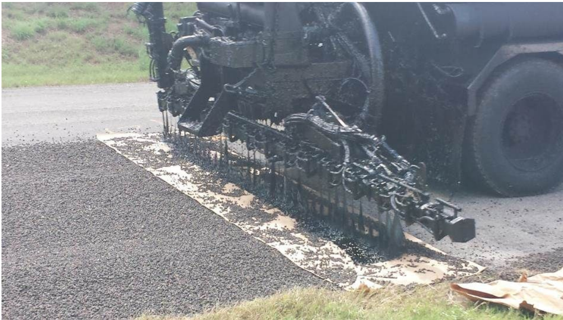
Figure 8-6. Correct Starting Position over Paper Joint.
