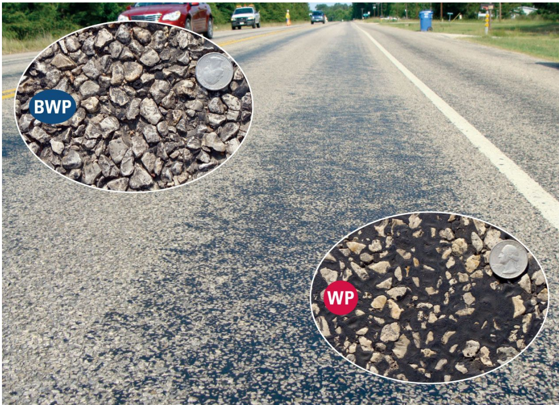
Figure 4-4. Lane with moderate to severe flushing.❖
