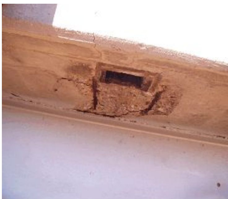
Figure 5-1. Corrosion damage due to concentrated de-icing solution at drain site.
