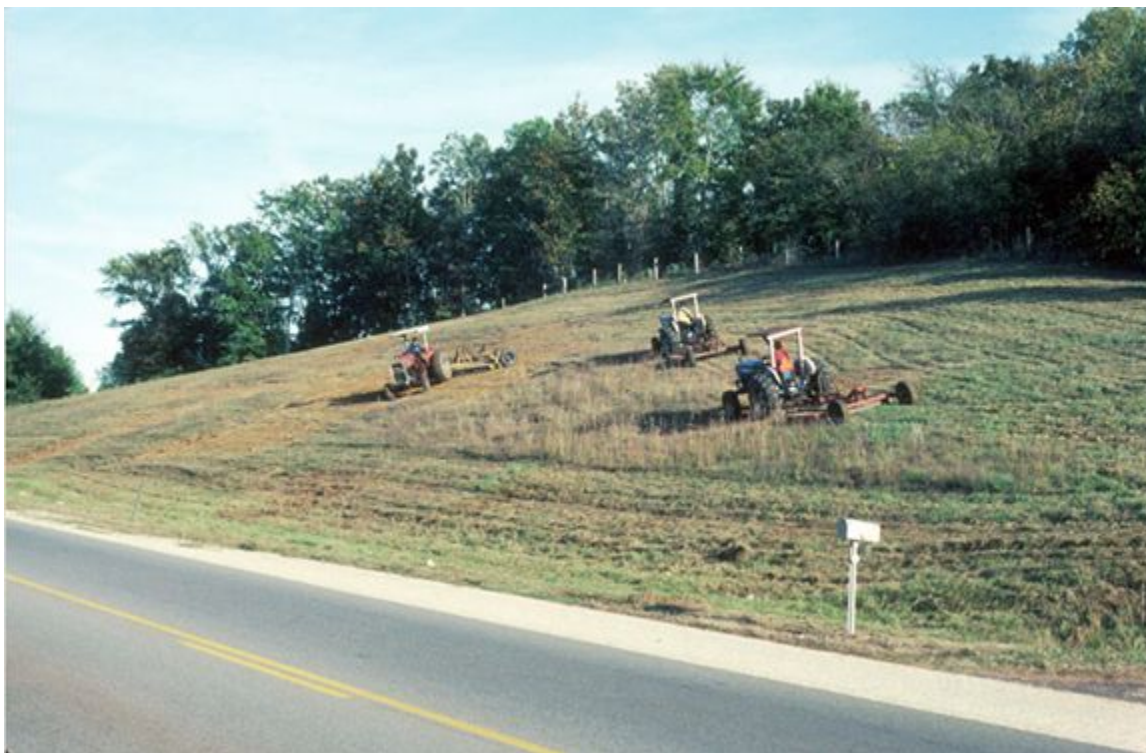
Figure 2-15. Mowing steep slope (rutting and slope failure).
