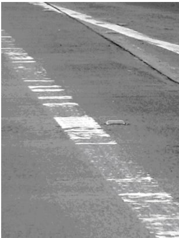
Figure 2-11. Major thermoplastic failure on concrete.
