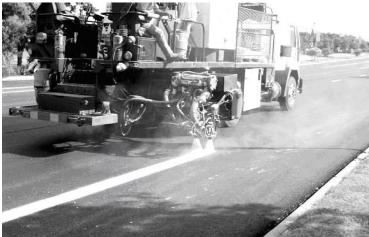
Figure 2-10. Typical sprayed thermoplastic operation.
