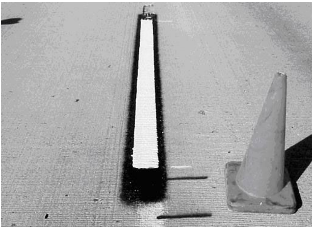
Figure 2-14. Typical bordered-contrast pavement marking for lane line.
