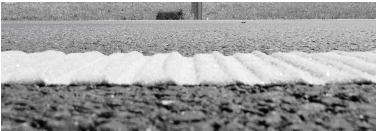
Figure 2-12. Typical inverted-profile thermoplastic marking (profile view).
